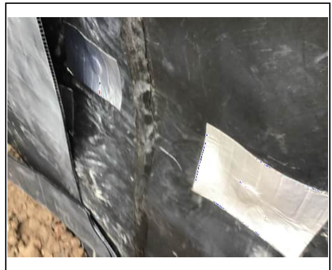
Pegs installed either side of
