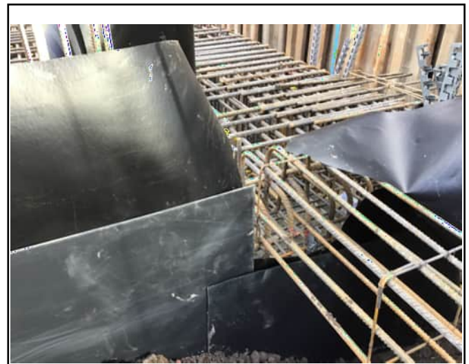
Membrane cut around ring beam
