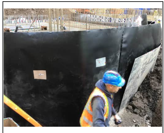
Pegs to bed in concrete sealed
