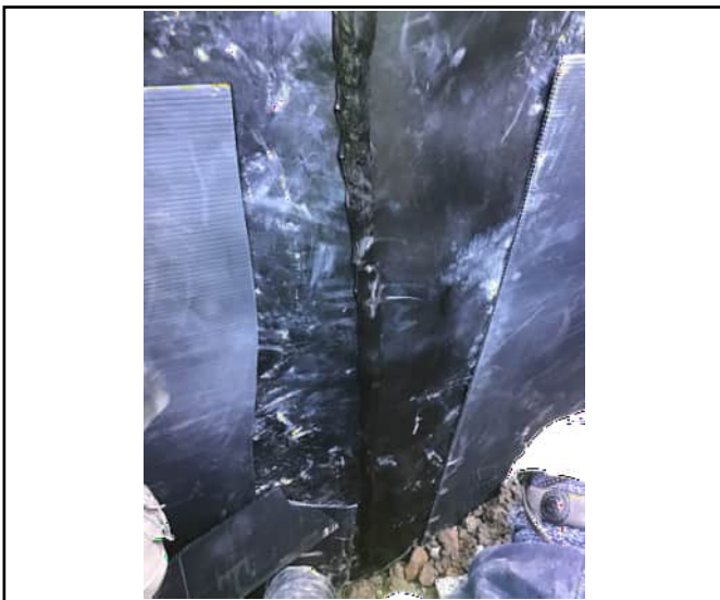
Extrusion weld on complete
