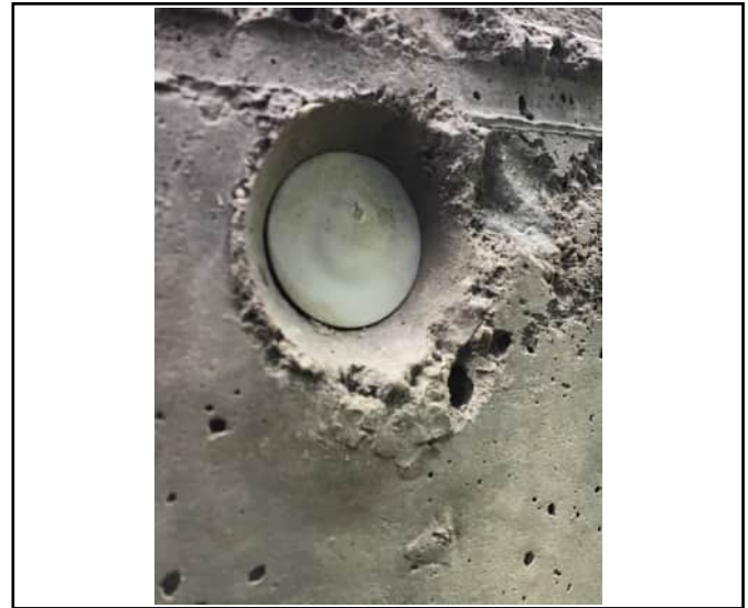
Dividag holes plugged with rubber
