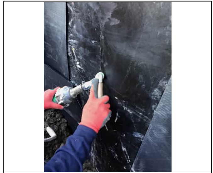
Hot weld in before extrusion
