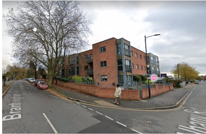
Figure 1 Street view of site
