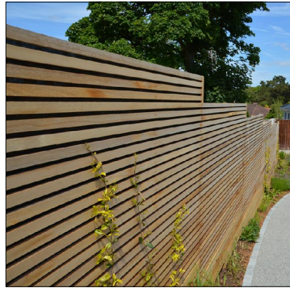
Timber Hit&Miss Fencing
