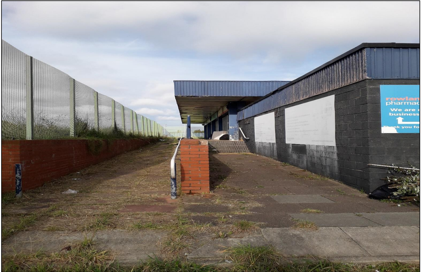
View along South West Facing side elevation of building.
