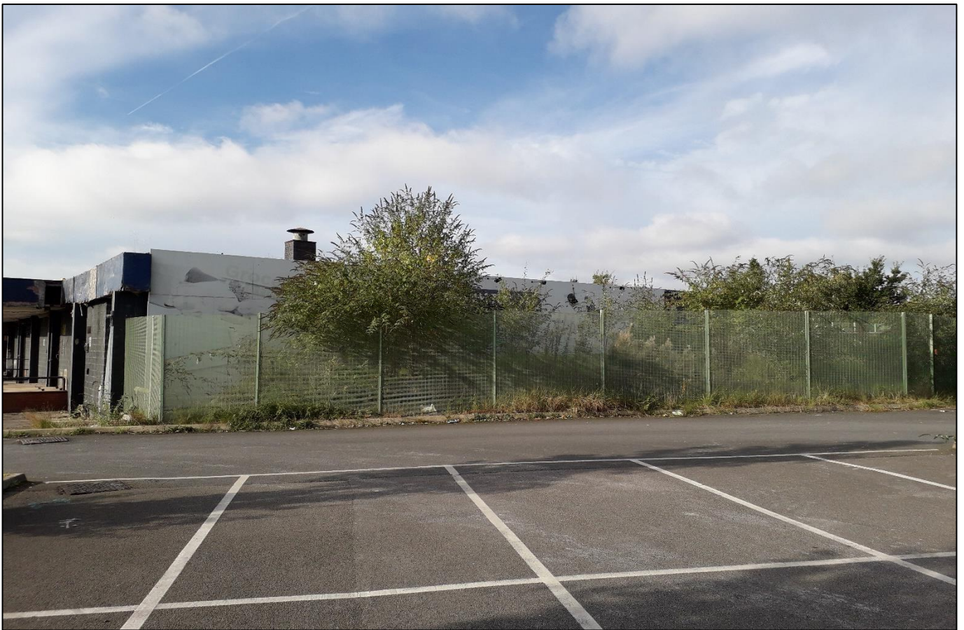
View along North East facing side elevation of building.
