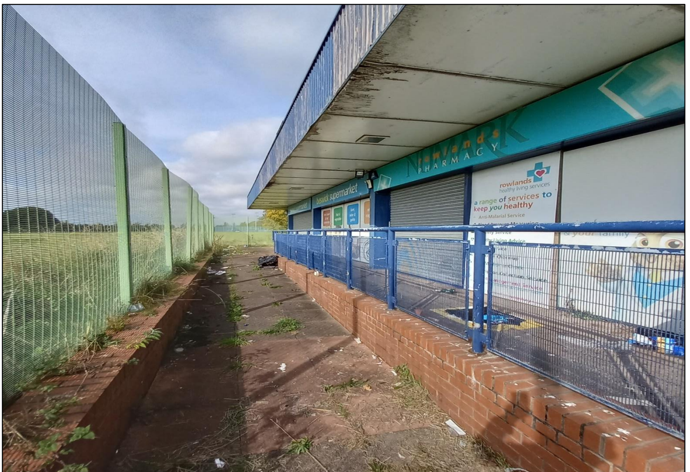
View along South West facing side elevation of building. Main entrances to the three shop units.
