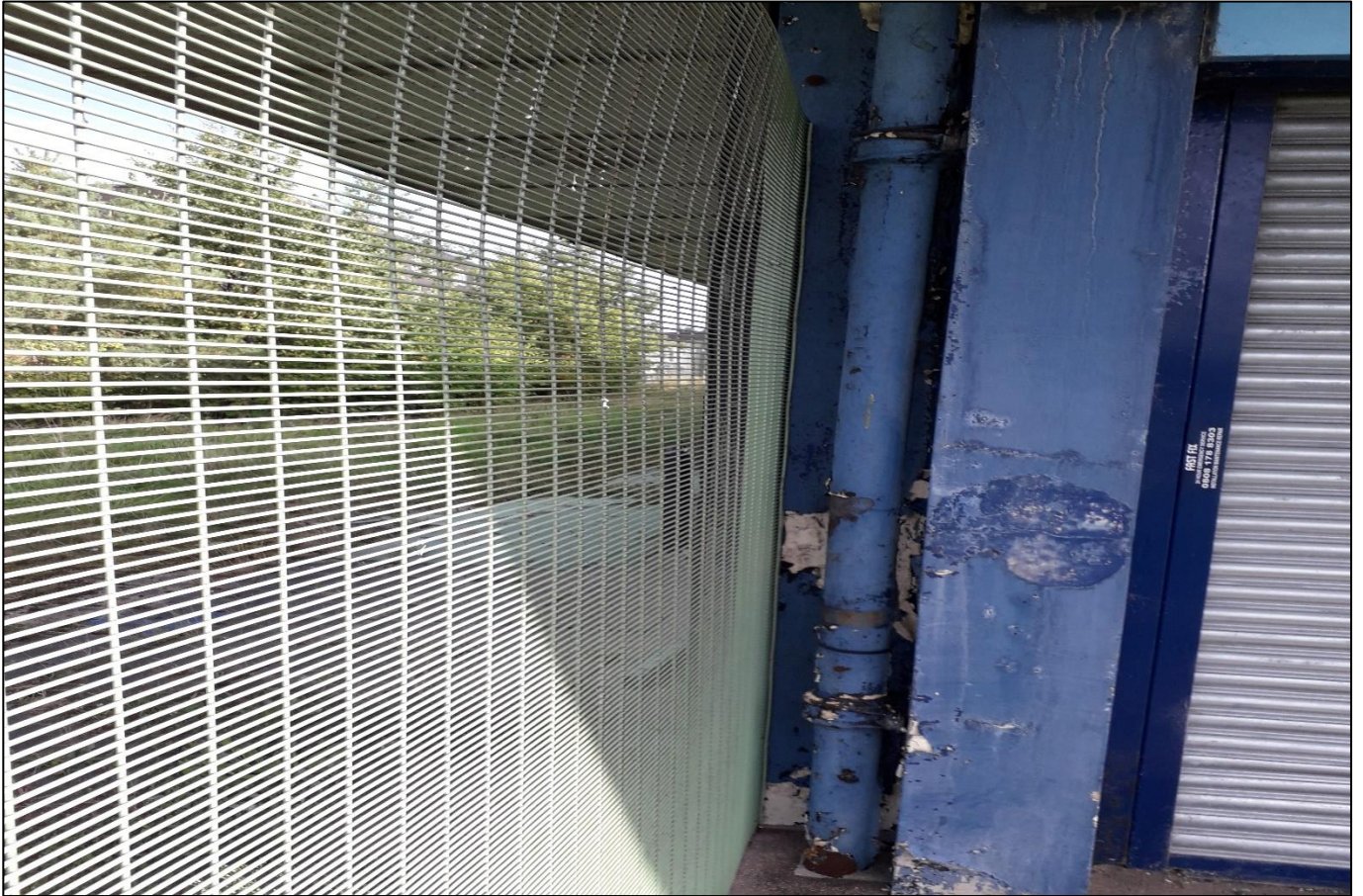
View at rear elevation of building – Existing fencing stops at the corner of the building.
