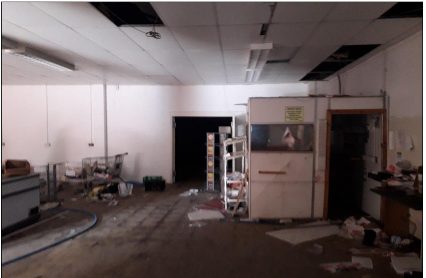
View within loading bay area to Unit 18.
