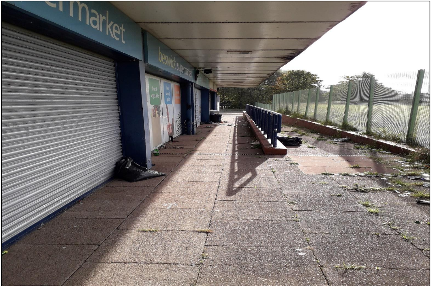
View along side elevation of building. Main entrances to the three shop units.
