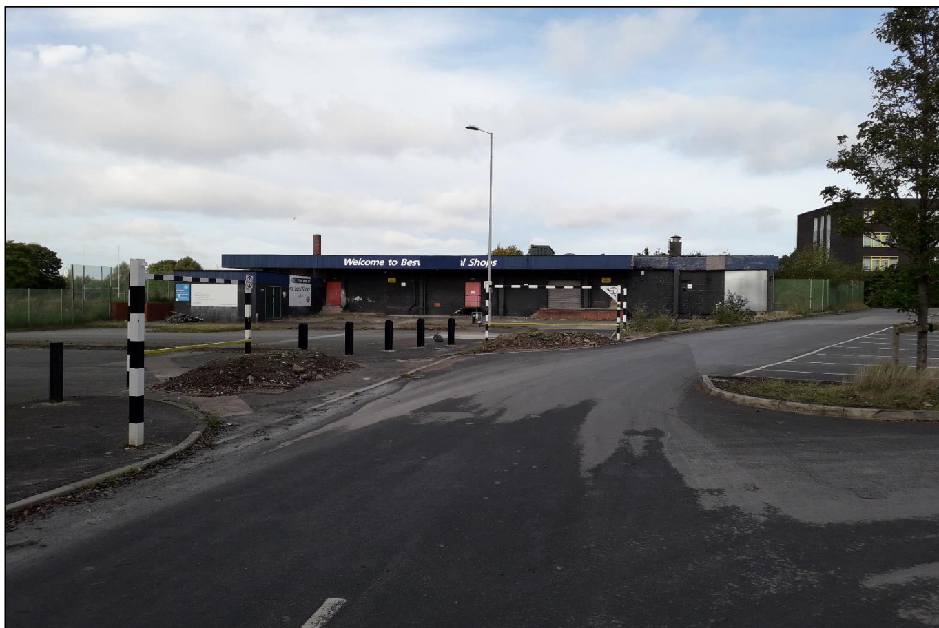
View of Beswick Shops to be demolished.
