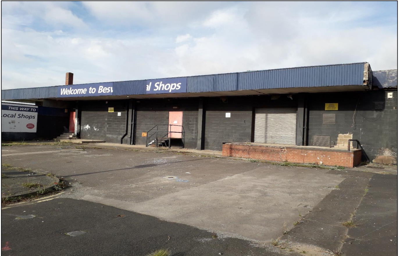
View of South East facing loading bay elevation.
