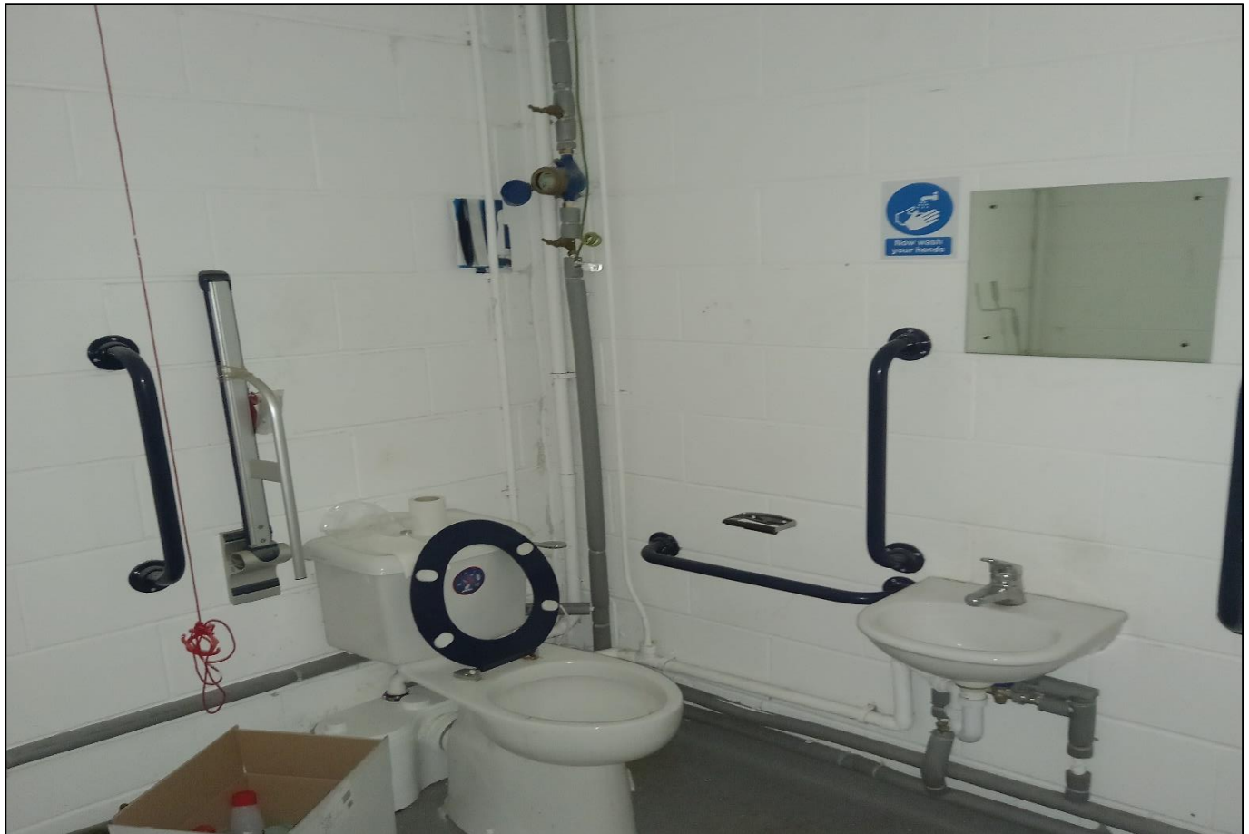
View of Rowlands Pharmacy Unit 11 – Accessible W.C.
