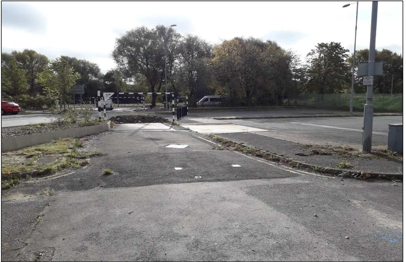
View of access road in front of the Beswick Shops (looking South East back towards Kylemore Way).
