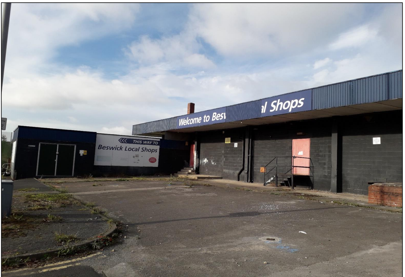
View of South East Facing Elevation.
