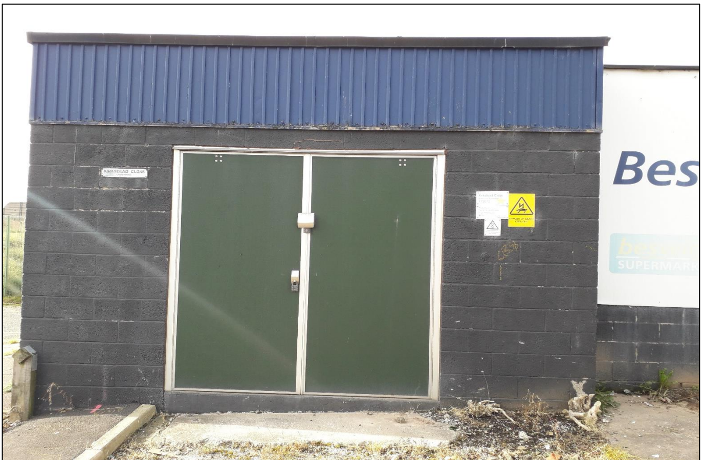
View of Kirkstead Close Electrical Substation – To remain in place, walls abutting it to be demolished.
