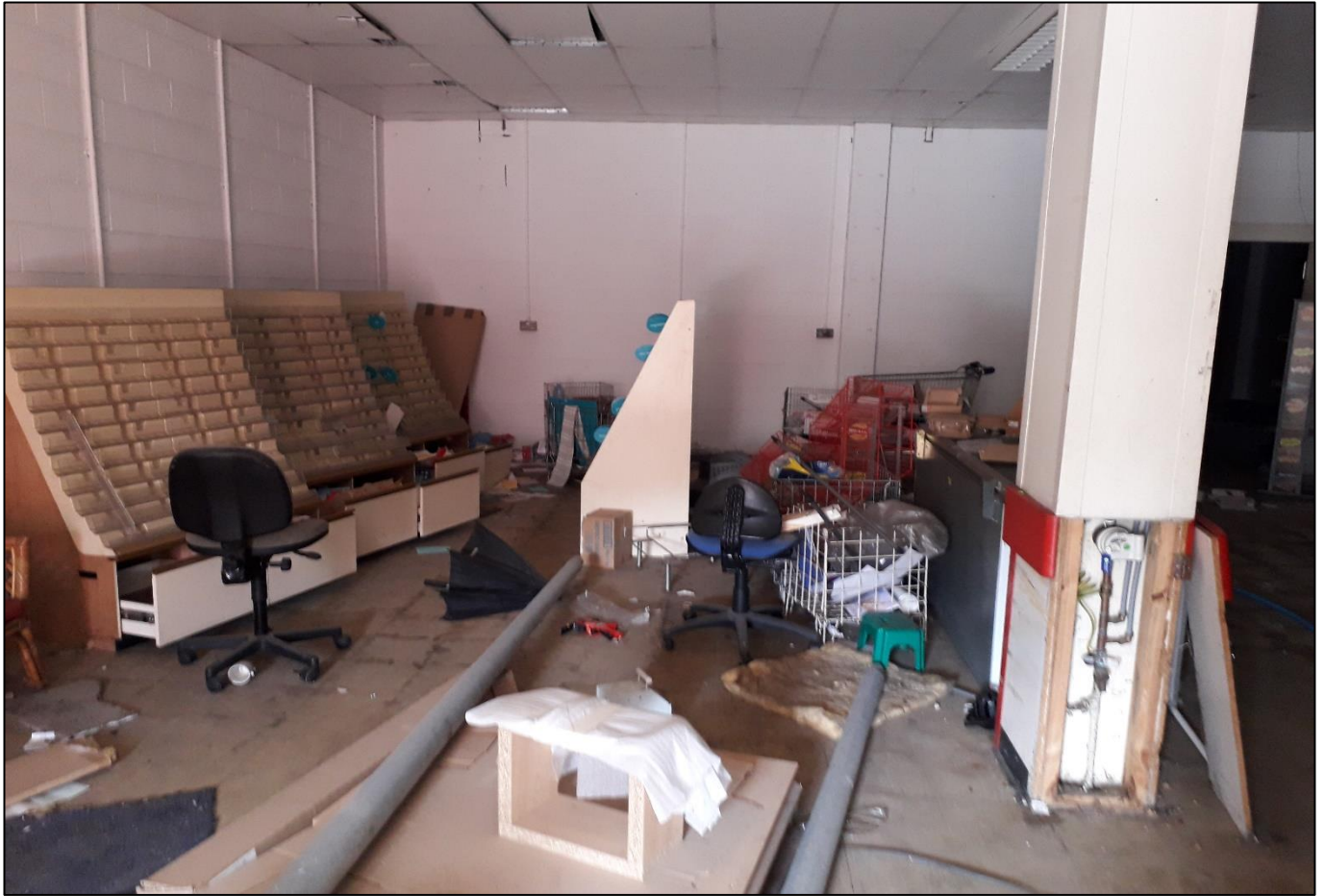
View within loading bay area to Unit 18
