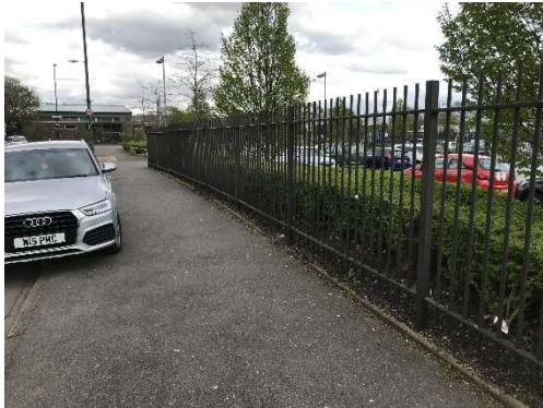
Existing fence to Albert Street
