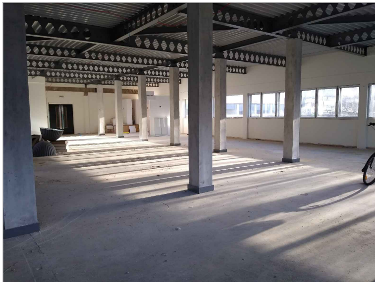
Existing 3rd Floor Ceilings
