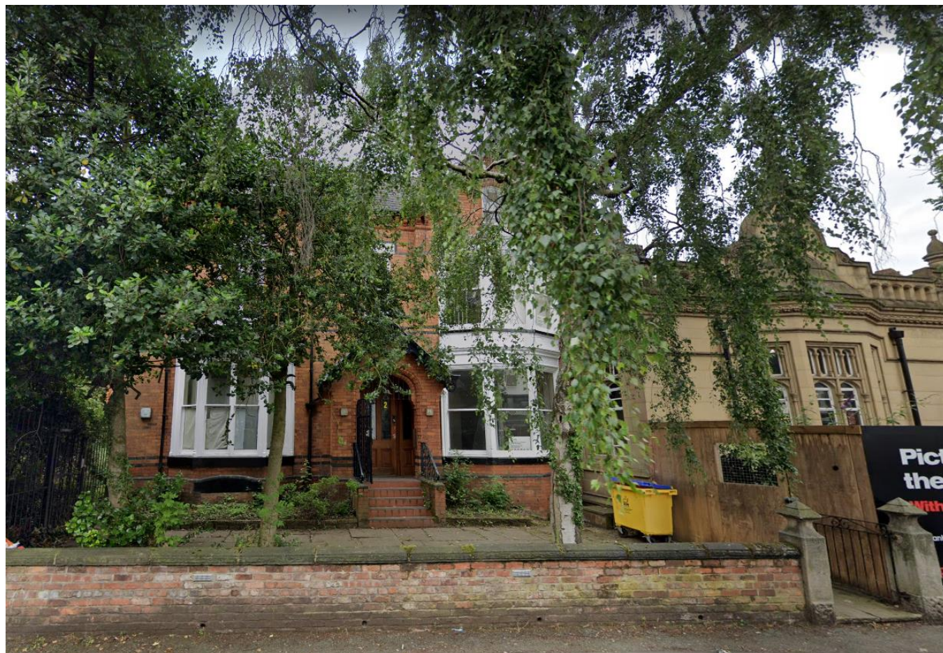
Front of the application property prior to works commencing on the adjacent land
