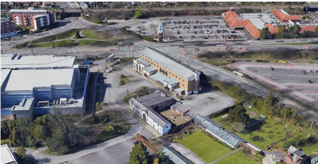
The Stable block is not completely subsumed by surrounding developments from the early years of the 21 st century
