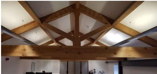
Replacement roof trusses from 2002 repairs/conversion.
