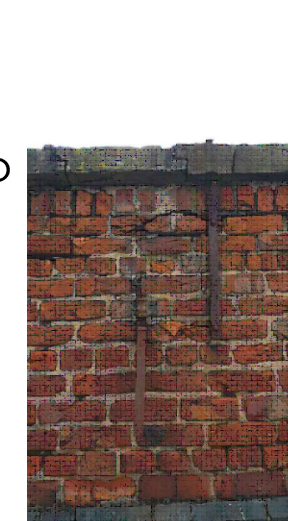
4 Steel dowel through coping stone, record photo
