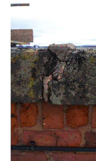
2 Coping stone mortar joint, record photo
