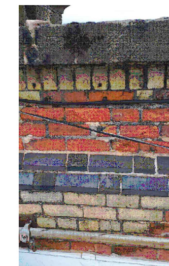
1 General view of front parapet, record photo
