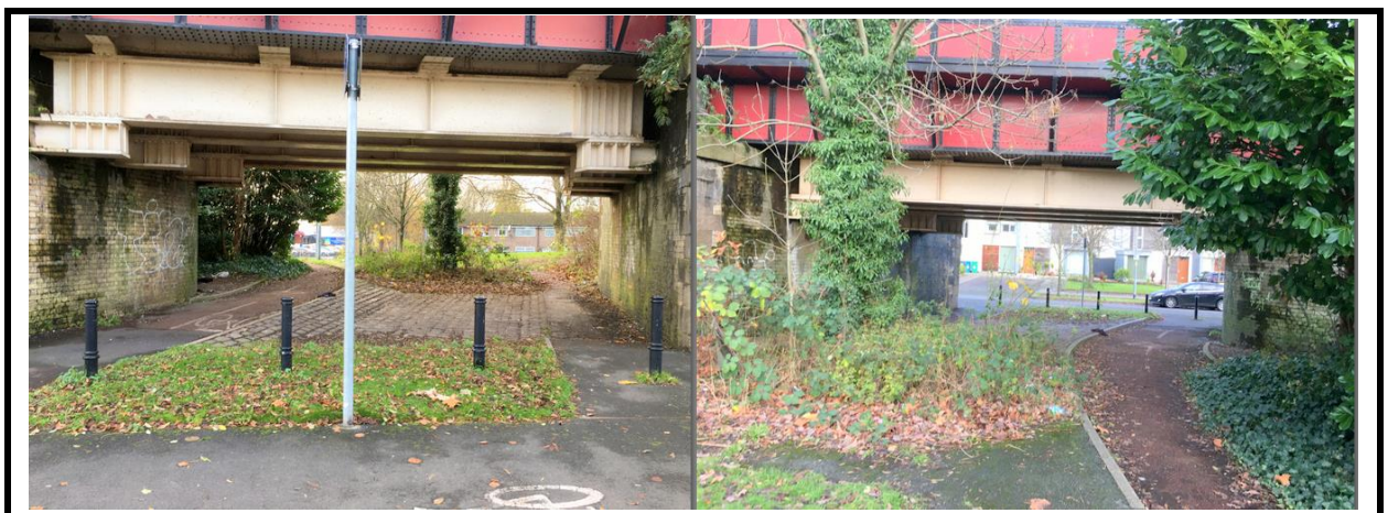
View west and east under viaduct route
