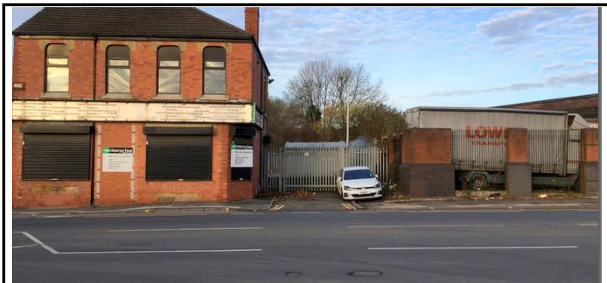
Site access from Ashton Old Road
