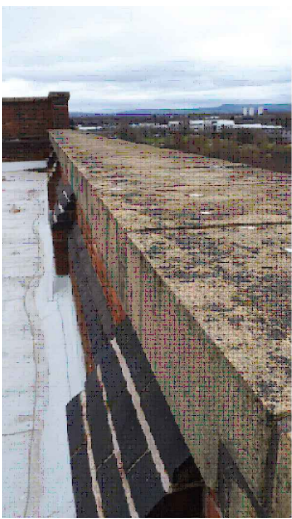
11 Modern concrete copings to rear elevation, record photo
