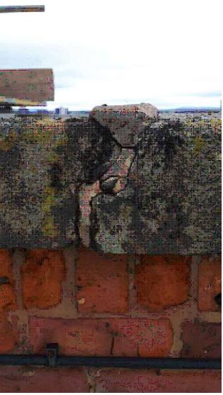
2 Coping stone mortar joint, record photo
