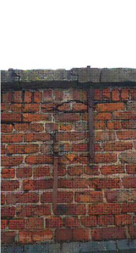
4 Steel dowel through coping stone, record photo
