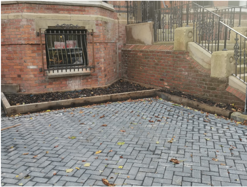
Raised planters using treated timber planters.
