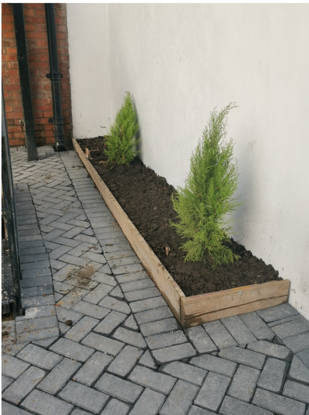
Rear: Raised planter using treated timber sleepers. Hard Landscaping.
