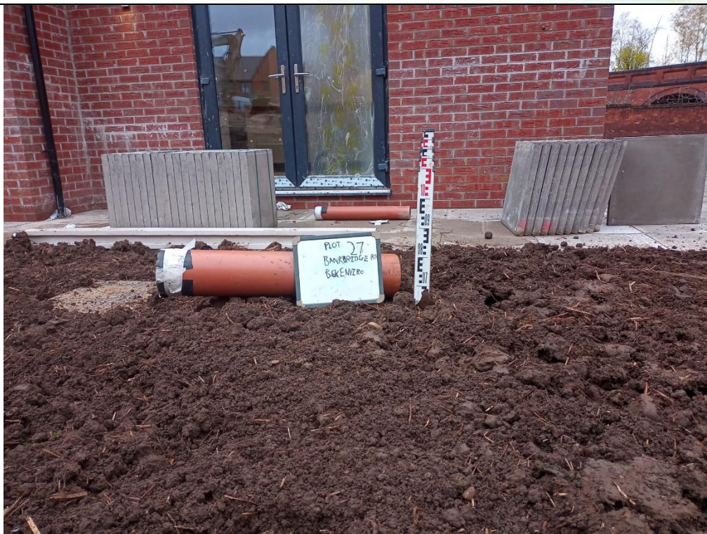
Photograph 2: Validation of Garden Capping Thickness
