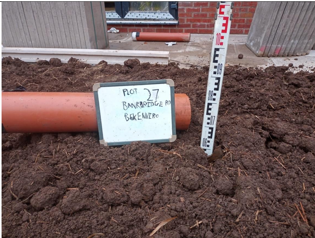
Photograph 1: Validation of Garden Capping Thickness
