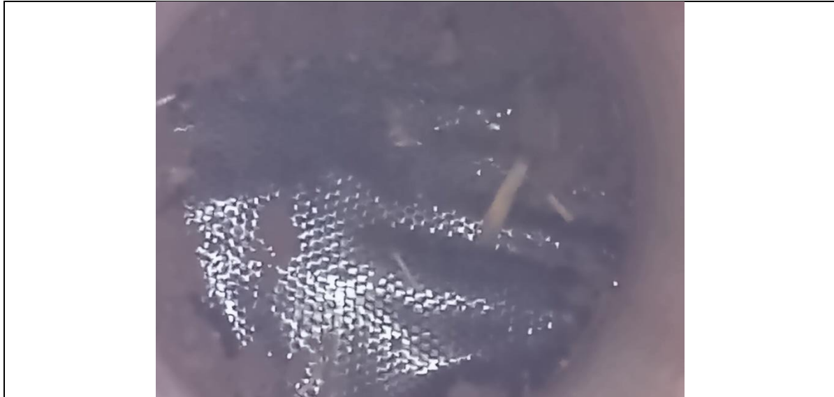
Photograph 3: Validation of Geotextile Membrane
