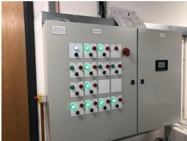
Figure 7.2: Typical Mechanical Services Control Panel
