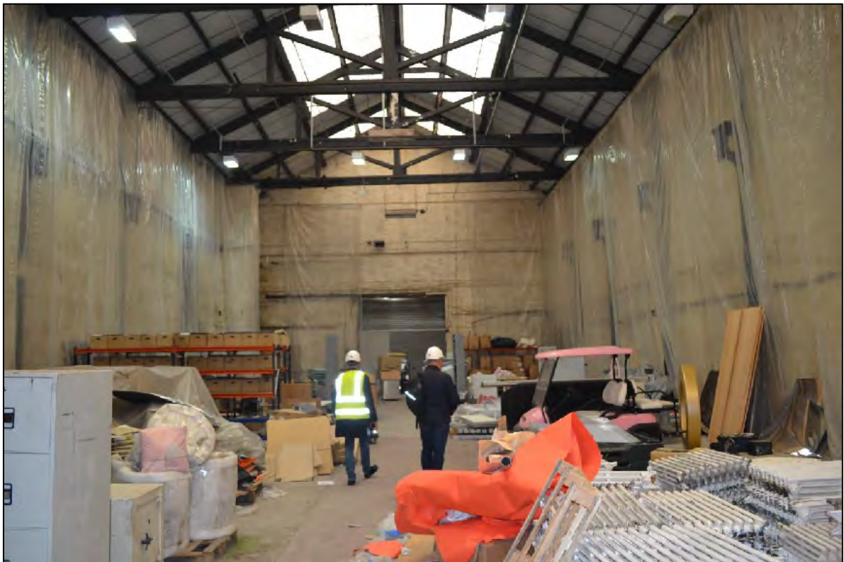
Photograph 72: General view south-east within C2
