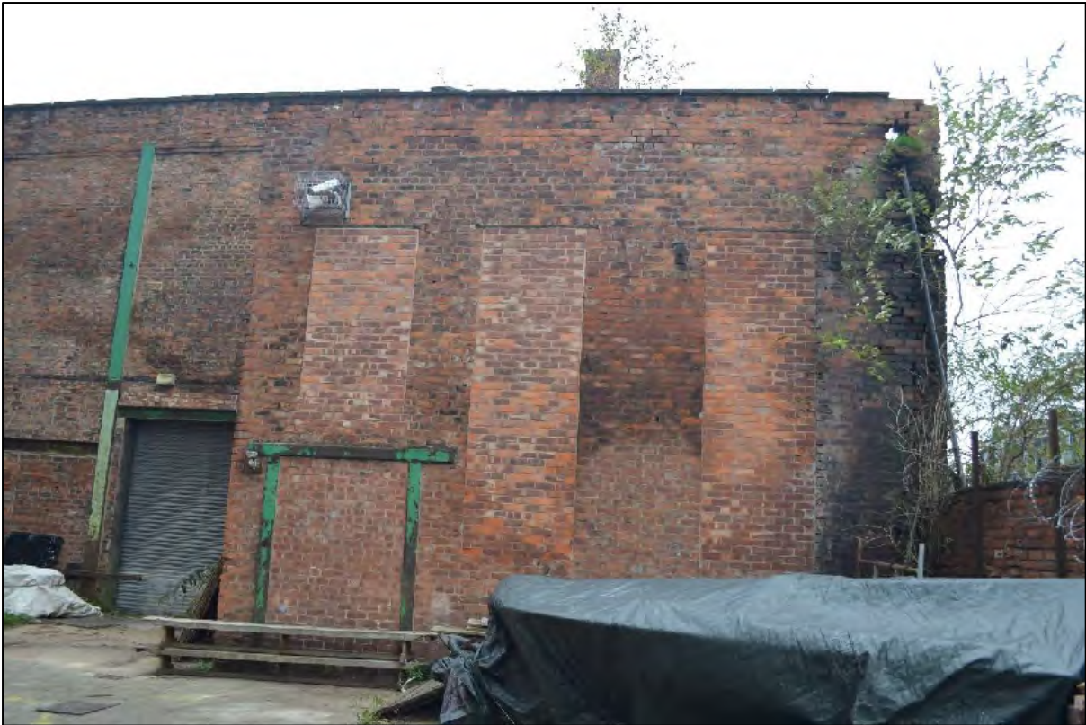
Photograph 27: View west of the north-eastern elevation of Structure C5
