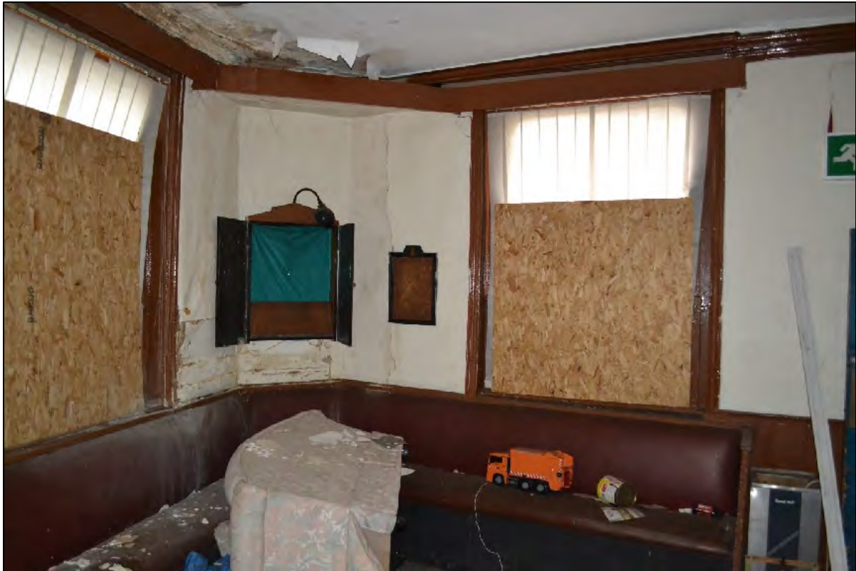
Photograph 119: View south of former corner entrance to Public House
