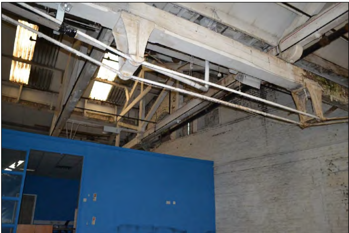
Photograph 64: General view of ceiling of Structure B from first floor
