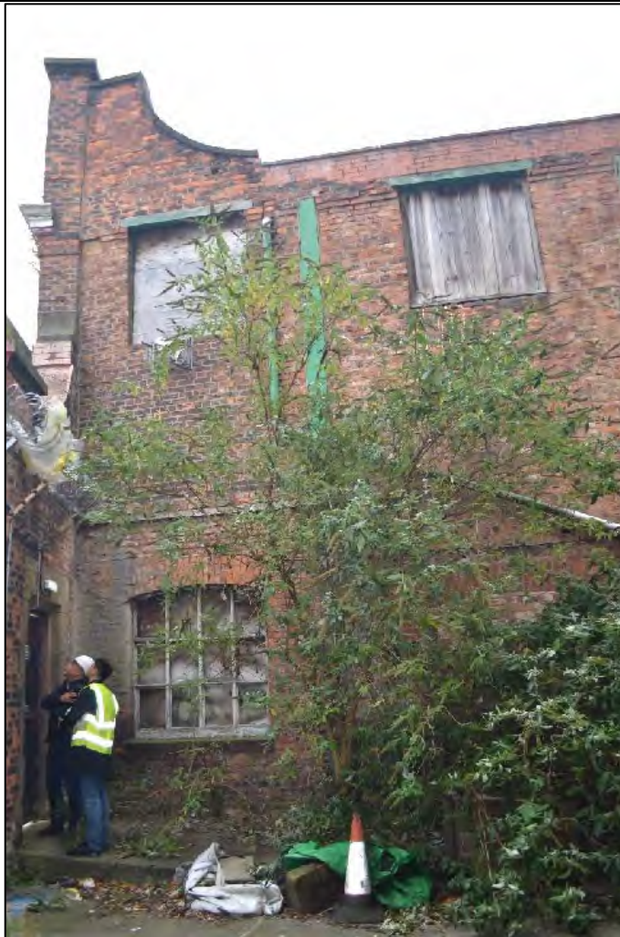
Photograph 21: View west of the north-eastern elevation, Structure C1
