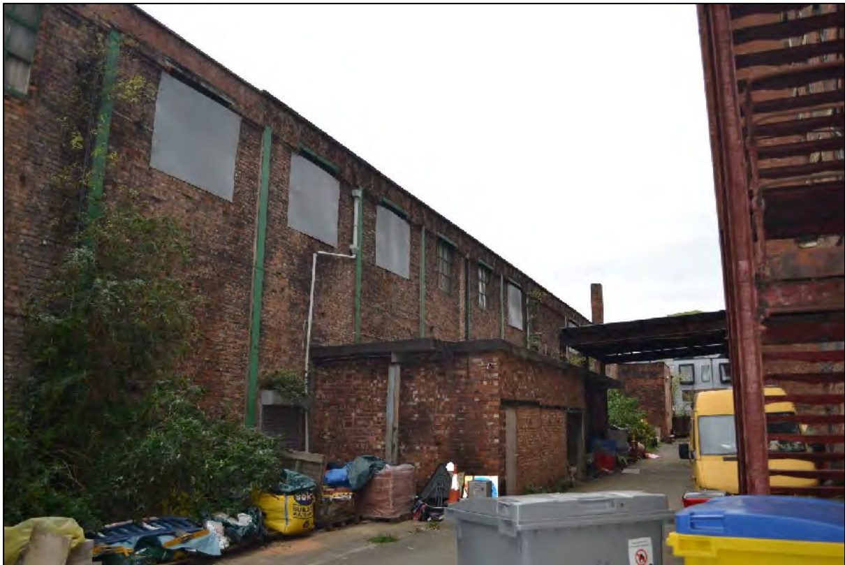
Photograph 19: View north of the north-eastern elevation of the site, the exterior of Structures C2 and C4
