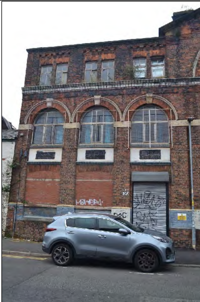
Photograph 13: View north-west of the Pollard St exterior of Structure A
