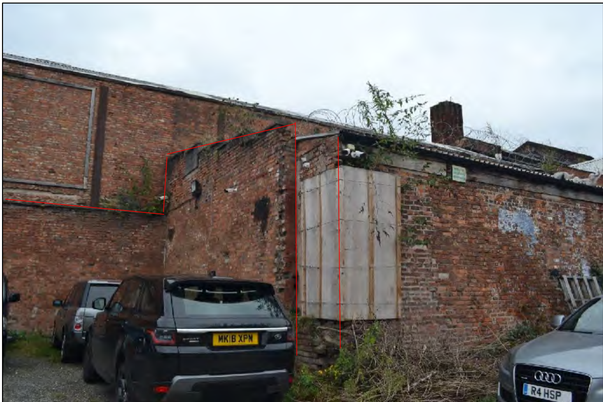
Photograph 36: View east of the corner of Structure E, showing evidence of since demolished buildings (red lines)
