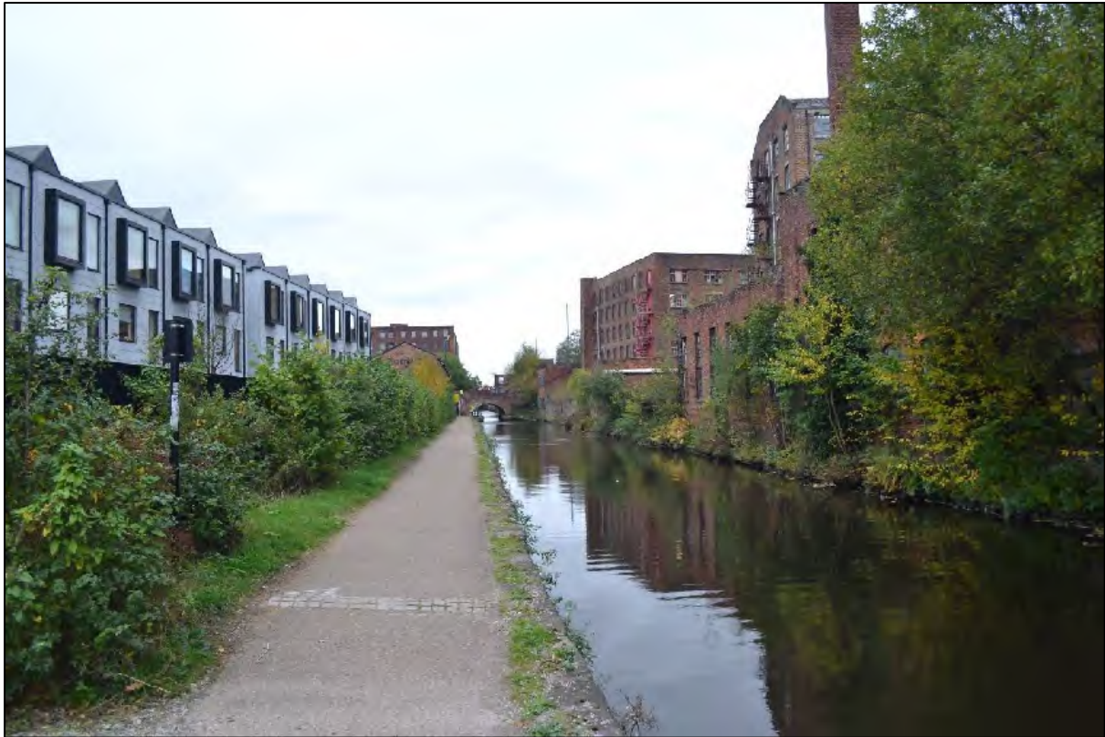
Photograph 143: View north-east along the Ashton Canal from Bridge Number 4 to Bridge Number 5
