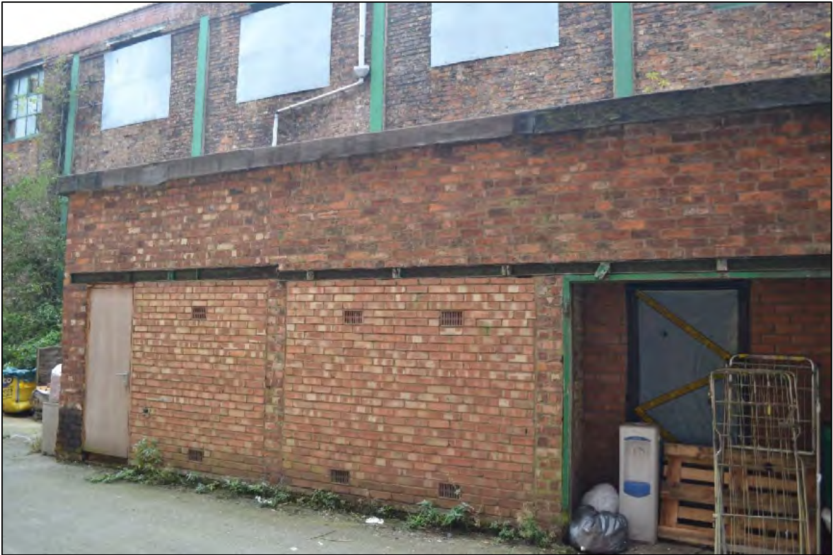
Photograph 79: View south of the north-eastern elevation of C4
