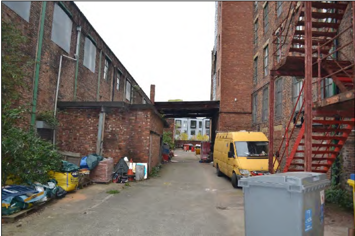
Photograph 5: View north-west within the courtyard separating the PDA from the adjacent Hope Mill
