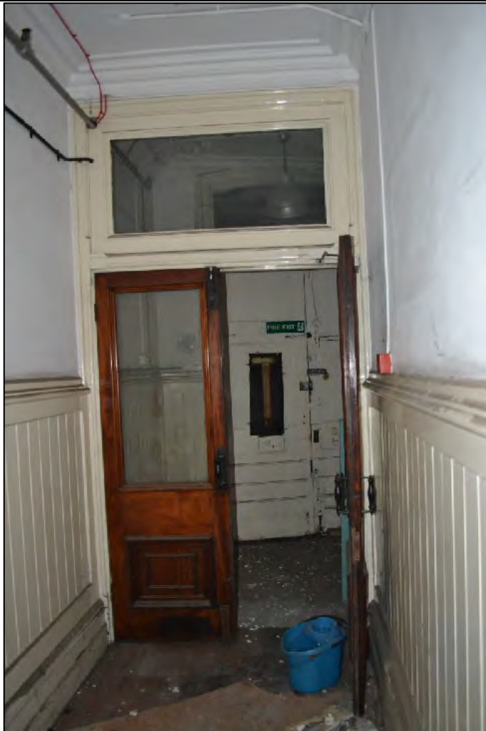
Photograph 43: View south-east of the wooden doors between the Pollard Street entrance and main hall
