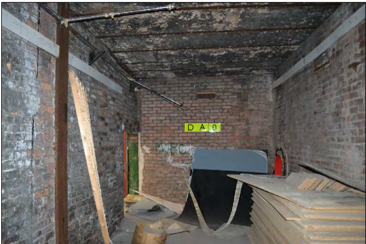
Photograph 84: View south-east across the northernmost room of C4
