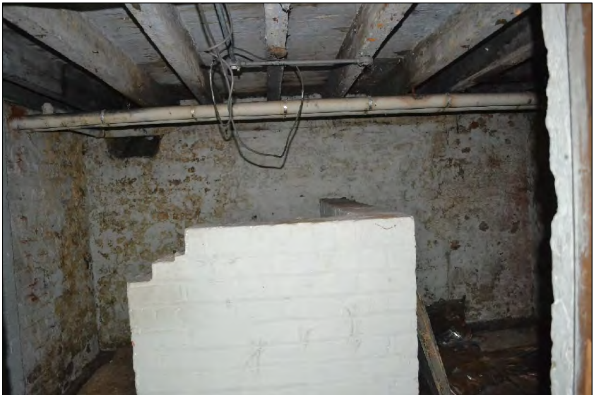
Photograph 128: View south-west of former storage room within cellar
