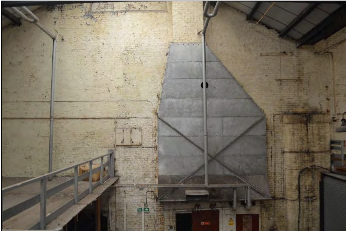
Photograph 99: View of the metal extractor hood for D3 on the wall of D2
