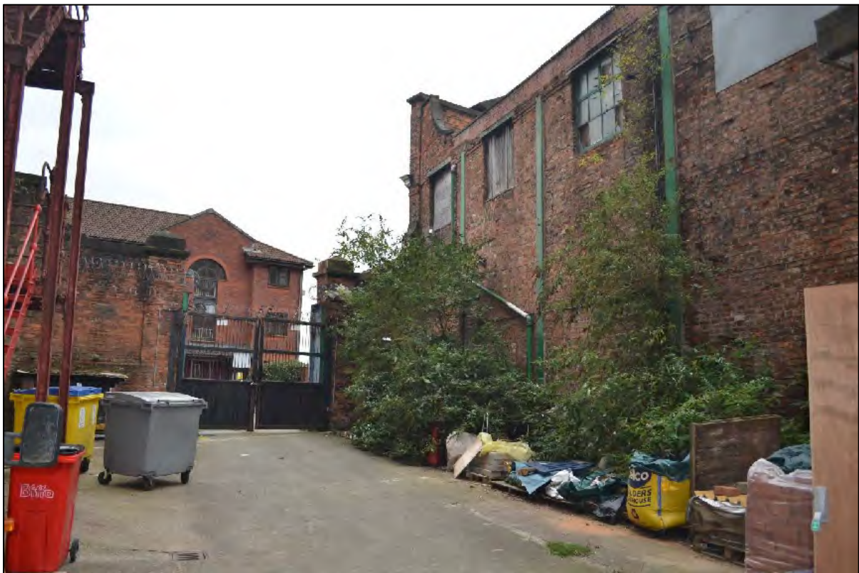
Photograph 20: View south of the north-eastern elevation of the site, the exterior of Structure C
