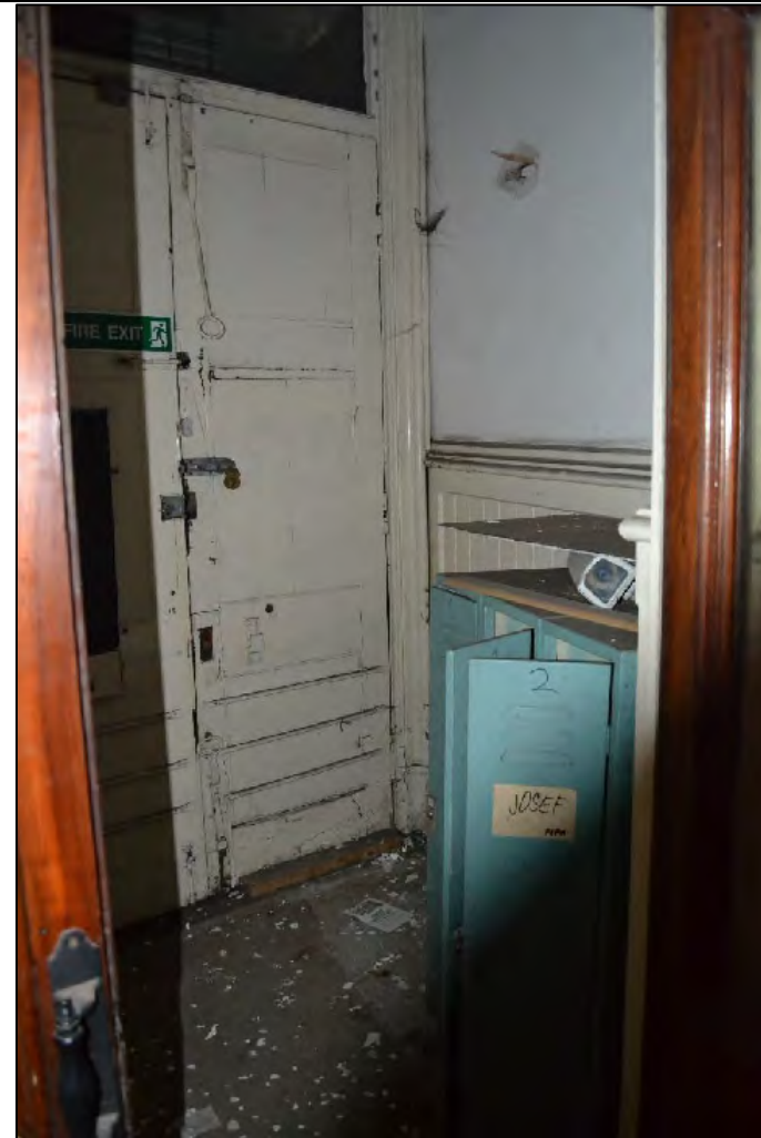
Photograph 42: View south of the wider entryway to Structure A from Pollard Street
