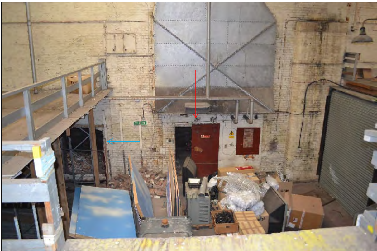
Photograph 98: View north-west of the entrance to D3 (red arrow) and blocked entrance to D4 (blue arrow)
