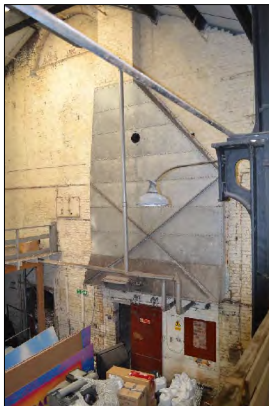
Photograph 94: View of north-western wall of D2 from the first floor of C3
