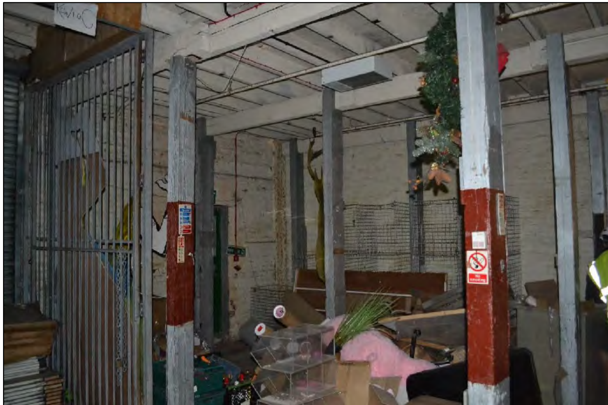
Photograph 74: View east of ground floor within C3. Note the pillars supporting the timber first floor
