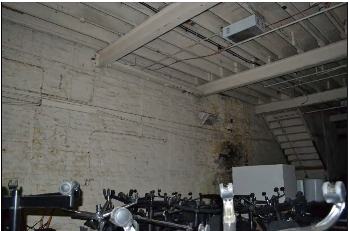
Photograph 60: General view north-east of ground floor of Structure B. Note staircase in background leading to first floor
