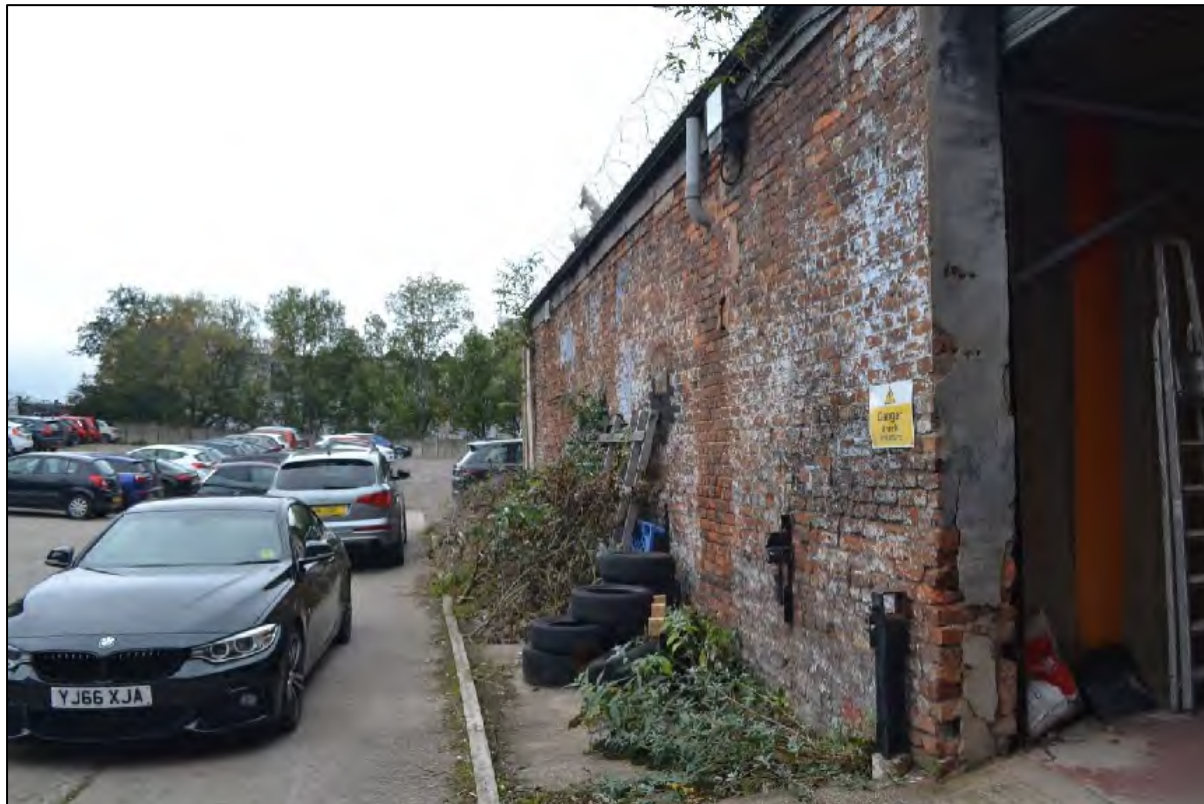
Photograph 34: View north along the north-western elevation of Structures E1 and E2
