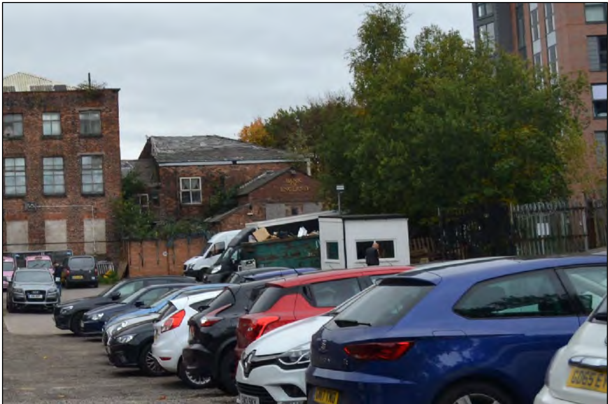
Photograph 113: General view south of the north-western, first floor elevation of the former Public House
