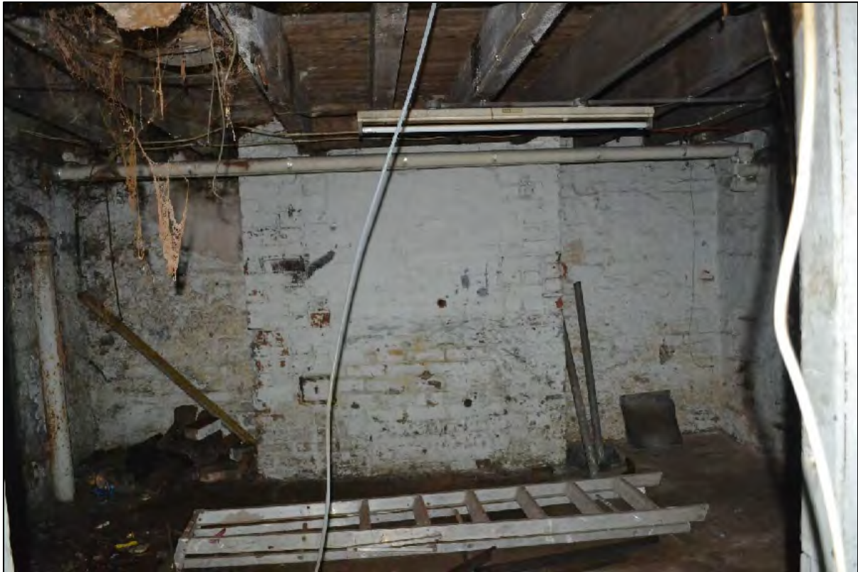
Photograph 129: View north-east of former storage room within cellar
