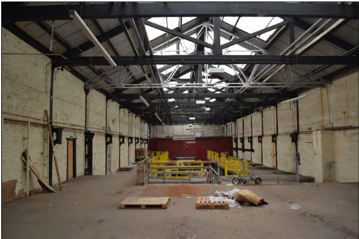
Photograph 96: General view south-east across the first floor mezzanine within D2
