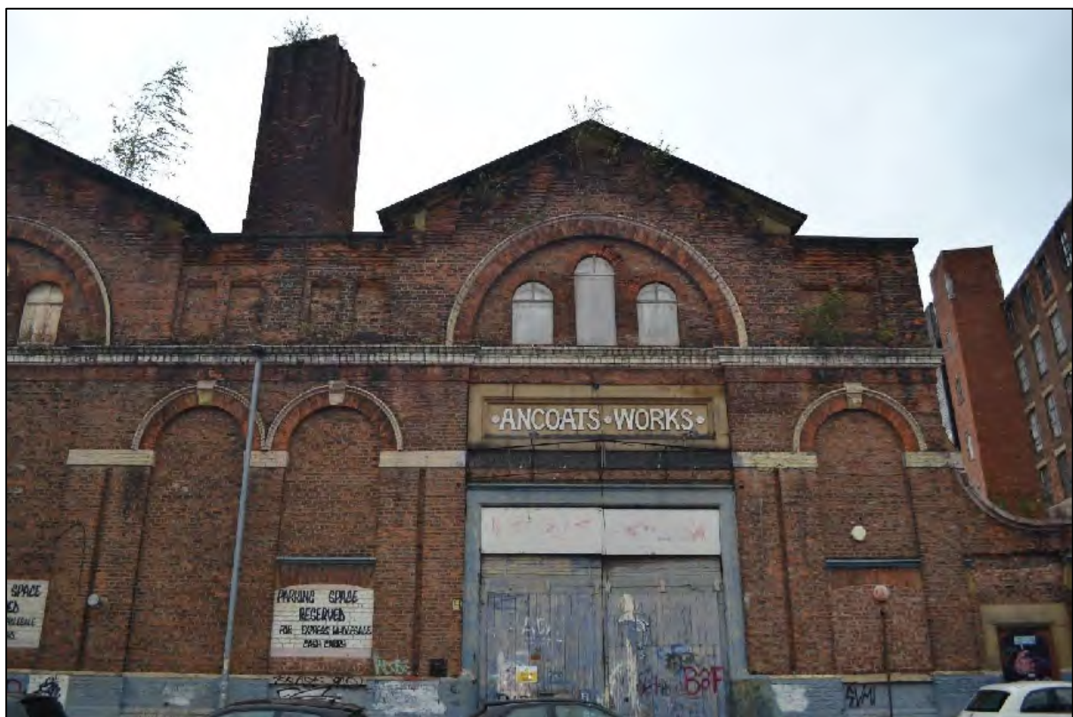
Photograph 16: View north-east of the Pollard St exterior of Structure C
