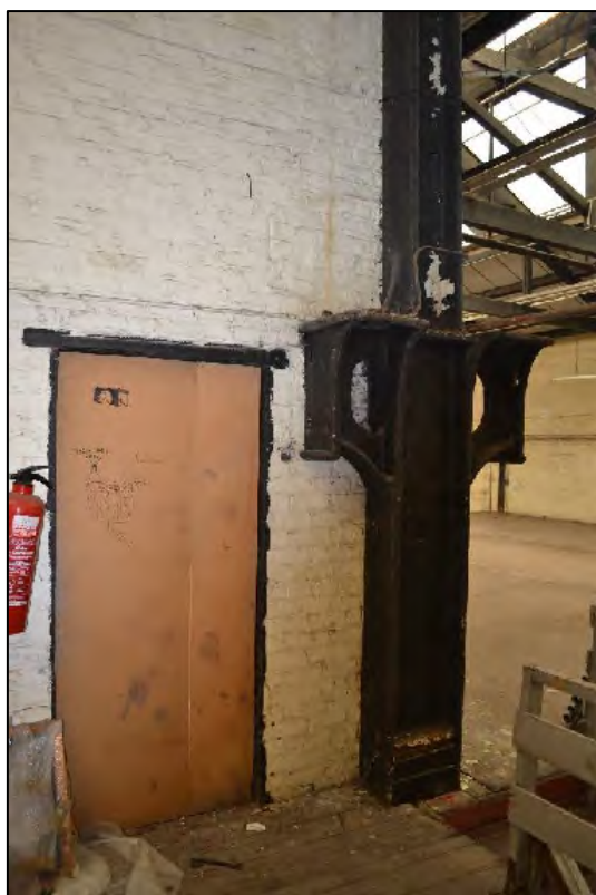
Photograph 77: Detailed view of the former first floor doorway connecting C3 and C2
