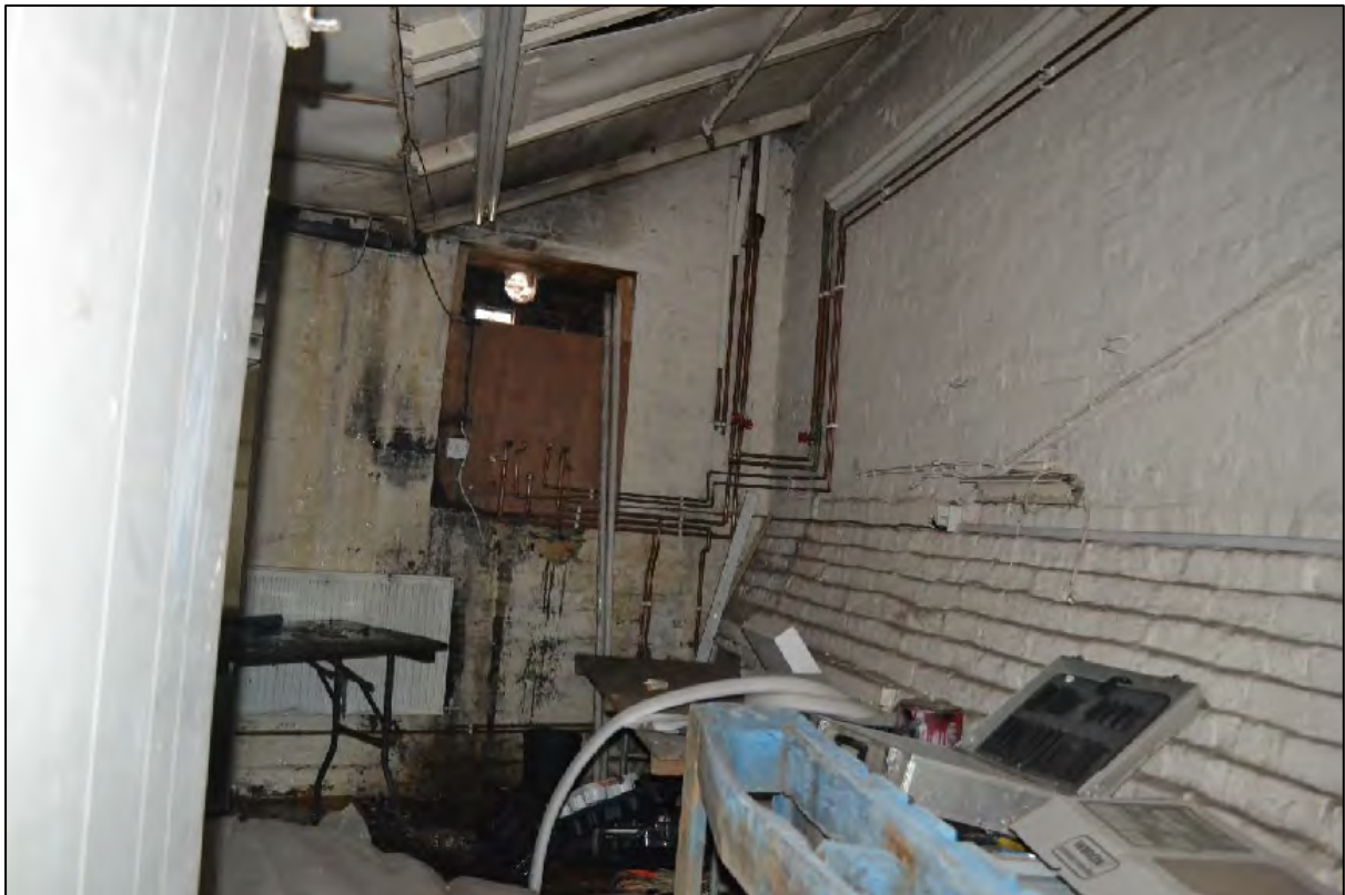
Photograph 61: View south within plant room within Structure B ground floor
