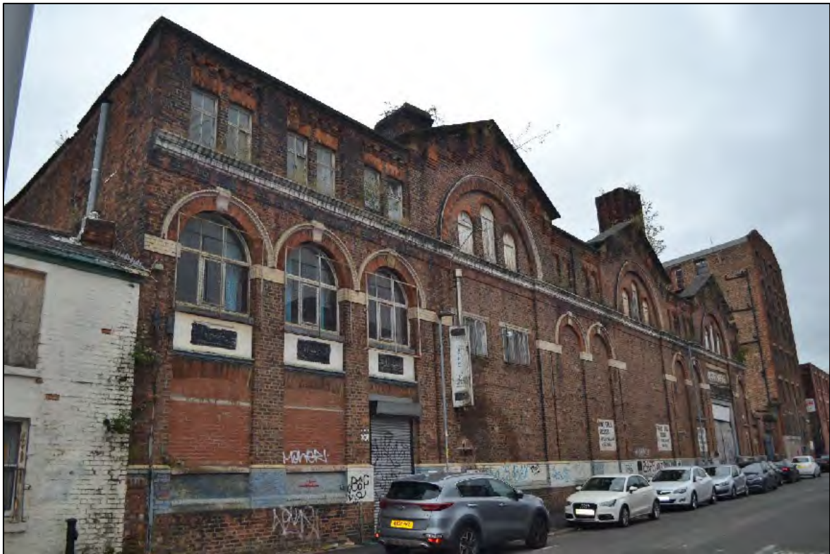
Photograph 12: View north of the entire Pollard Street façade
