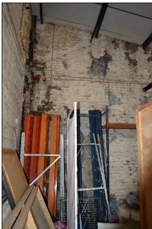
Photograph 105: View of the south-eastern wall within E1.
