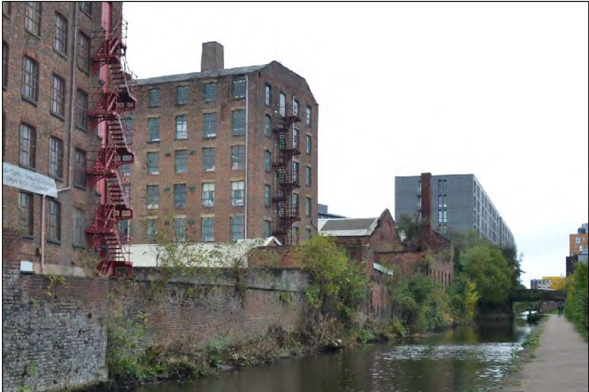
Photograph 137: View south-west from the Ashton Canal towpath of the north-eastern and north-western elevations of Hope Mill between Spectator Mill and the Ancoats Works
