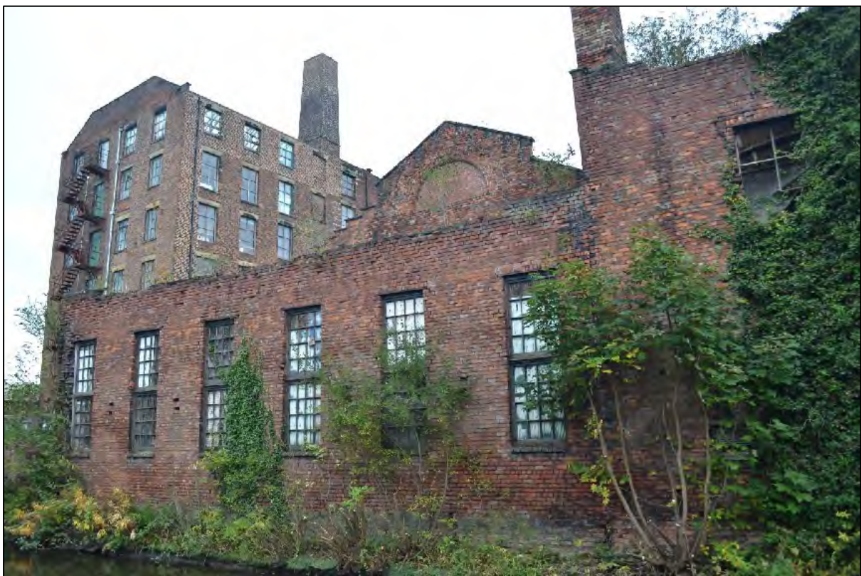
Photograph 136: View east from the Ashton Canal towpath of the north-western and south-western elevations of Hope Mill with Ancoats Works in the foreground
