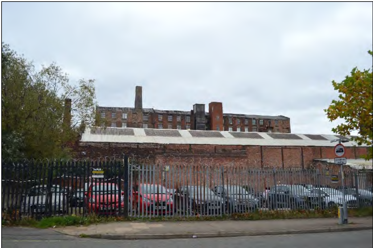
Photograph 135: View north-east from Carruthers Street of the upper floors of Hope Mill above the Ancoats Works roofline
