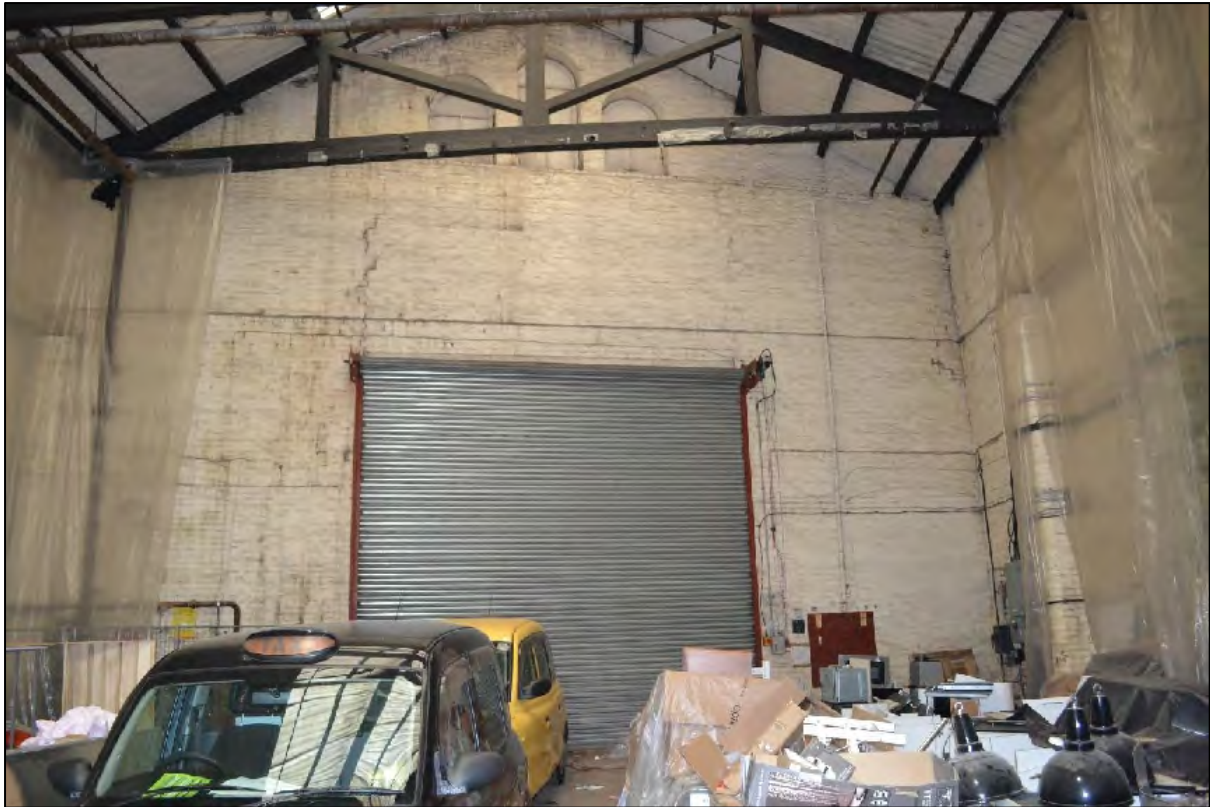
Photograph 65: View south-east of rolling shutter access to Pollard Street, from within C1
