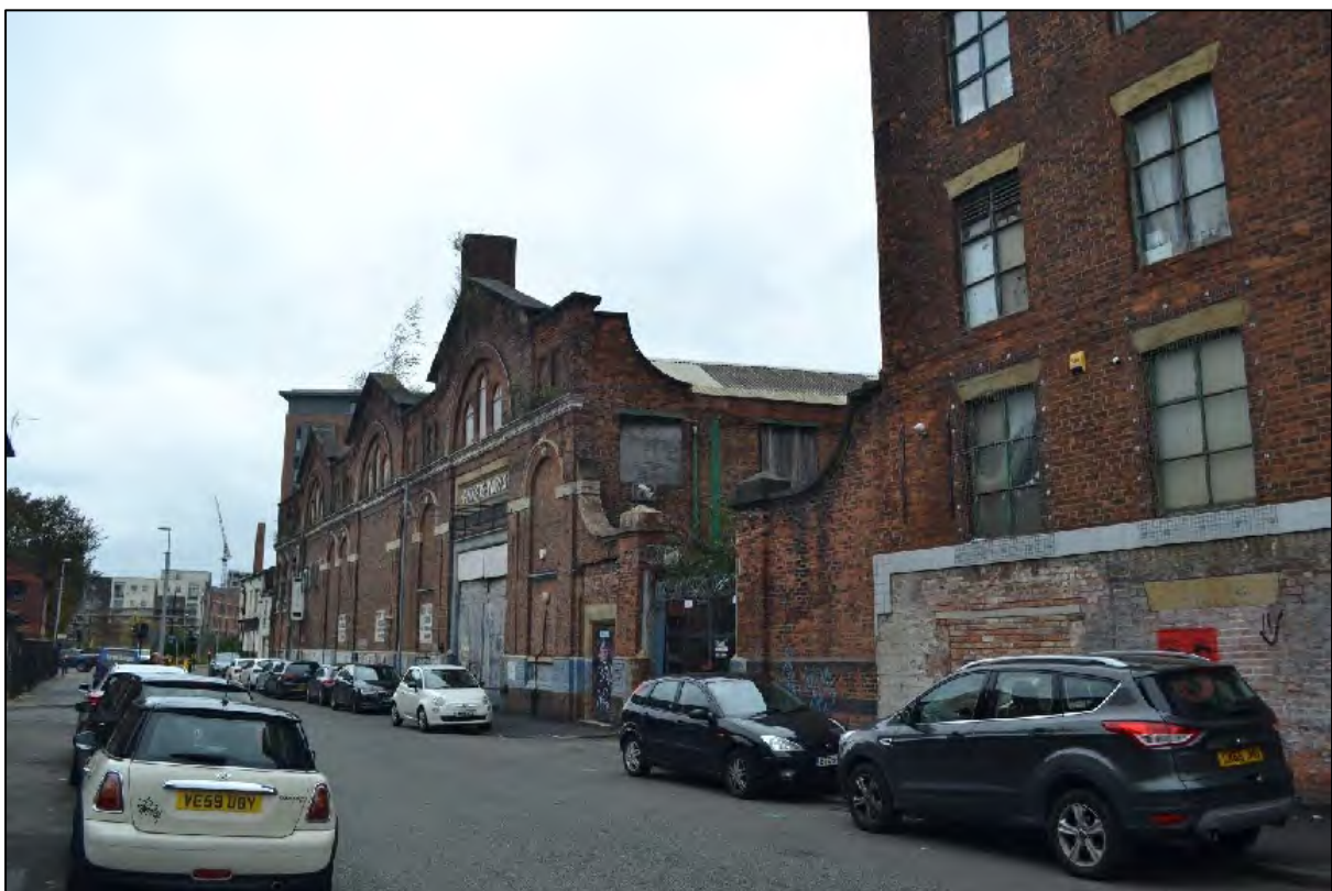
Photograph 18: View west along Pollard Street of the Ancoats Works façade
