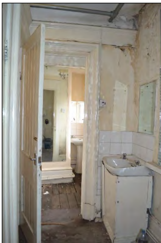
Photograph 57: General view west of second floor toilets, Structure A
