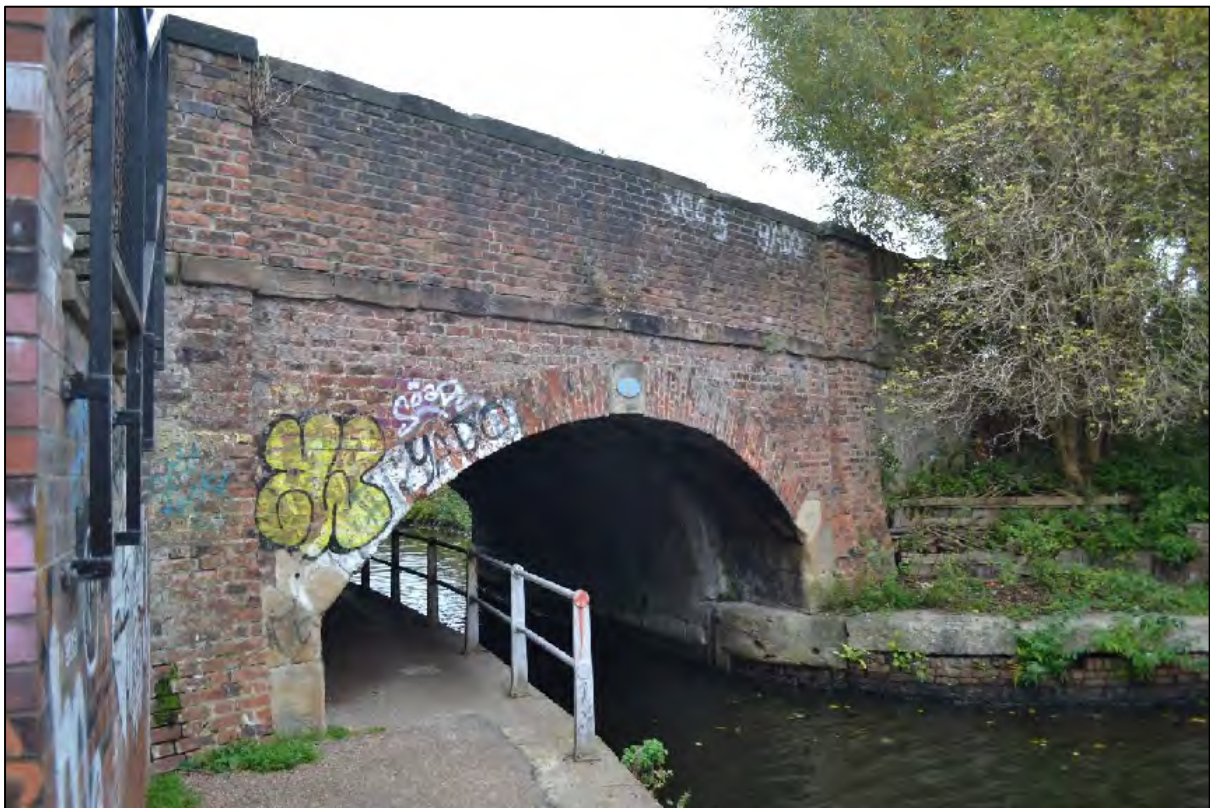
Photograph 144: View of the south-western façade of the Grade II listed Bridge Number 5
