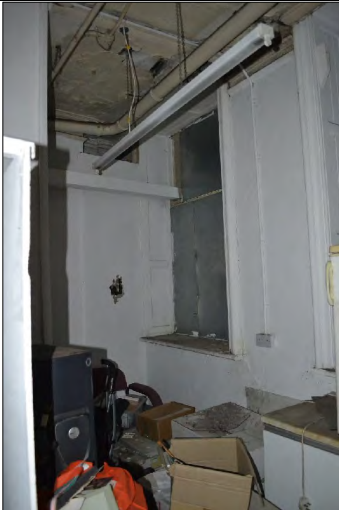
Photograph 51: View west of the former first floor kitchen space, Structure A
