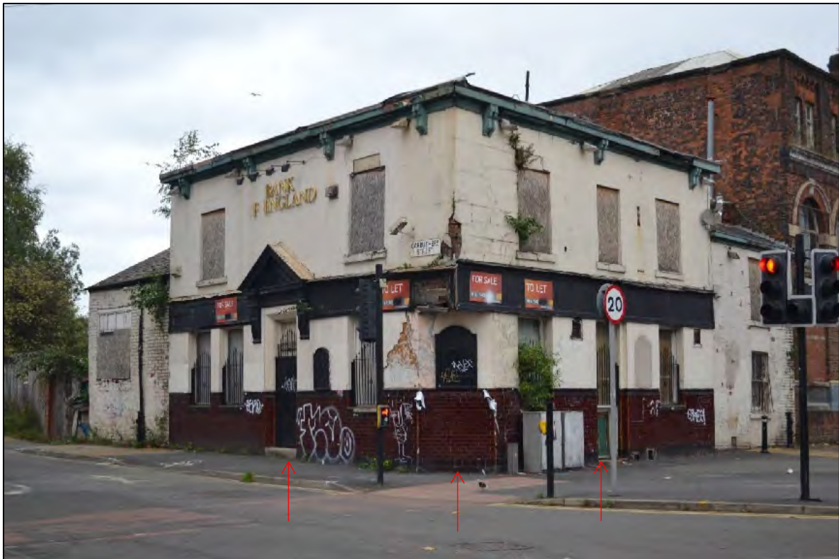
Photograph 107: View north of the Bank of England PH at the junction of Pollard Street and Caruthers Street. Note the three former entrances (red arrows)
