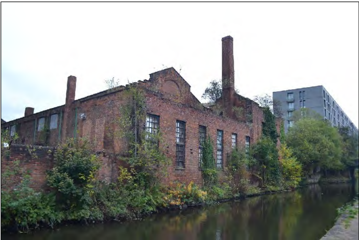
Photograph 28: View south-west of the north-western elevation, Structures C5, D3 and D4
