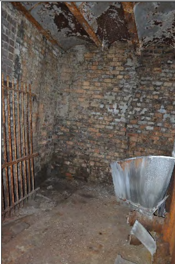
Photograph 101: General view of the northern corner of D3
