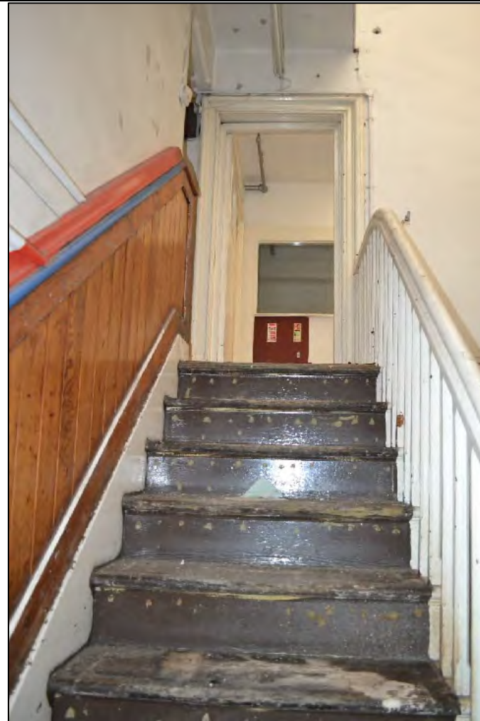
Photograph 54: View north-east along the staircase leading to the second floor, Structure A
