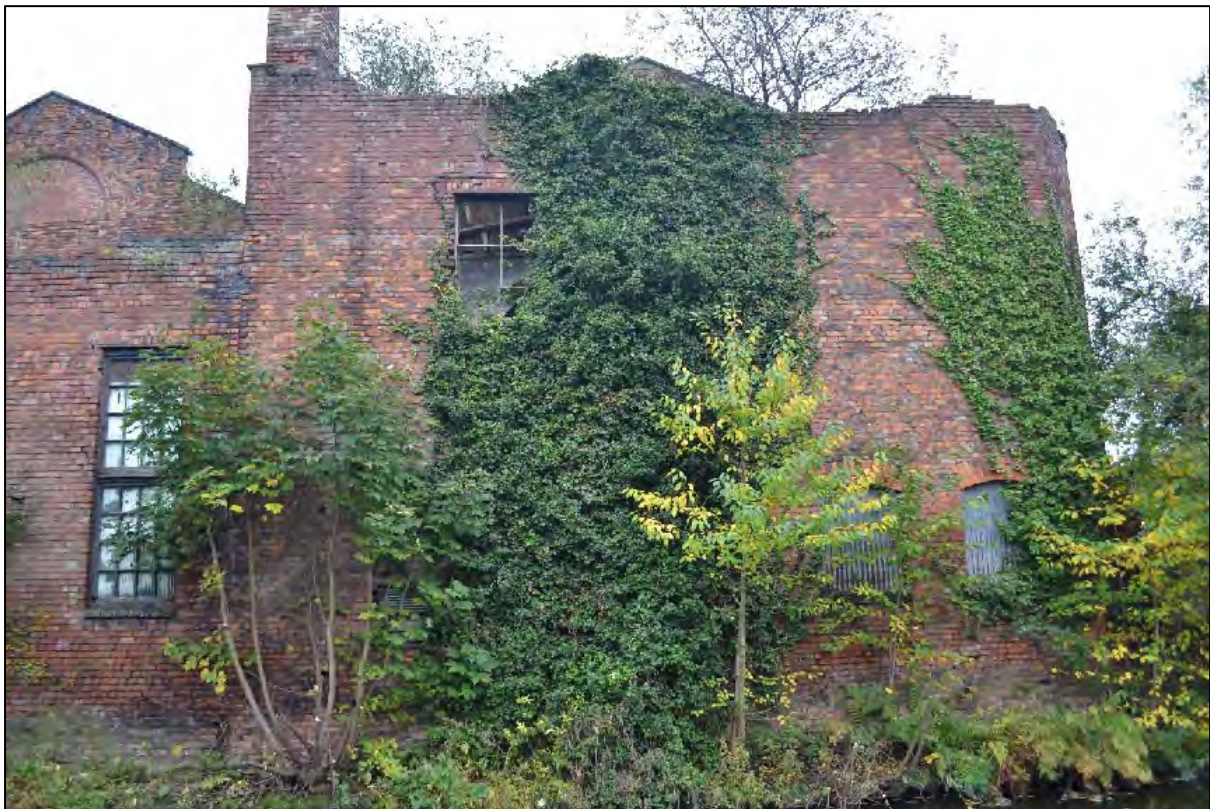
Photograph 30: View south-east of the north-western elevation, Structures D3 and D4
