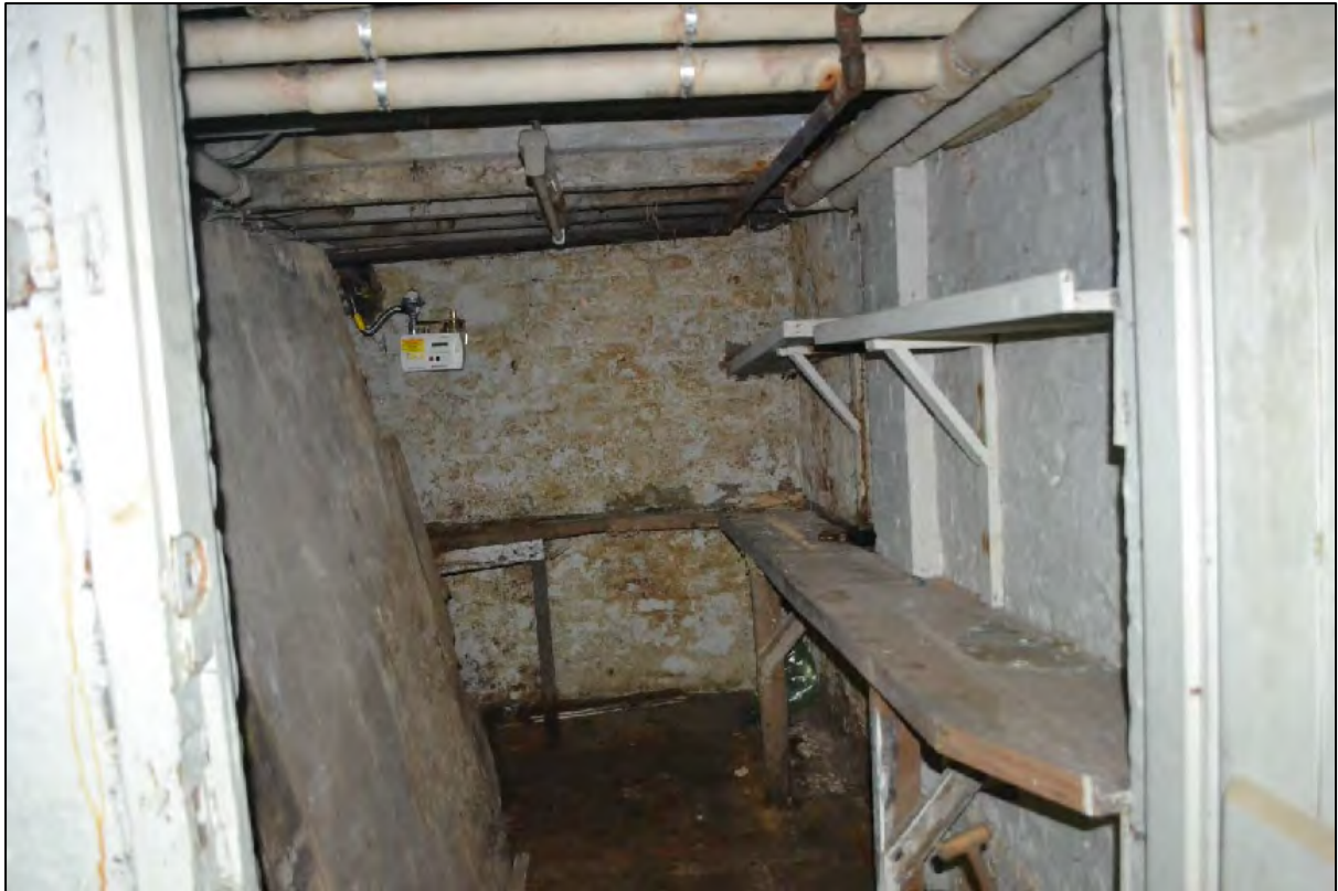
Photograph 127: View south-west of the former spirits room within the cellar
