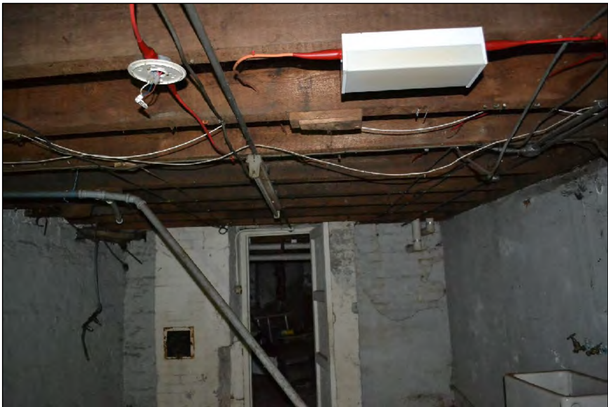
Photograph 126: View north-west of hallway within cellar
