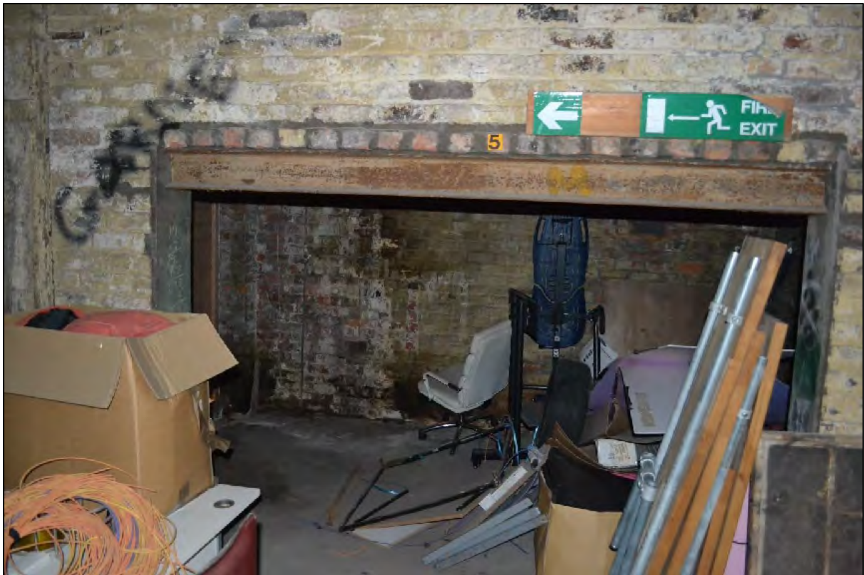
Photograph 83: View south-east from the central room of C4 towards the southernmost room
