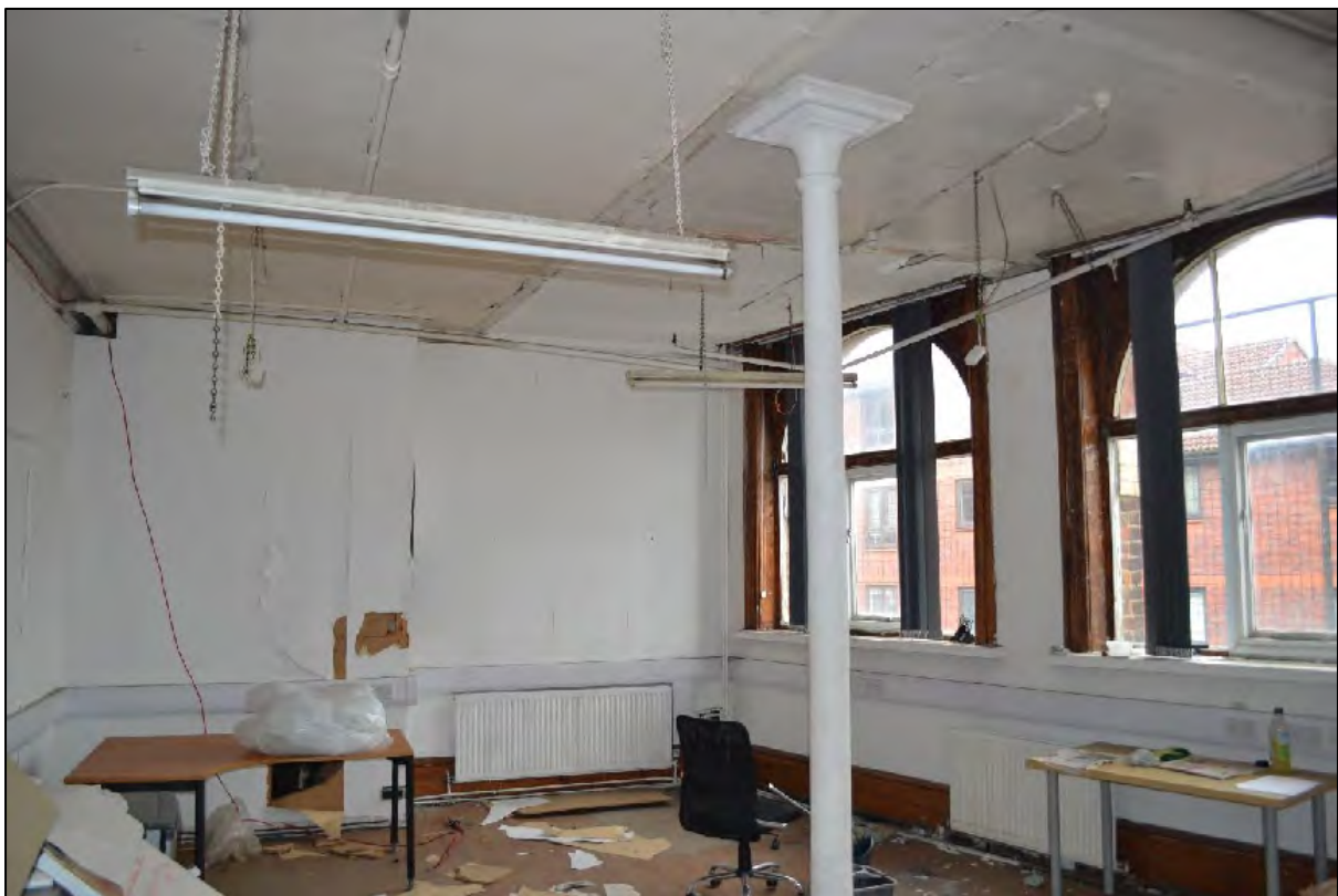
Photograph 50: View north-east within the main first floor office, Structure A
