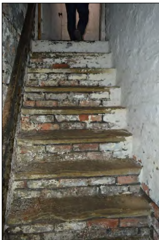
Photograph 123: General view of cellar stairs of Public House
