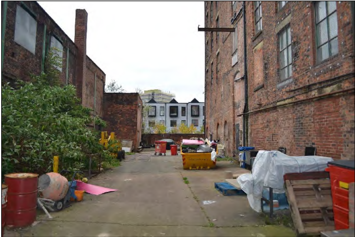
Photograph 133: View north-west from within the courtyard showing the close proximity between the two industrial works
