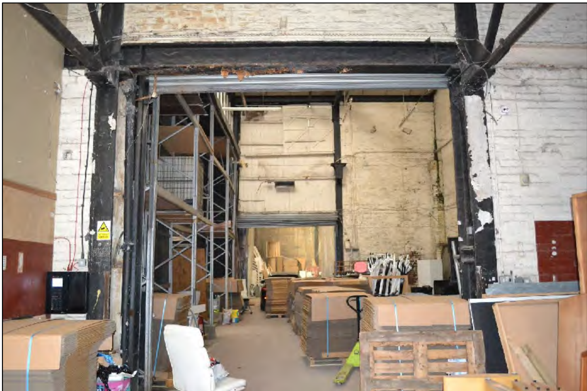
Photograph 104: View of the rolling shutter separating E1 from D1
