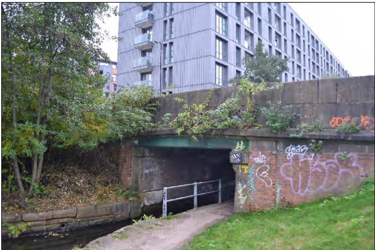
Photograph 138: View of the north-eastern elevation of Bridge Number 4
