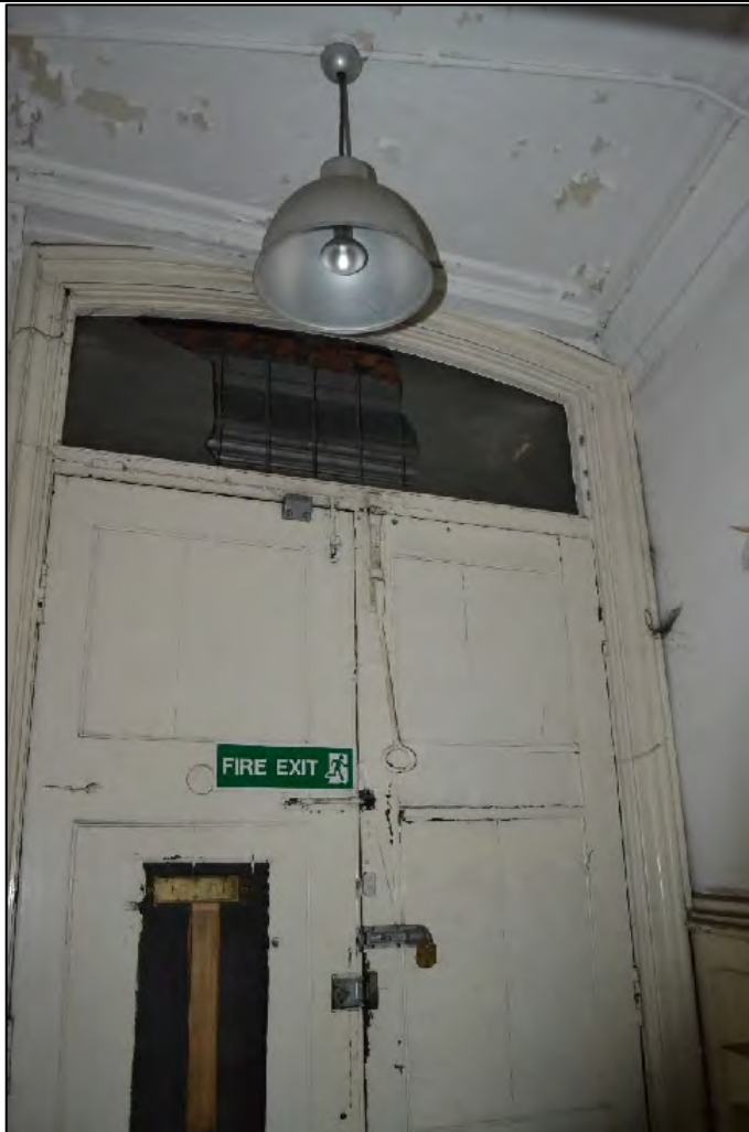
Photograph 41: View south of the Pollard Street entrance to Structure A
