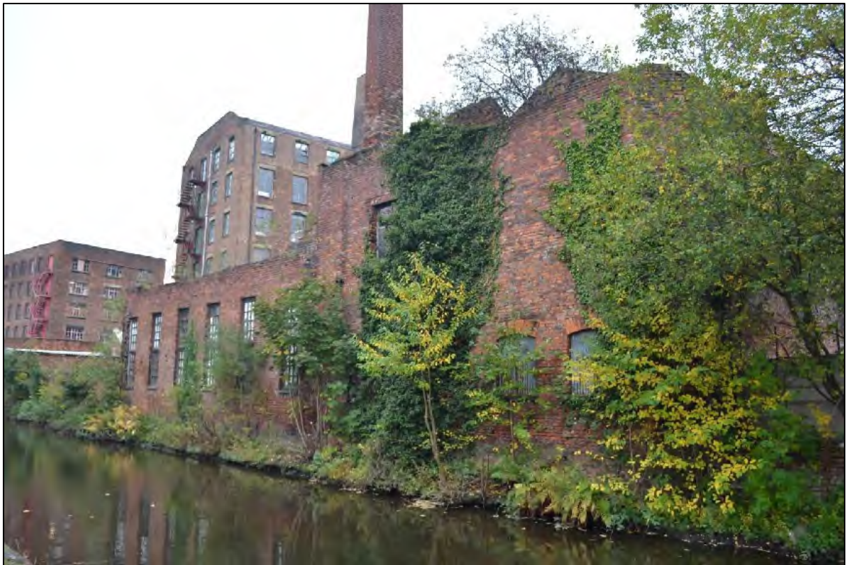
Photograph 31: View east of the north-western elevation, Structures D4, D3 and C5
