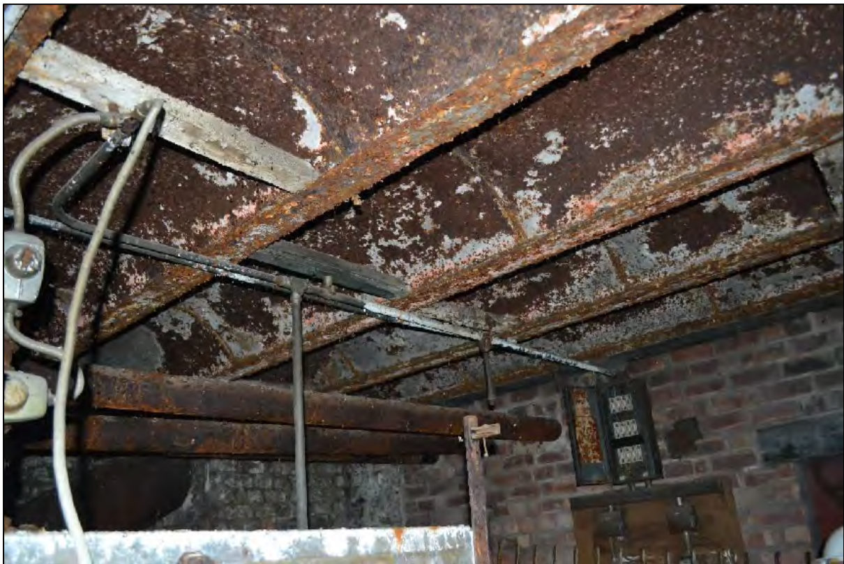
Photograph 100: General view of the metal arched ceiling within the ground floor of D3
