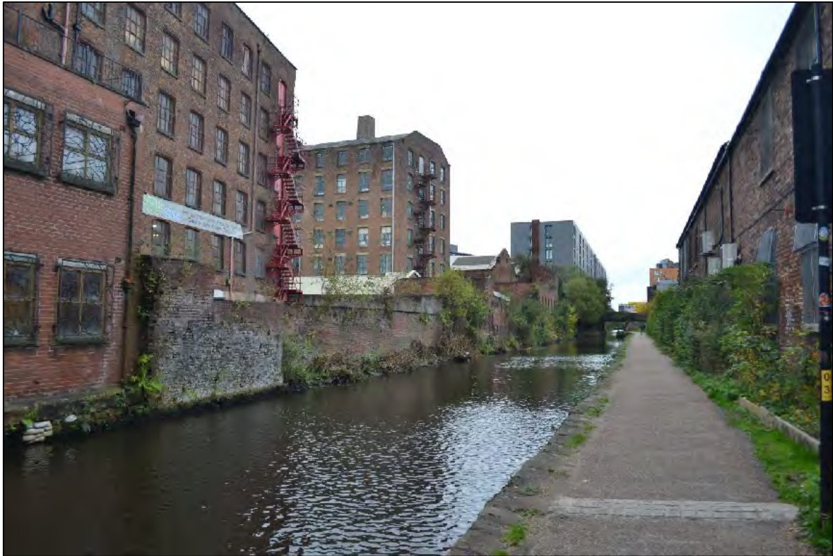
Photograph 145: View south-west along the Ashton Canal from the south-western façade of the Grade II listed Bridge Number 5
