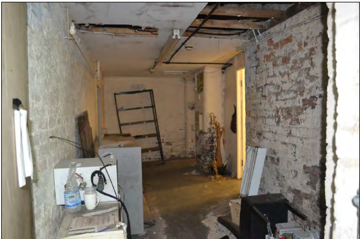
Photograph 62: General view south of hallway within Structure B, which provides access to Structures A and F
