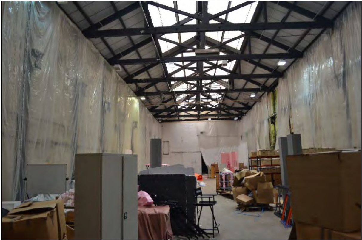
Photograph 67: General view north-west across C2
