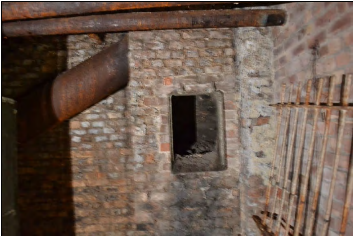
Photograph 103: View of the possible chimney opening within the eastern corner of D3
