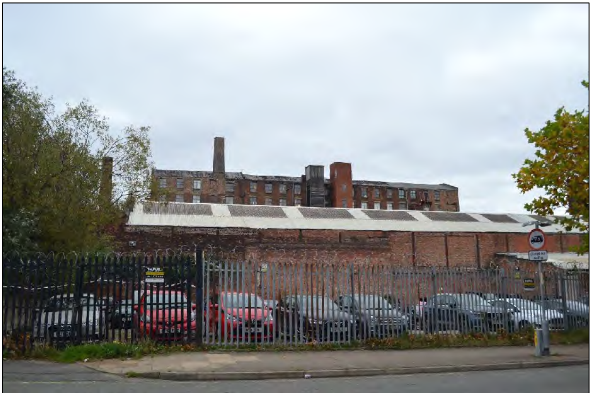
Photograph 32: View east of the south-western elevation, Structures D2 and E2
