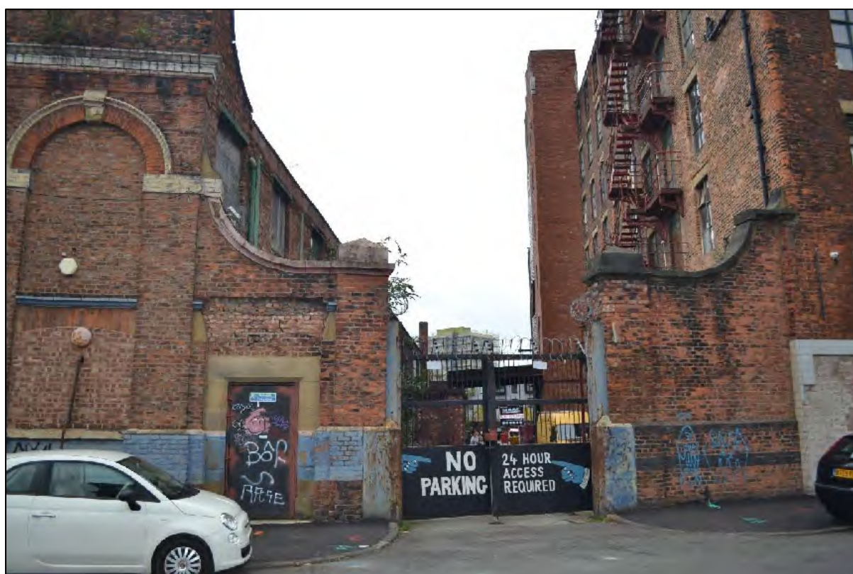
Photograph 132: View north-west of the gated entry to the courtyard between Hope Mill to the right and Ancoats Works to the left
