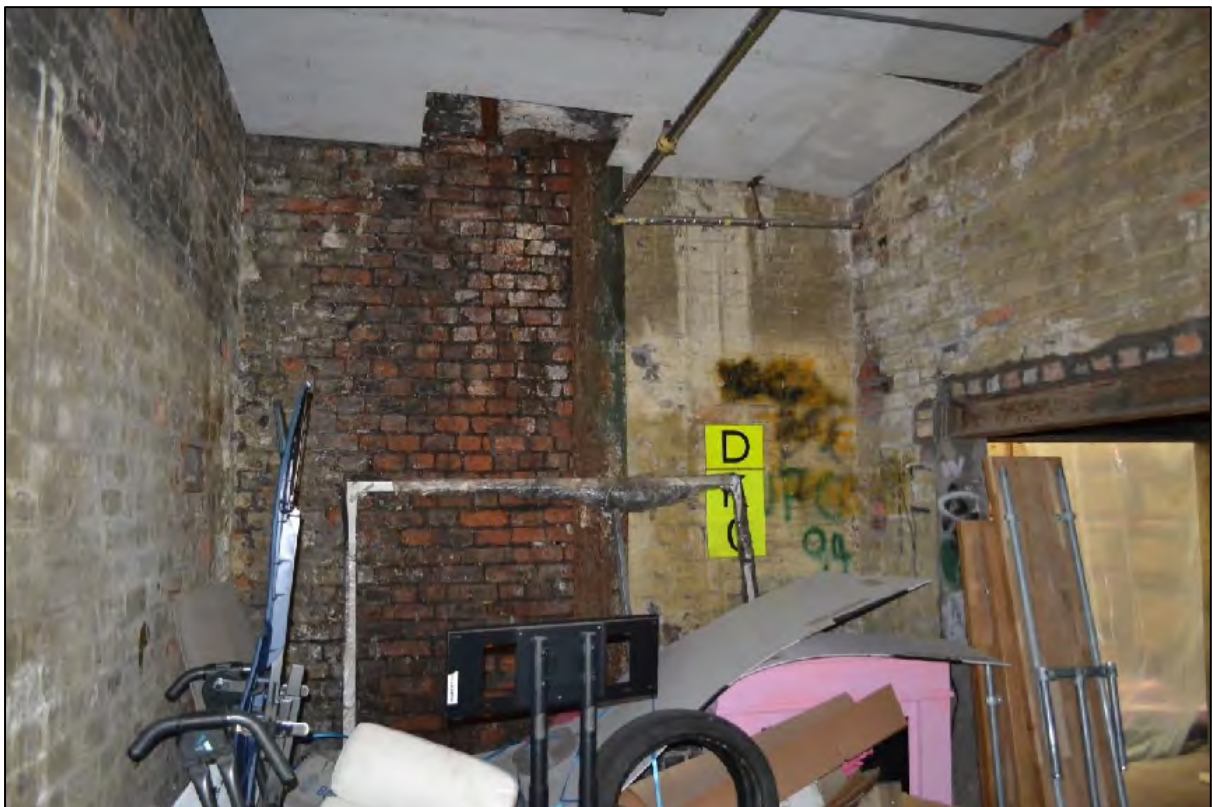
Photograph 82: View south-west within the southern room of C4
