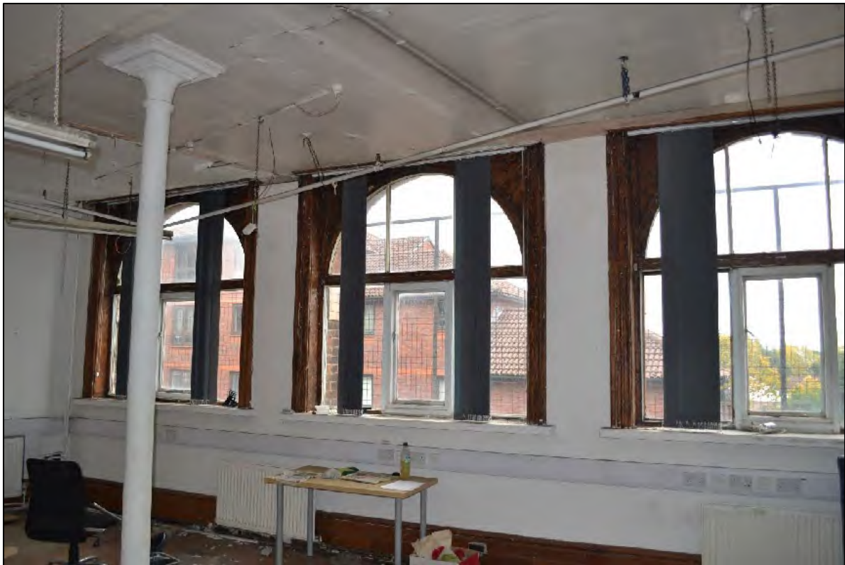
Photograph 49: View east within the main first floor office, Structure A
