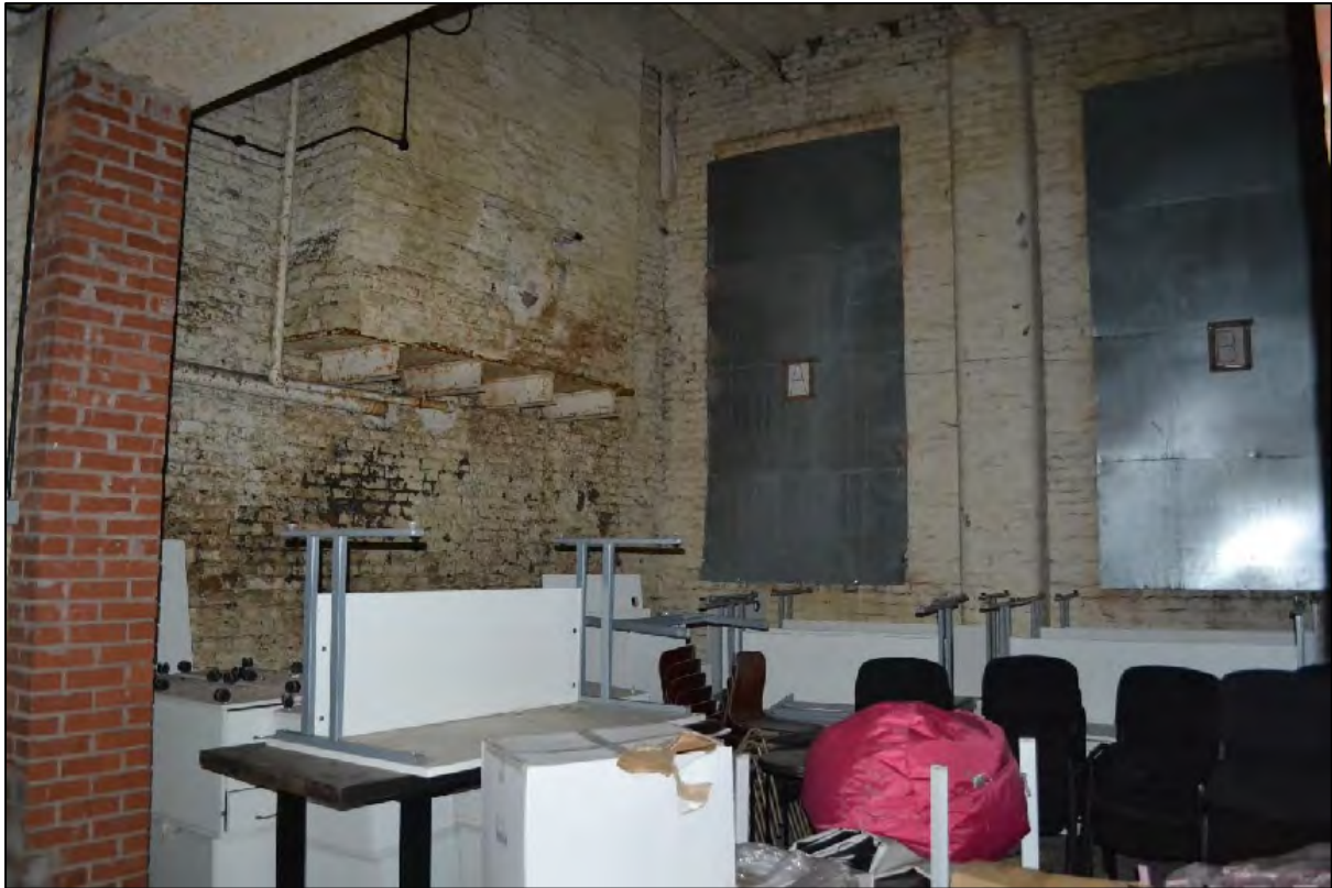
Photograph 87: General view north of C5 from ground floor entrance with C3. Note chimney base along south-western wall
