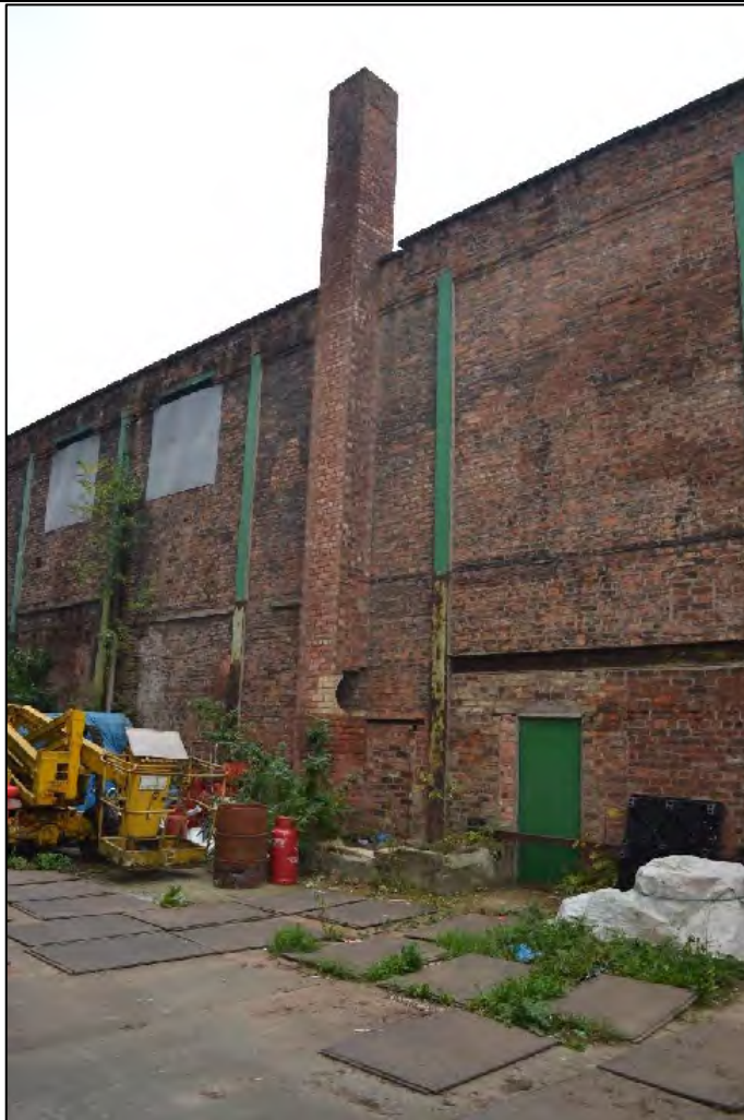
Photograph 25: Detailed view of the chimney stack along the north-western elevation, Structure C2
