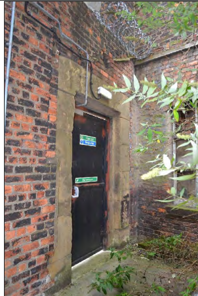
Photograph 22: View of the entrance adjacent the gated courtyard entrance
