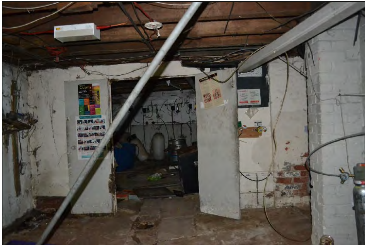
Photograph 124: View south-west across cellar rooms
