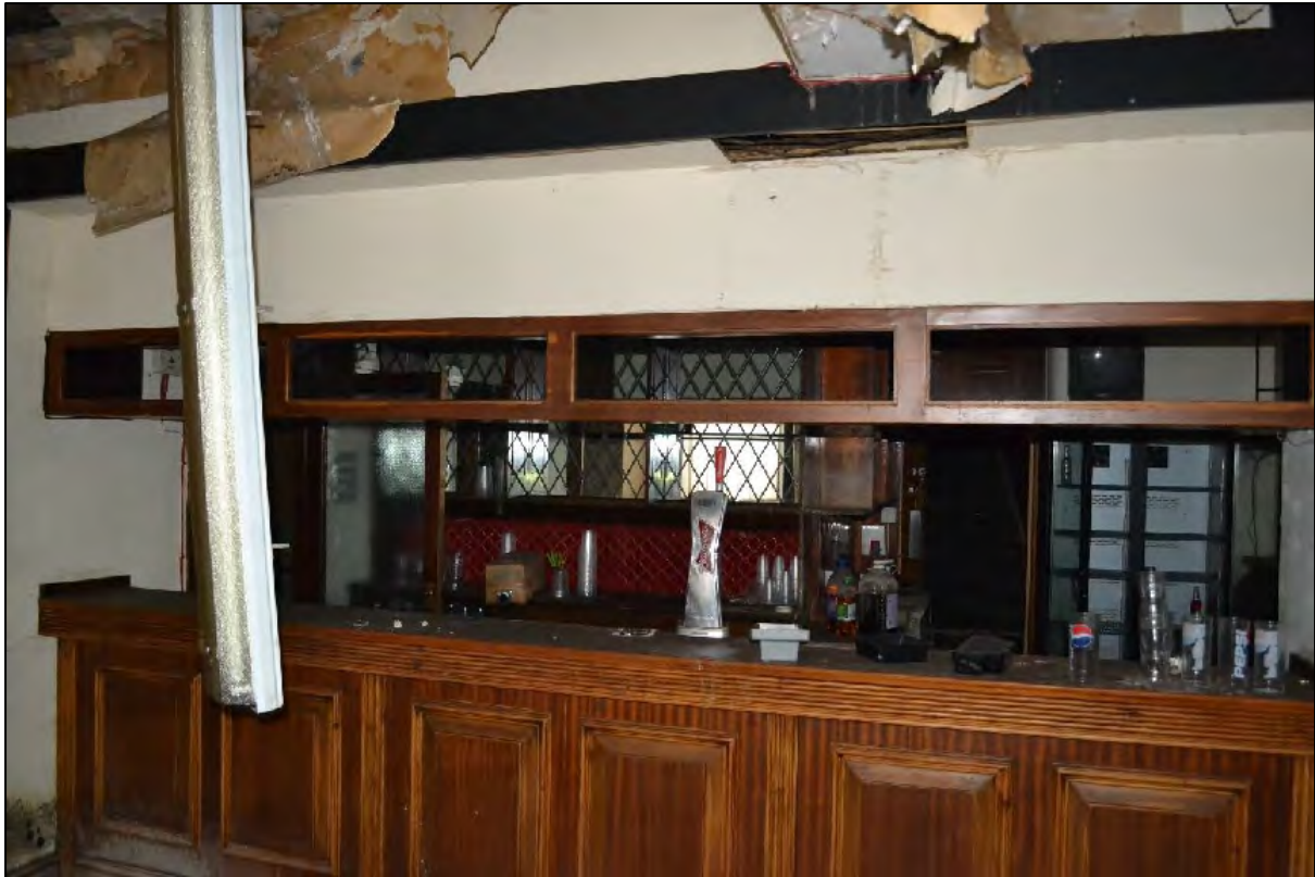
Photograph 115: View north-east towards bar on ground floor of Public House
