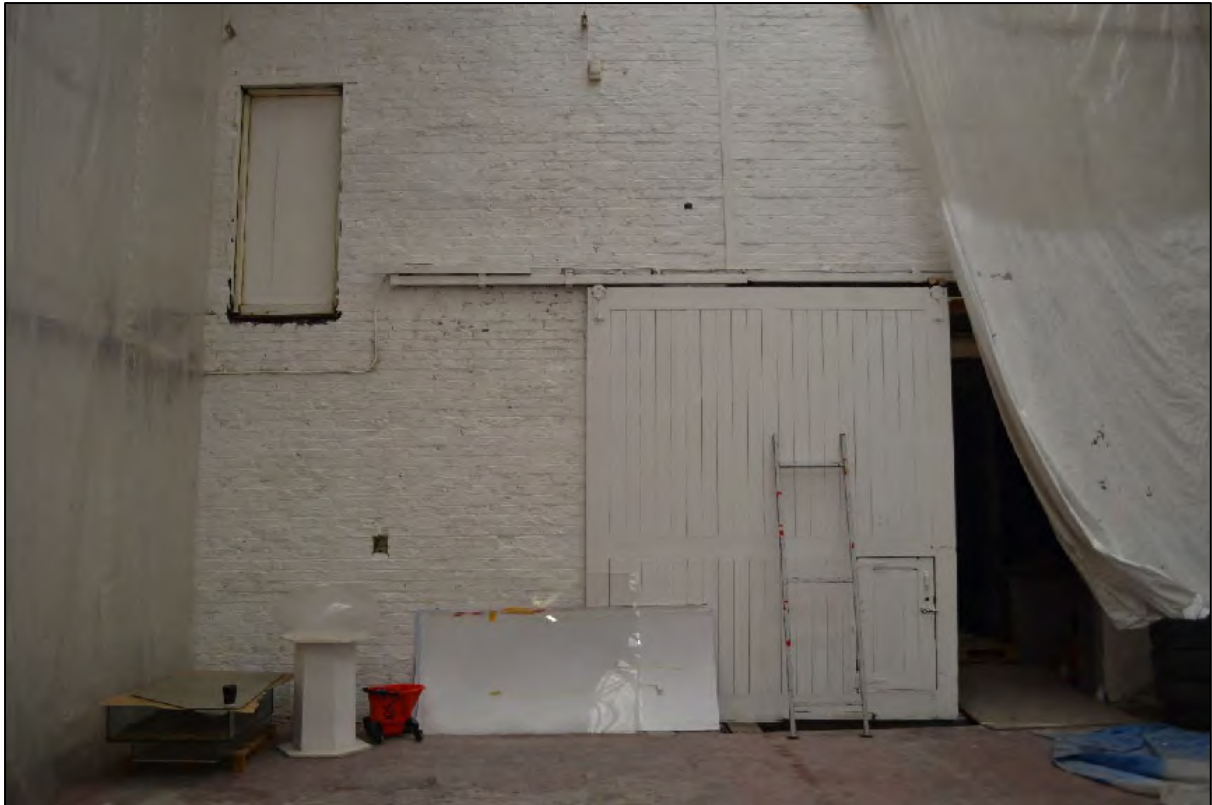
Photograph 69: View north-west of wooden rolling door separating C2 from C3, ground floor and former first floor access doorway
