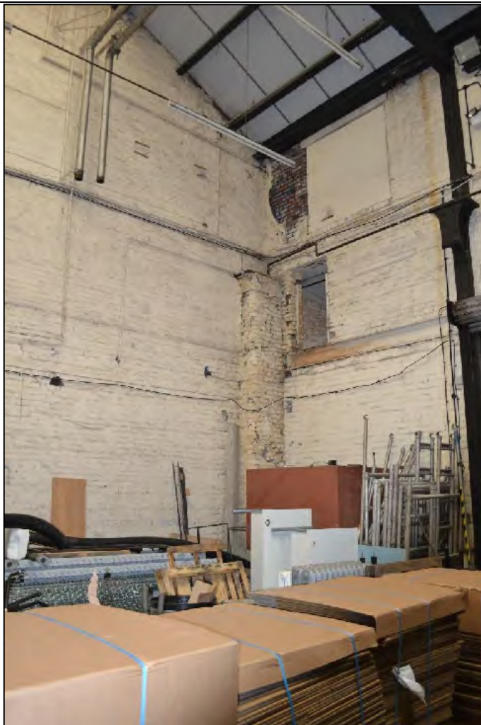
Photograph 89: View south of southern corner of D1 showing former floor entrances along south-western wall
