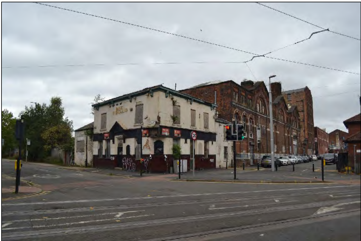
Photograph 134: View from the Carruthers Street and Pollard Street Junctions showing Hope Mill to the rear of Ancoats Works
