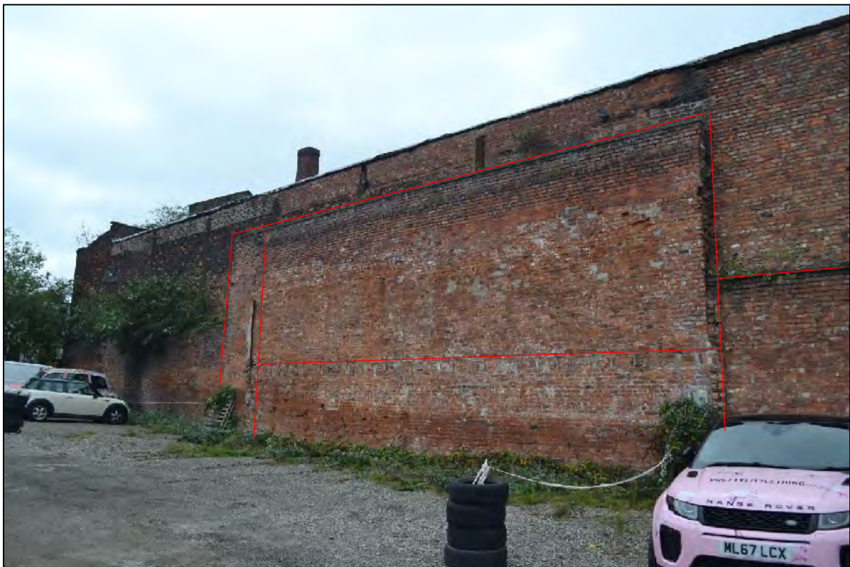
Photograph 38: View north-east of the south-western elevation, Structure D2. Demolished building remnants are visible (red outline)
