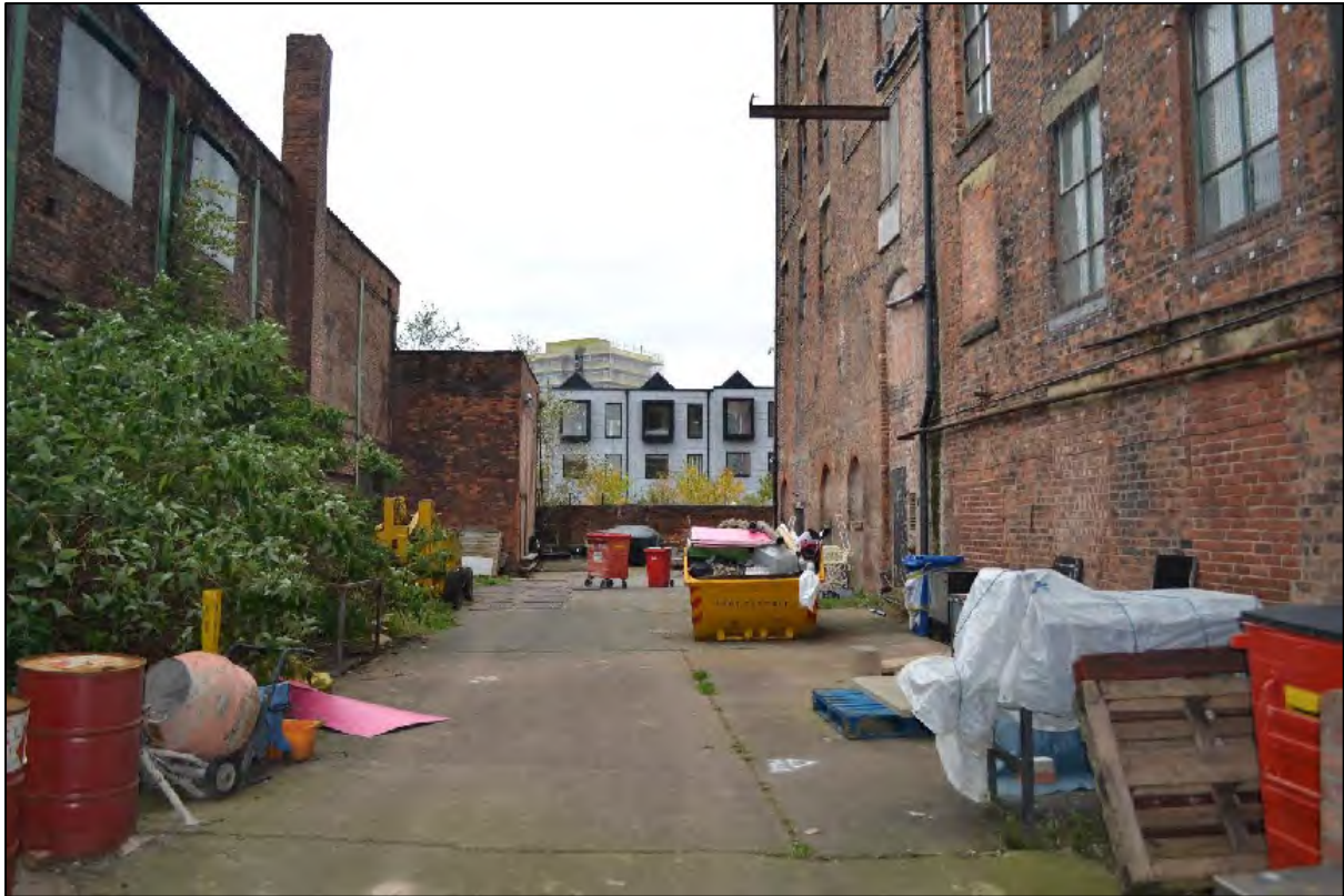
Photograph 23: View north-west along the north-eastern elevation of Structures C2, C3 and C5
