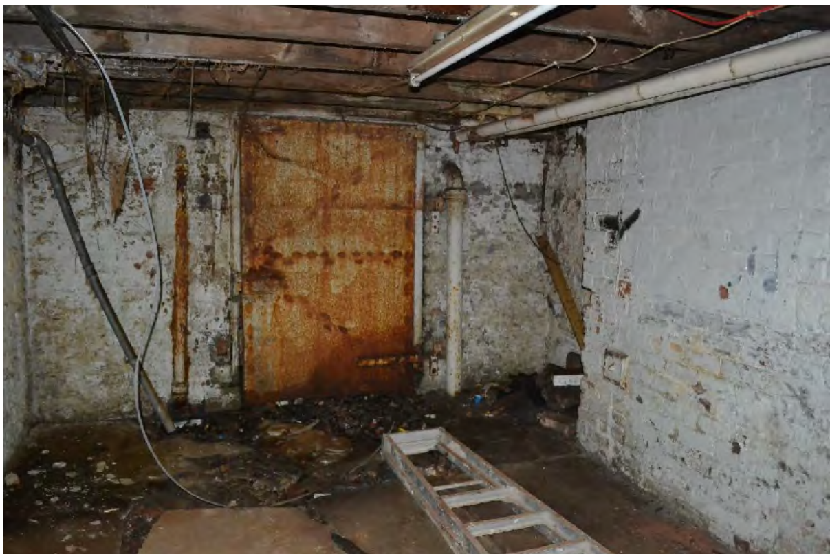
Photograph 130: View north of the former cellar entrance to the ground floor, which allowed for provisions access
