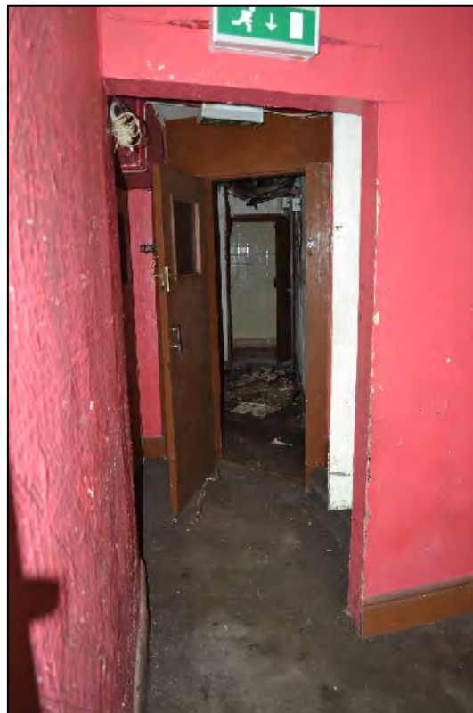
Photograph 122: View north along hallway leading to toilets in the northern half of the ground floor of the Public House
