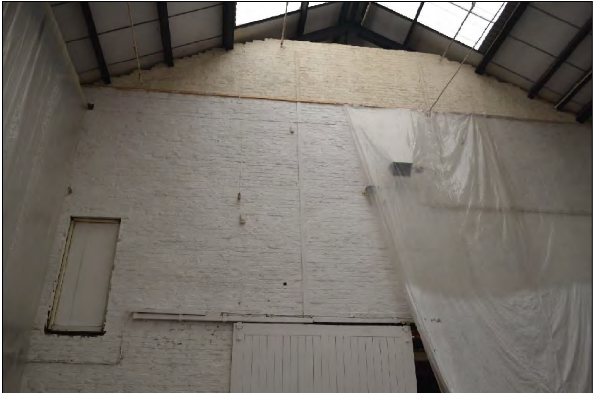
Photograph 71: General view of the separating wall between C2 and C3, showing the possible later northern addition to the top of the separating wall
