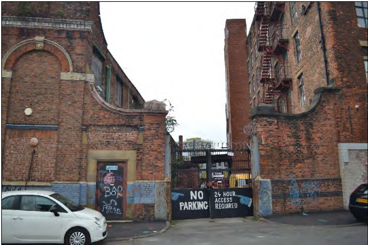
Photograph 17: View north-west of the gated entrance between Ancoats Works and Hope Mill
