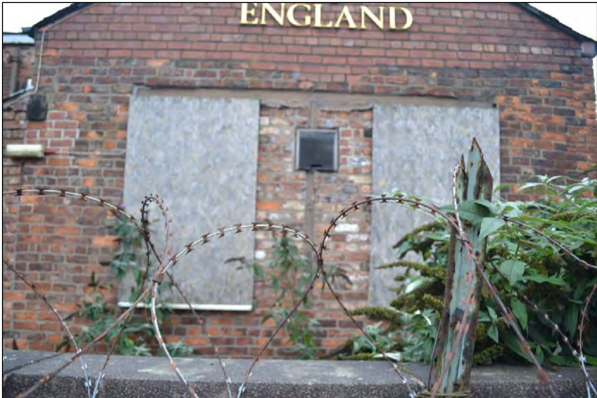
Photograph 111: Detailed view of the north-western façade of the Bank of England Public House
