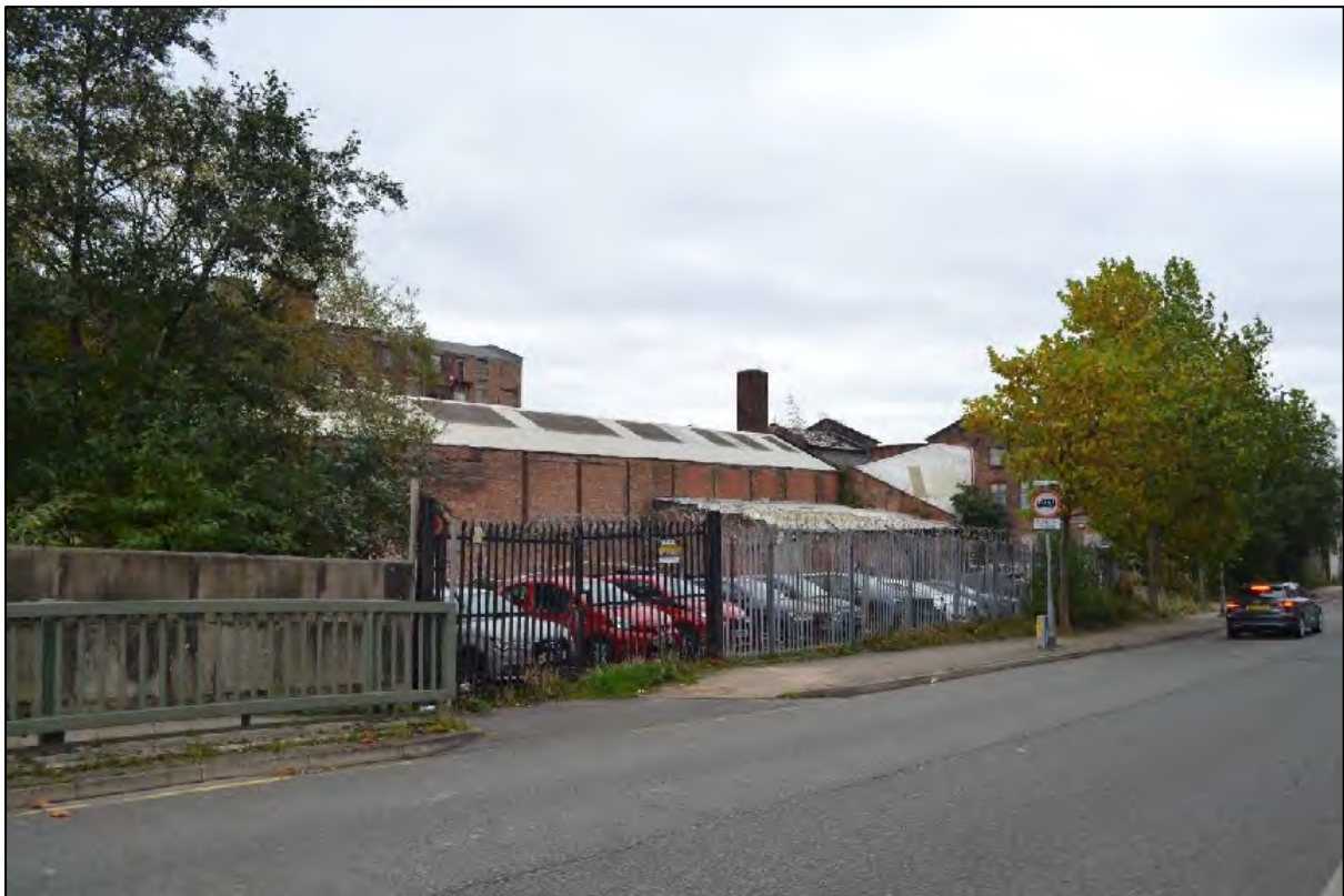
Photograph 140: View from the top of the listed Bridge Number 4 towards the PDA
