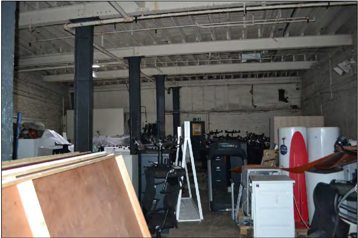
Photograph 59: General view south-west within ground floor of Structure B
