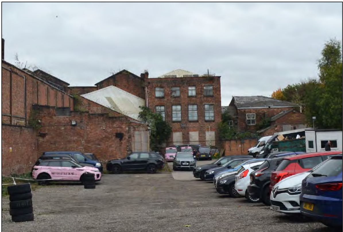
Photograph 40: General view south-east of the south-western and north-western elevations
