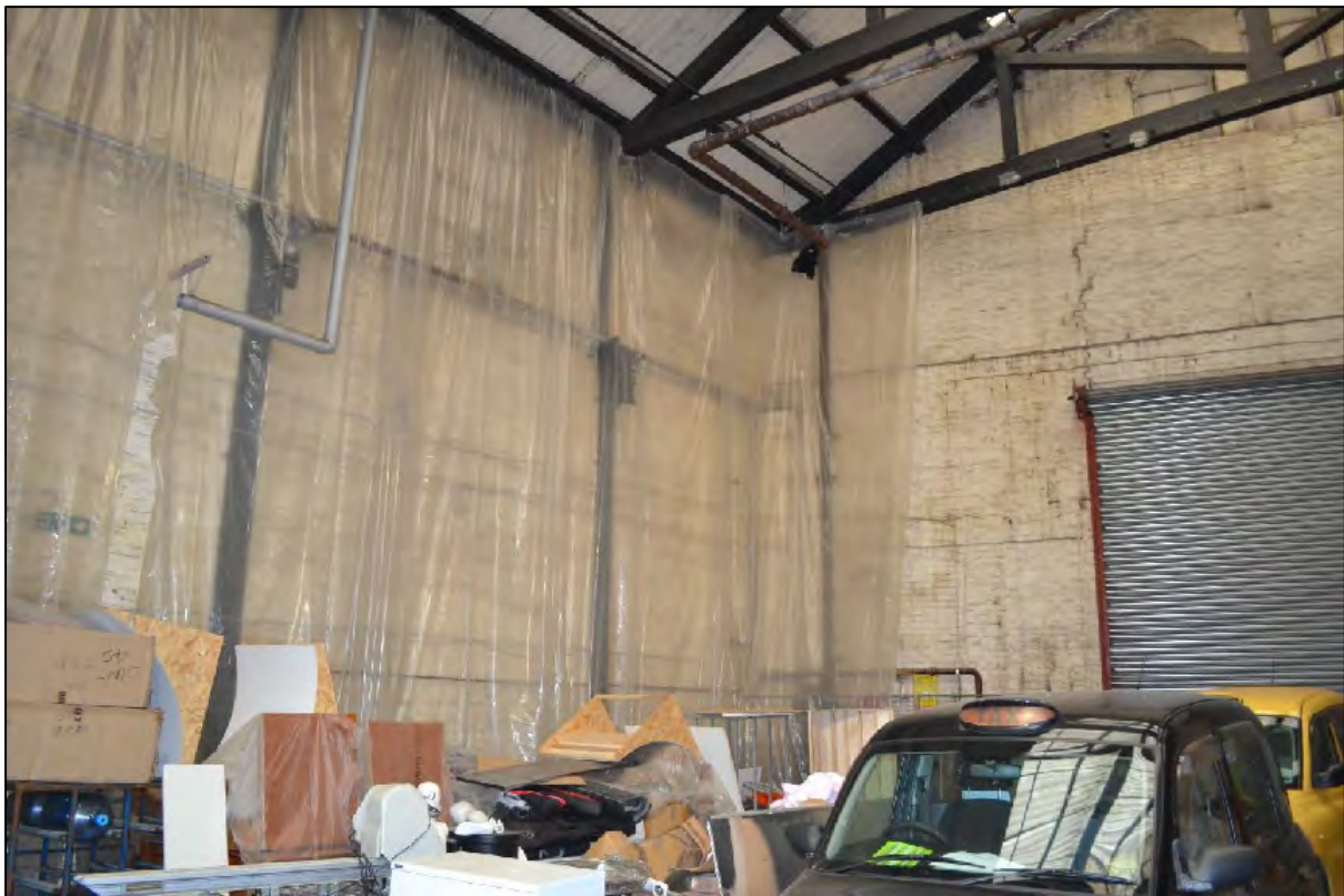
Photograph 66: View east within C1 showing extant columns covered with plastic
