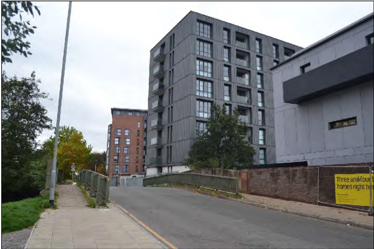
Photograph 139: View from Carruthers Street across the listed Bridge Number 4
