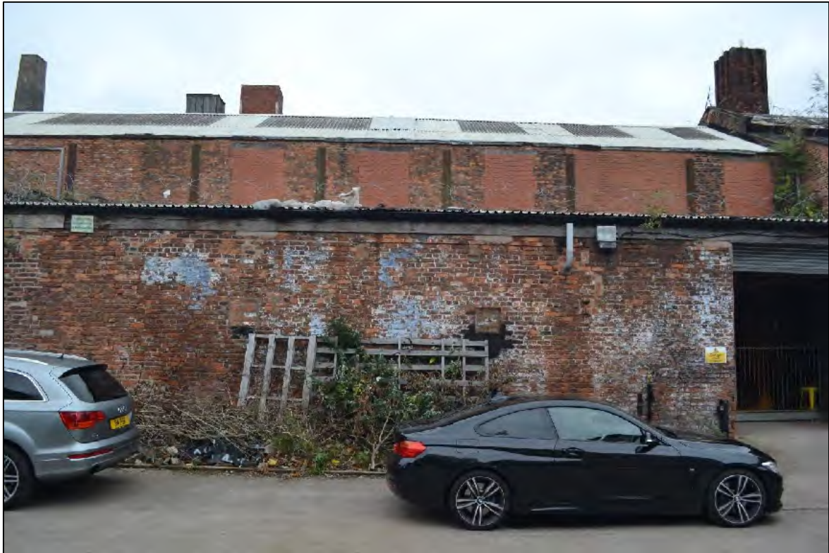
Photograph 35: View east of the south-western elevation, Structures D2, E2 and E1
