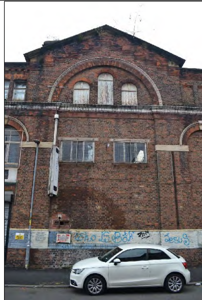
Photograph 14: View north-west of the Pollard St exterior of Structure B
