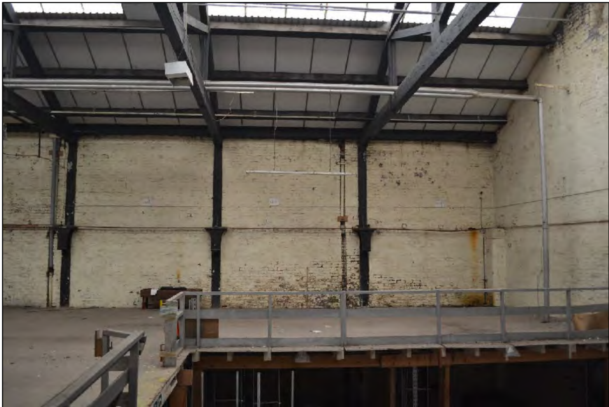
Photograph 95: View south-west of the south-western wall of D2
