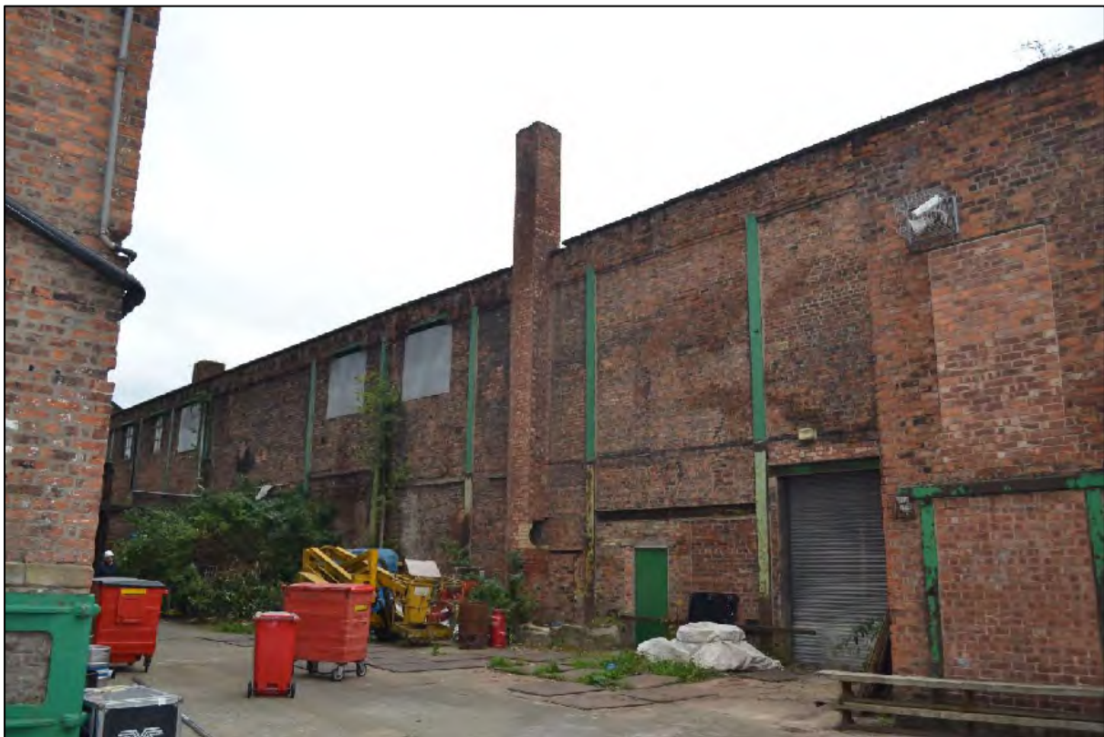
Photograph 24: View west of the north-eastern elevation of Structures C2, C3 and C5
