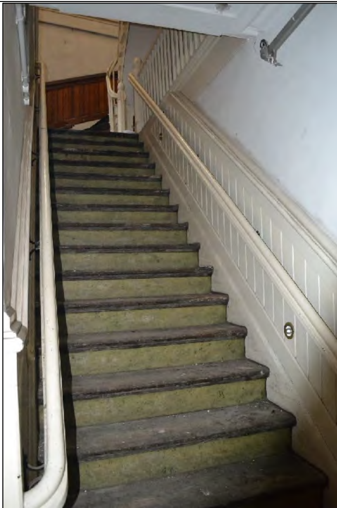
Photograph 47: View west of the wooden staircase leading from Structure A's ground floor to first floor
