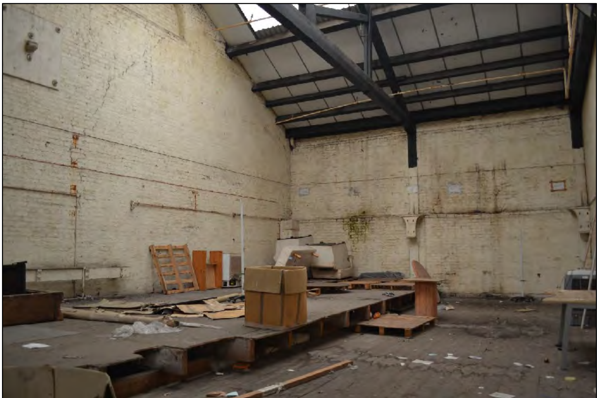
Photograph 76: View east across the first floor of C3
