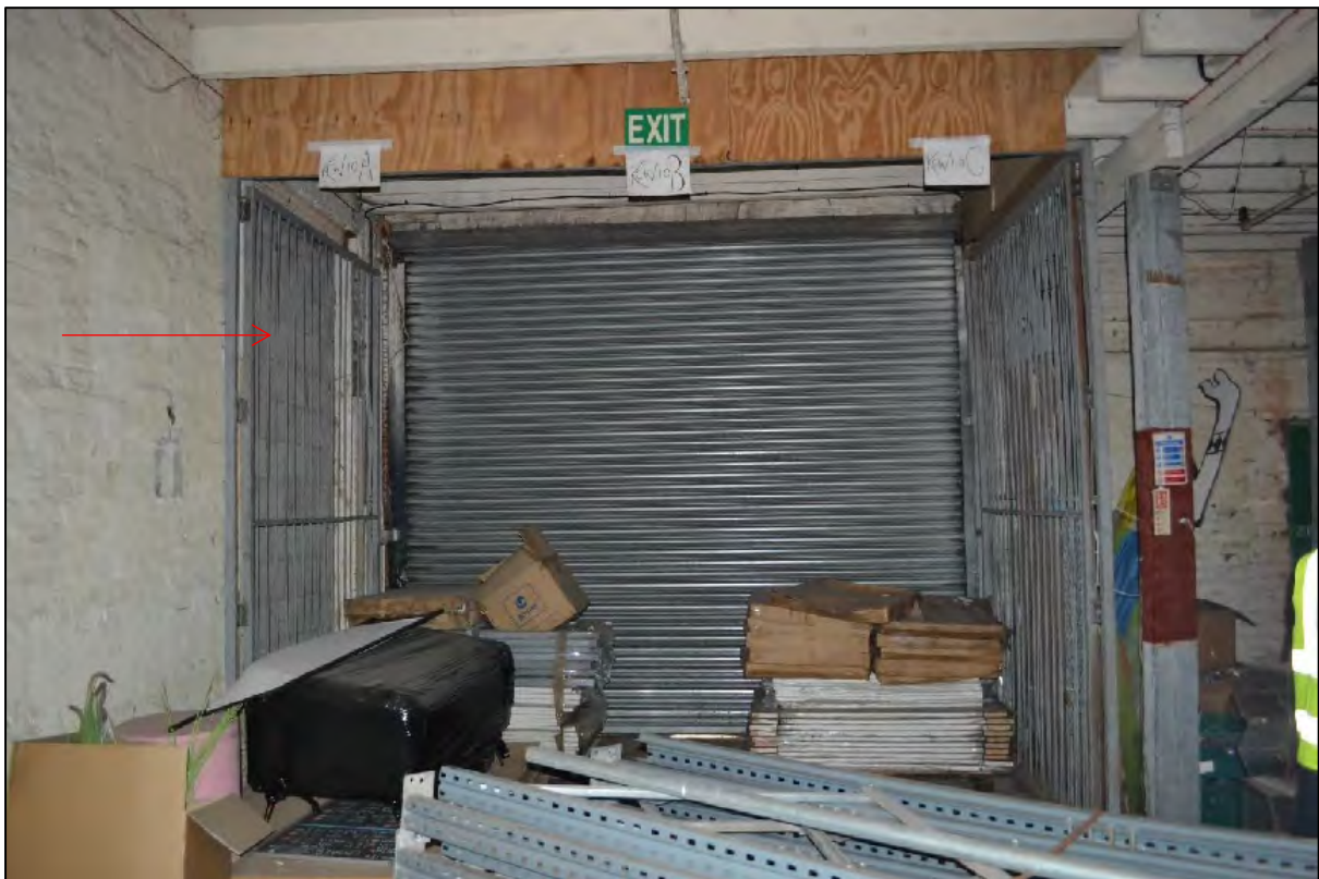
Photograph 86: View northeast within C3 showing the rolling shutter leading to the courtyard and the blocked door to C5 (red arrow)
