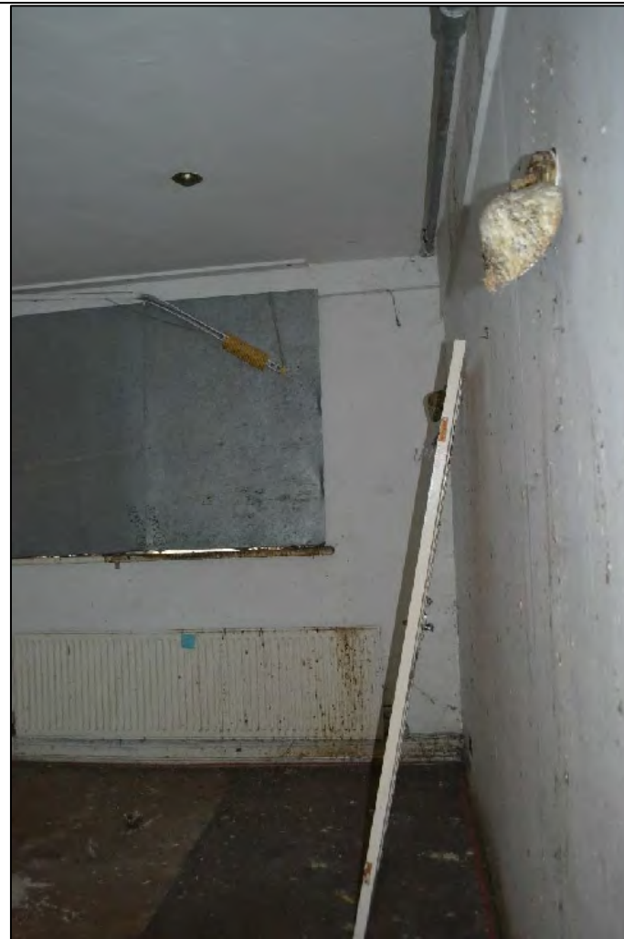
Photograph 56: View south-east of second floor office, Structure A
