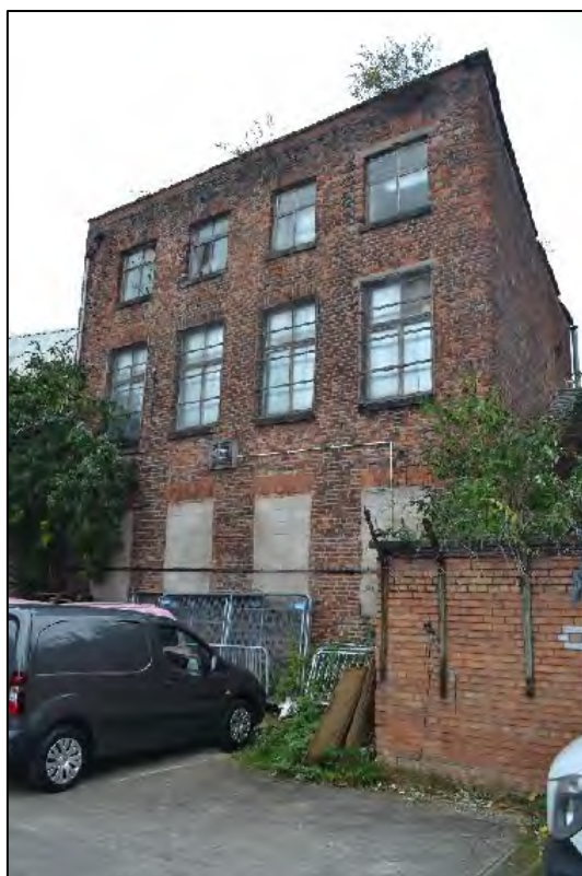
Photograph 33: View of the north-western elevation of Structure A
