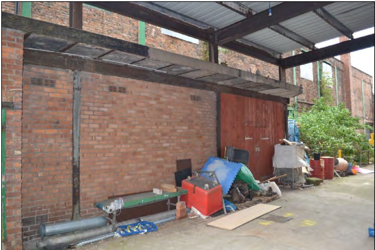
Photograph 81: View north-west of the north-eastern elevation of C4
