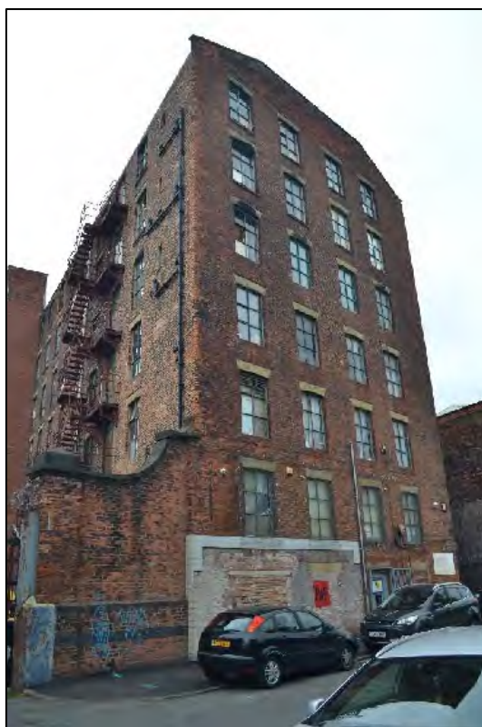
Photograph 131: View of the south-east Pollard Street elevation of Hope Mill
