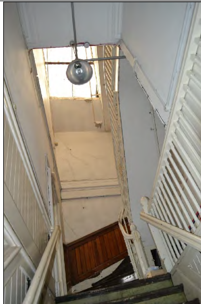
Photograph 48: General view of the open plan of the staircases across all floor levels within Structure A
