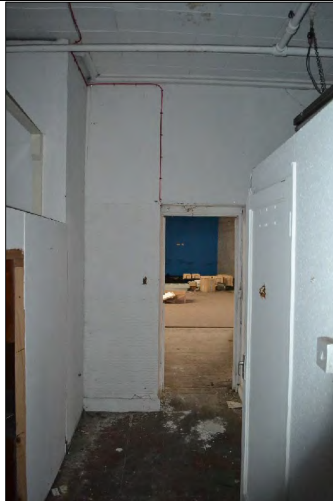
Photograph 52: View north-east along the first floor corridor in Structure A towards the entrance to Structure B
