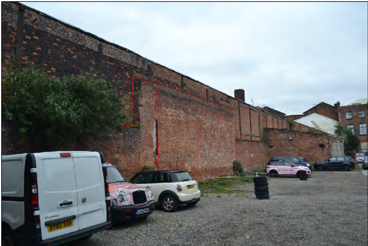
Photograph 39: View east of the south-eastern elevation, Structure D2, former buildings outlined in red
