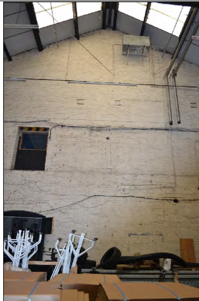
Photograph 90: General view of south-eastern wall of D1
