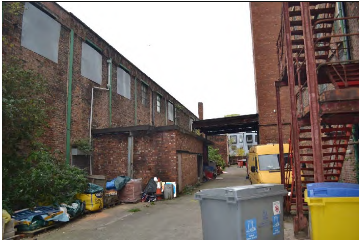
Photograph 78: View north-west of the south-eastern elevation of C4
