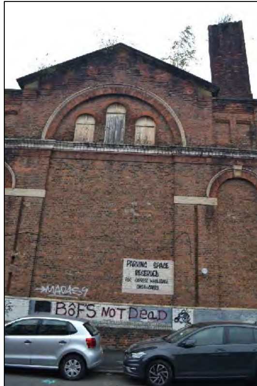
Photograph 15: View north-west of the Pollard St exterior of Structure B
