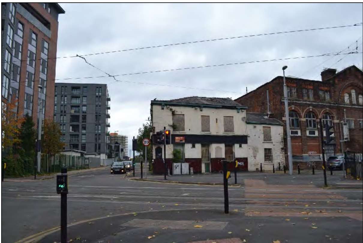
Photograph 2: View north-west along Carruthers Street
