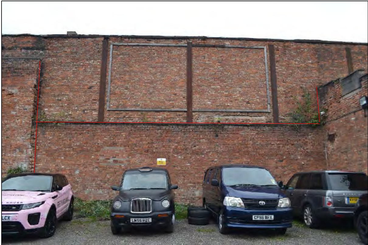
Photograph 37: View north east of south-western elevation, Structure D2. Demolished building remnants are visible behind the cars (red outline)
