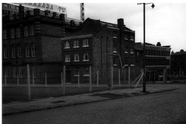
Figures 14: A view looking north along Lower Byrom Street towards its junction with Great John Street in 1964, showing the demolition of all buildings to the north and east sides of the Site by this time. The building to the left is now the Grade II listed Great John Street Hotel.
