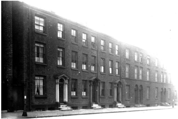
Figures 11: A view looking west along Great John Street in 1944, showing the early-19 th century houses that formed the northern perimeter of the Site.
