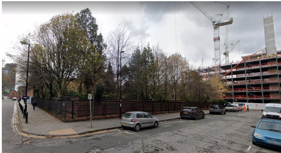
Figure 3: Looking west along Great John Street, showing the land at Atherton Street to the left.
