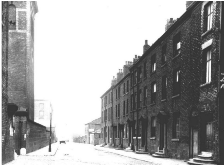
Figures 10: A view looking west along Grape Street from its junction with Lower Byrom Street (now private) in 1944, showing the early 19th century housing to the right side, which formed the southern boundary of the Site.
