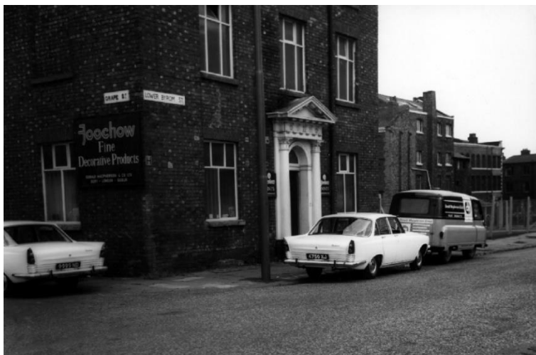
Figures 12: A view looking north along Lower Byrom Street (right), at its junction with Grape Street (left) in 1964, showing one of the few remaining buildings on the site (left) shortly before demolition.
