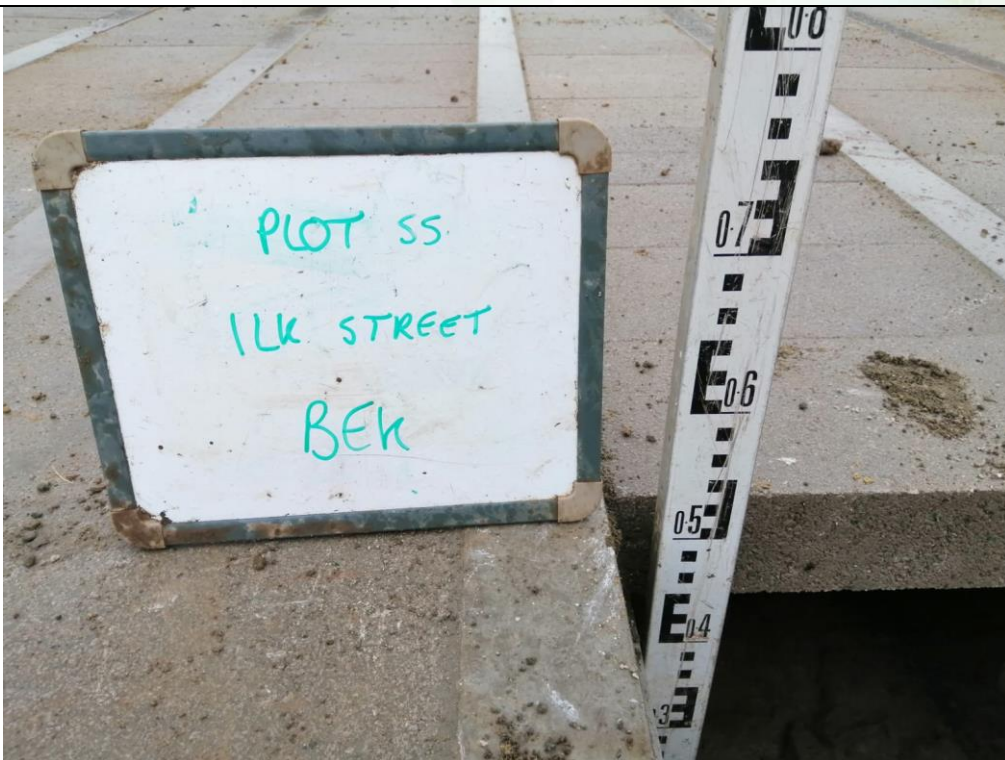
Photograph 4: Validation of Sub-Floor Void Space (min 150 mm)
