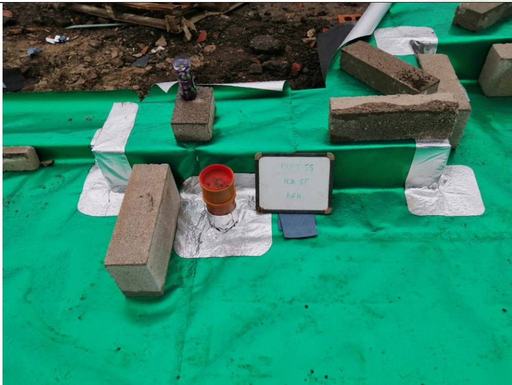
Photograph 8: Validation of Gas Membrane Installation
