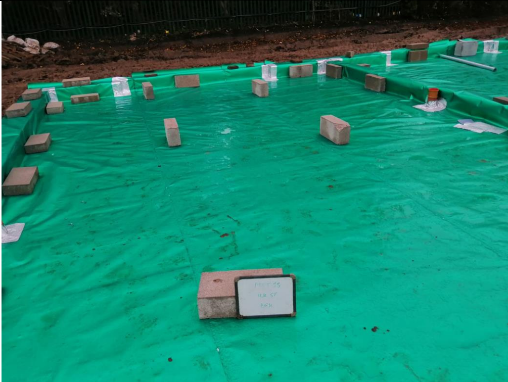
Photograph 5: Validation of Gas Membrane Installation
