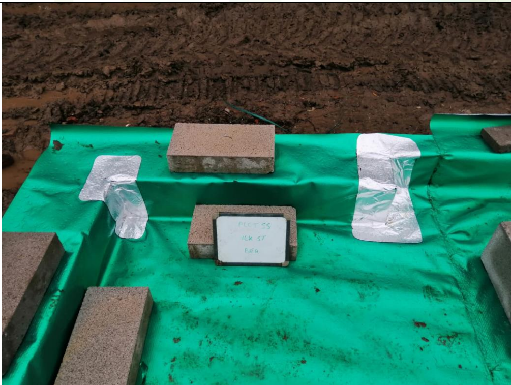
Photograph 6: Validation of Gas Membrane Installation
