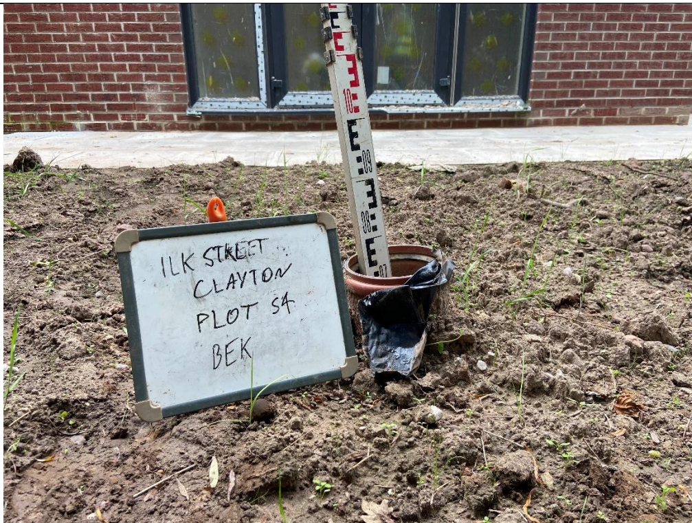
Photograph 1: Validation of Garden Capping Thickness (Plot 55, not 54)
