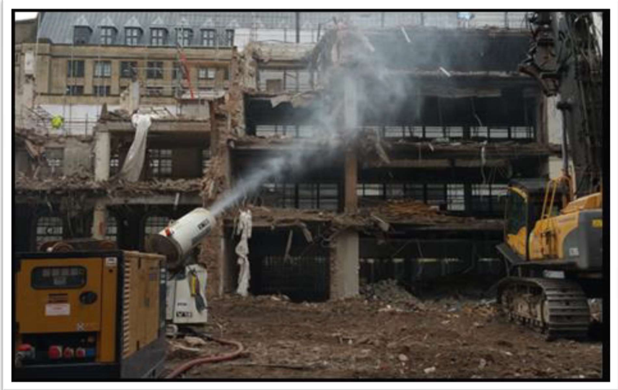
Typical View of Dust Suppression During Demolition Works
