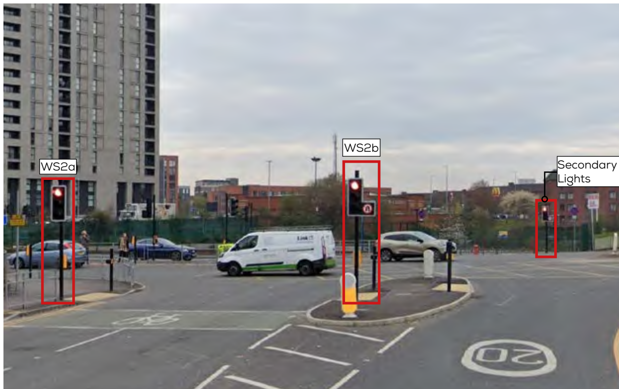
Fig. 154: Traffic Light Location
