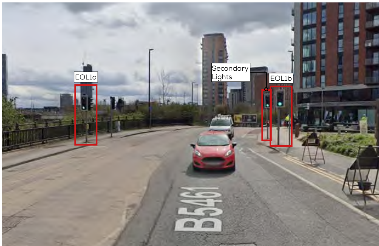
Fig. 35: Traffic Light Location
