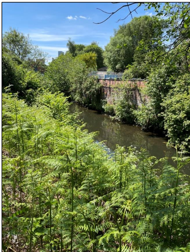
Figure 6: Downstream view of Reach 2 showing the brick wall on the right bank of the modified urban reach.
