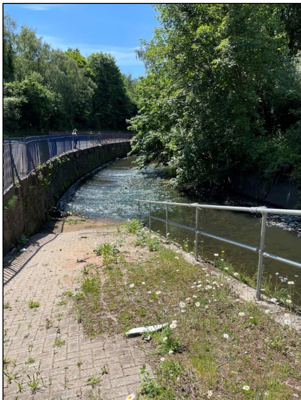
Figure 9: Downstream view of Collyhurst Weir (this is the upstream-most extent of Reach 3), showing flow types behind the weir which are sequences of runs and glides.
