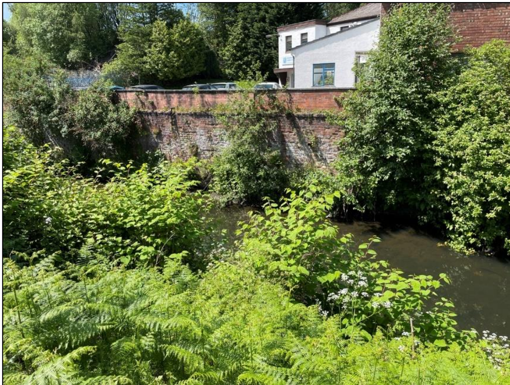
Figure 8: Right bank of Reach 2, showing a brick wall.
