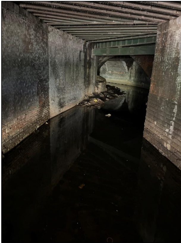
Figure 20: Culvert upstream of Scotland Weir
