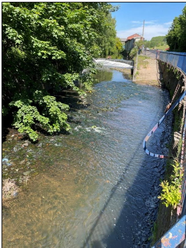
Figure 12: Looking upstream from Reach 3 to the boundary near Reach 2 (Collyhurst Weir)
