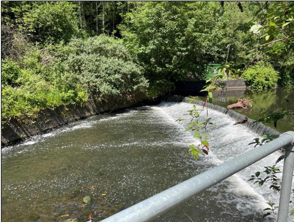
Figure 10: Upstream view of Reach 2 showing Collyhurst Weir.
