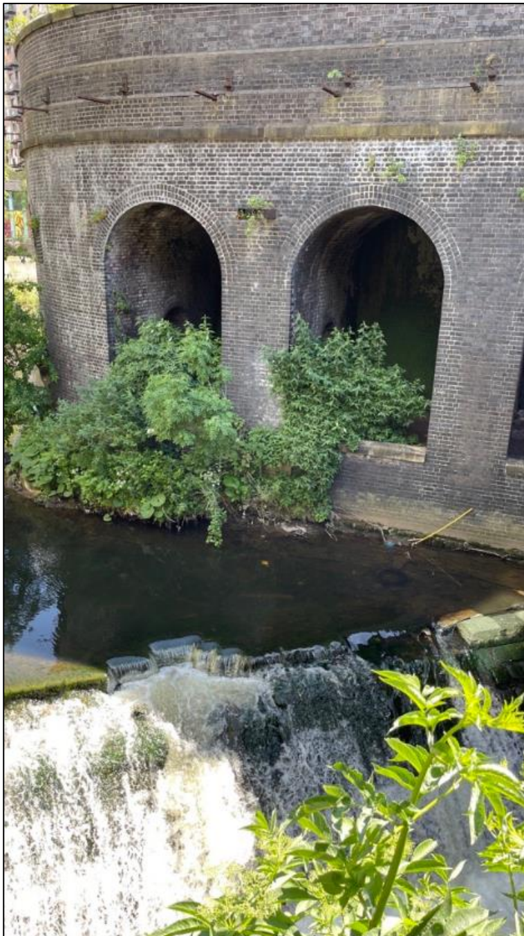
Figure 24: Scotland Weir, the downstream end of Reach 5 and the survey area.
