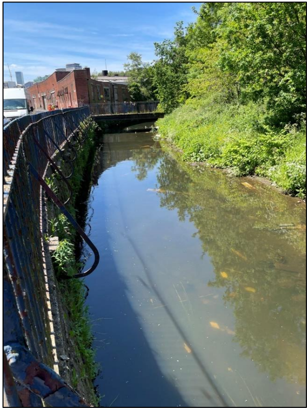
Figure 13: Downstream view of Reach 3 showing footbridge across the river.
