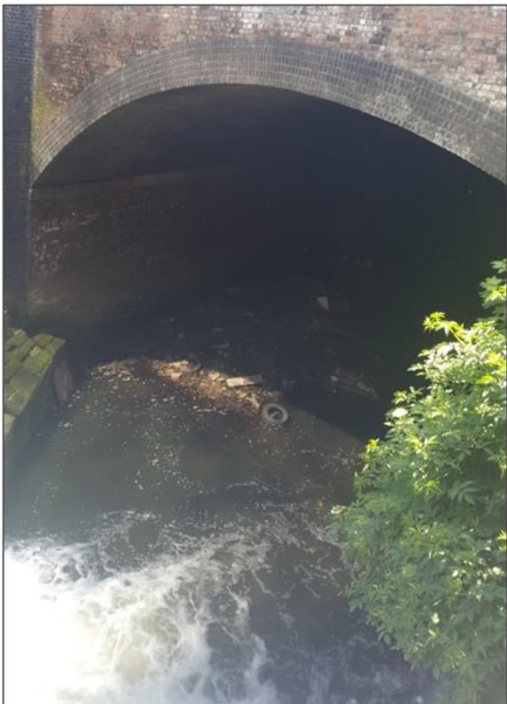
Figure 23: Bar under bridge d/s of Scotland Weir
