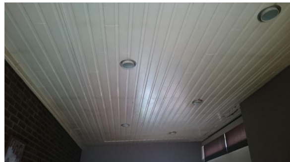
Photograph 4 Ceiling of main building, with no loft space
