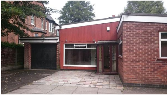
Photograph 1 Front view of building from the north
