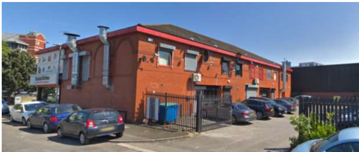
Figure 2. There is staff off-road parking to the rear of the premises
