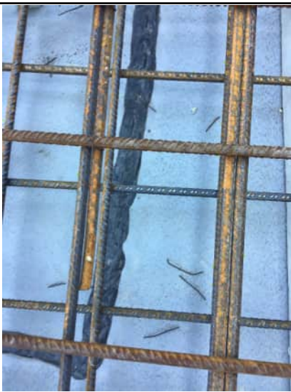
Extrusion weld on Visqueen
