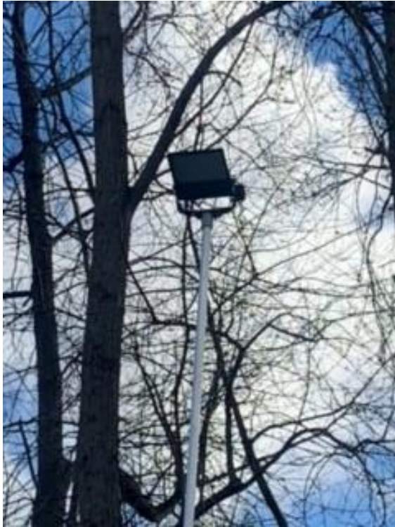
Single Lighting Column
