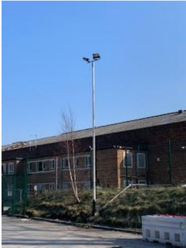
Existing Lighting Column
