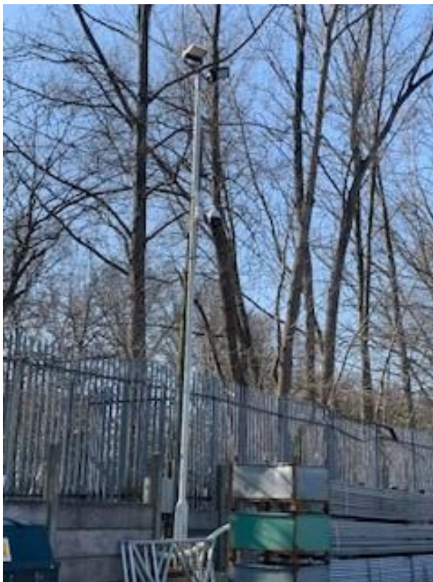
Existing Lighting Column
