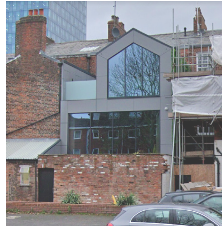
15 St. John street rear extension
