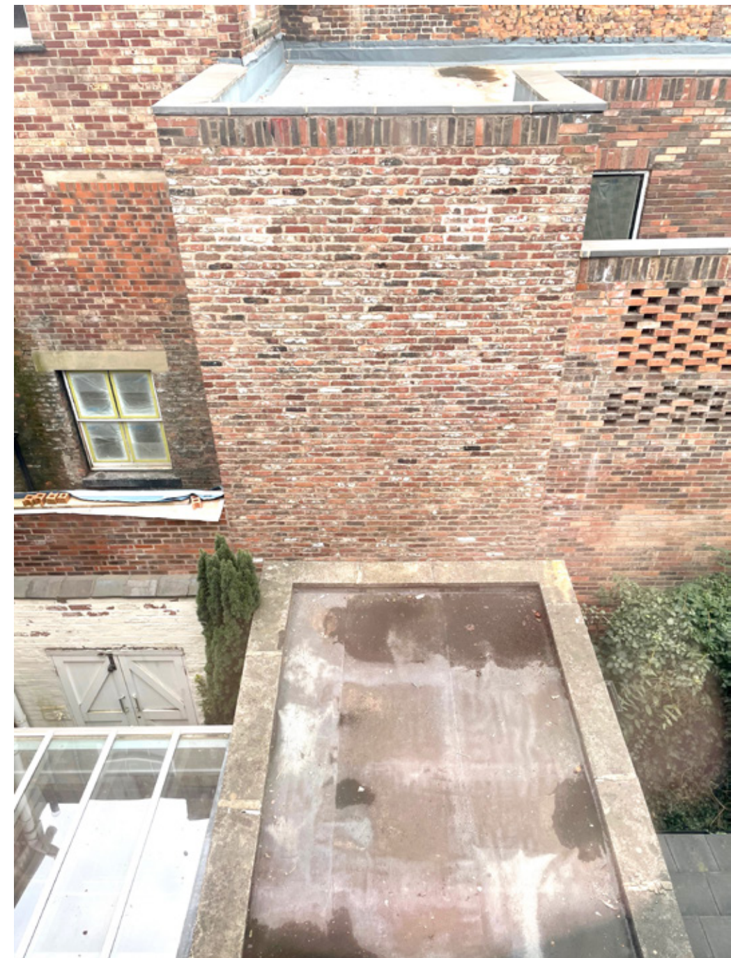
View from the second floor window of 27 Byrom Street Looking at the existing single story flat roof extension to 27 Byrom Street and the blank elevation of 21 St. John Street
