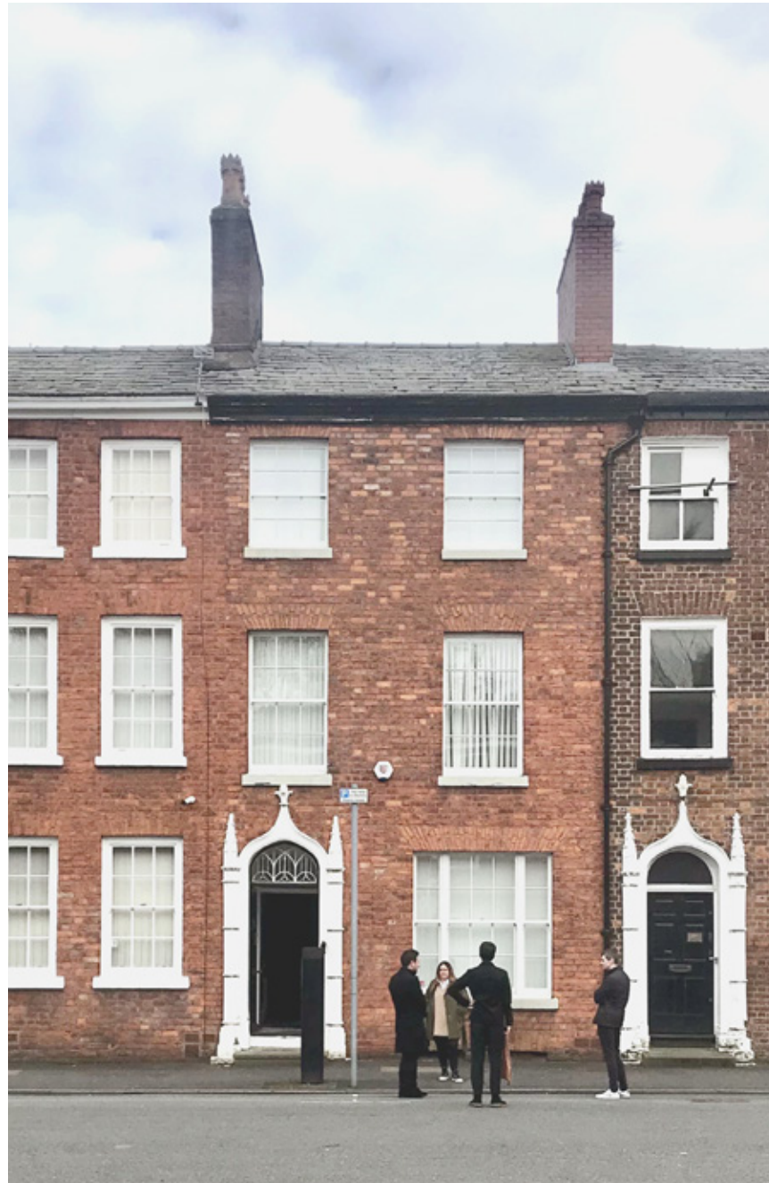
Front elevation of 27 Byrom Street
