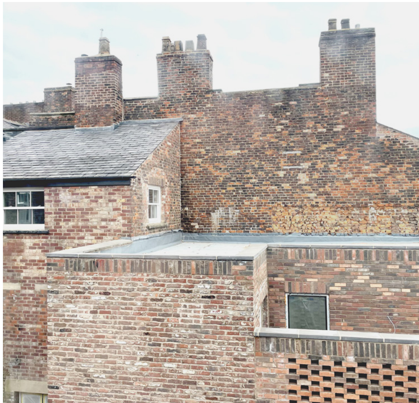
View from the second floor window of 27 Byrom Street Looking to the first and second floor extensions to the rear of 19 and 21 St. John Street
