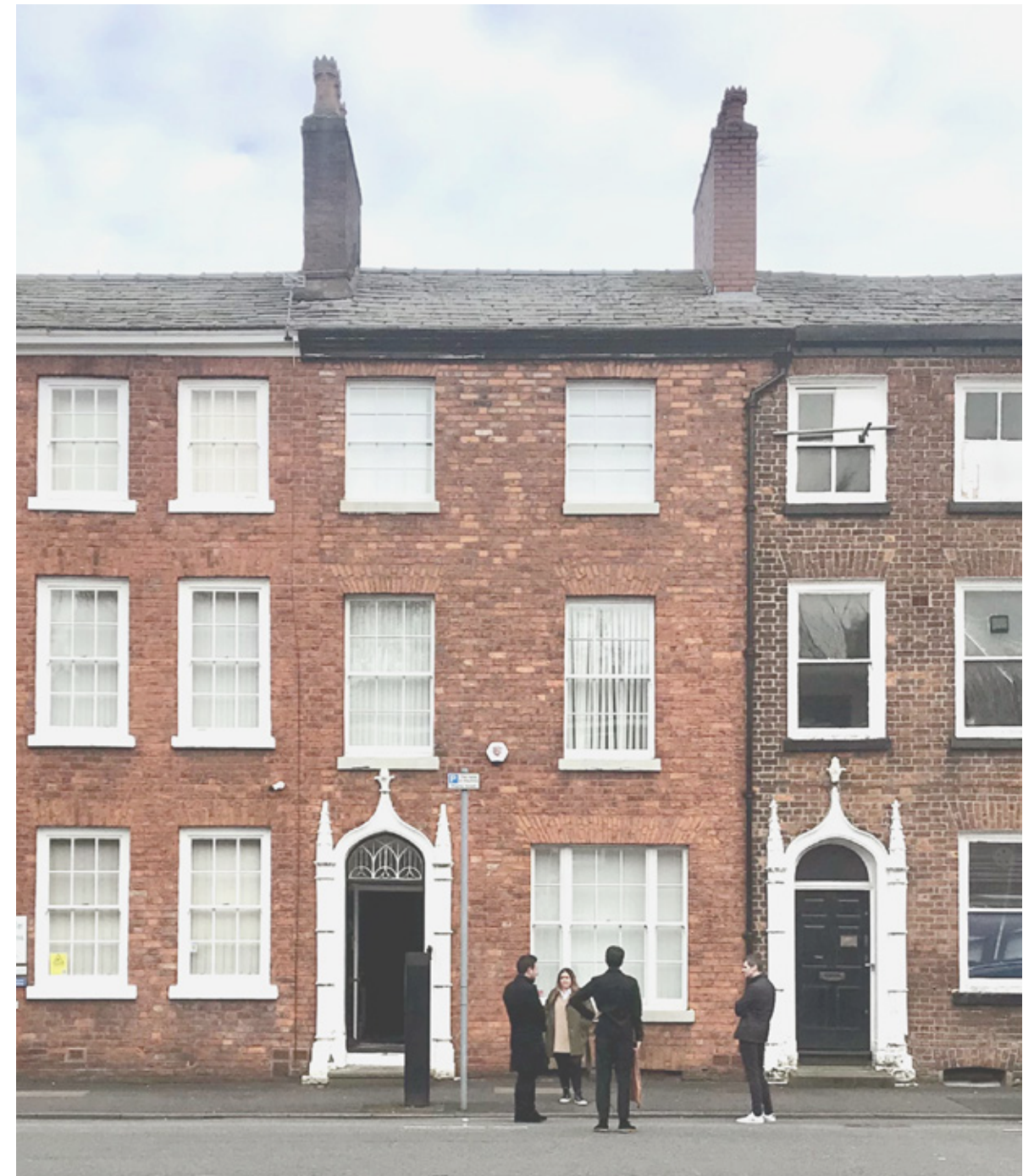
Front elevation of 27 Byrom Street
