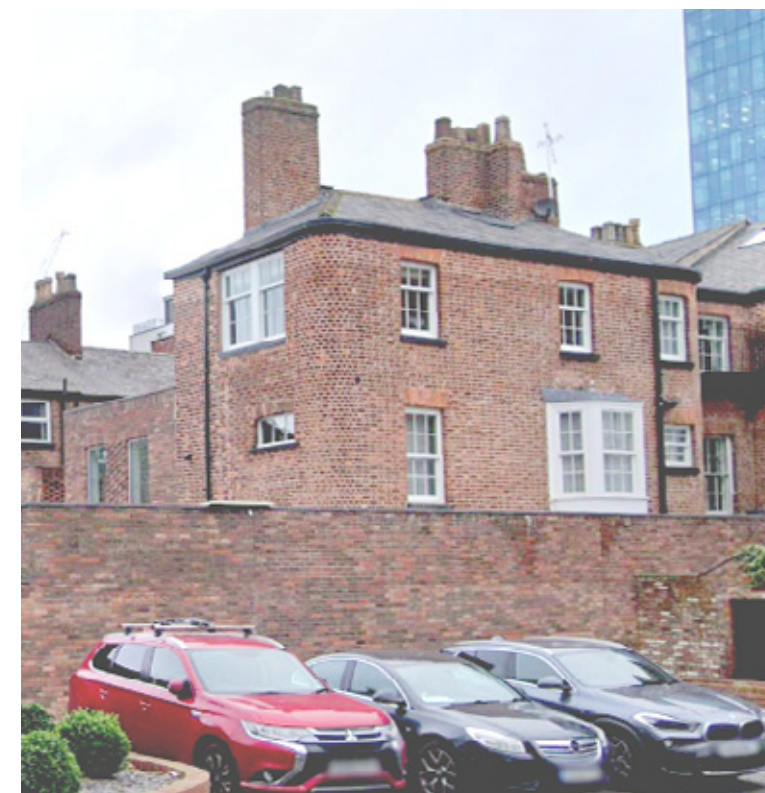
19 St. John street rear extension
