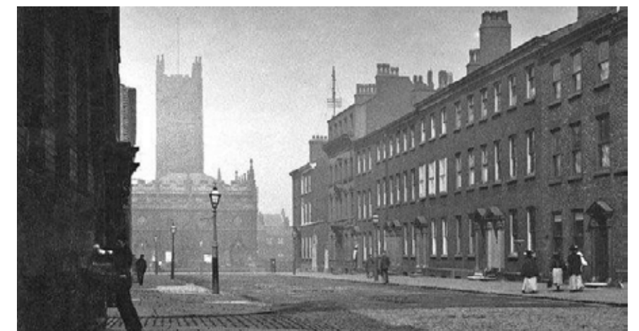
B. Archive image of St John Street from Deansgate (the elevations of St. John street are largely unchanged to this date)
