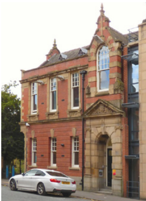
① Byrom Street Chambers Grade II listed late 19th Century building A building with decorative facades combining sandstone and red brick
