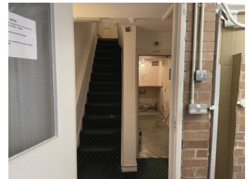
02. View of the staircase from the basement to ground floor
