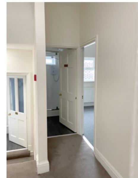
02. View of later additions of a stud wall and shower room
