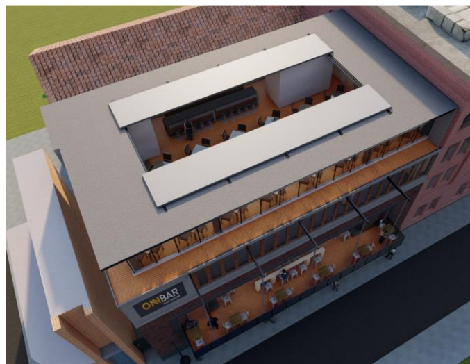
Figure 3 Rooftop terrace showing retractable roof
