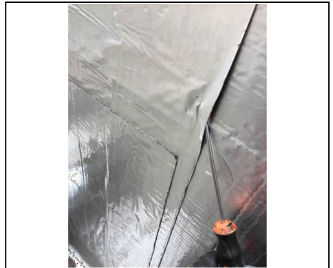
Pick and probe test to perimeter
