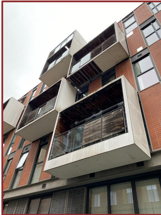
Photograph 02 - South Elevation showing Pod Balconies and HPL Cladding
