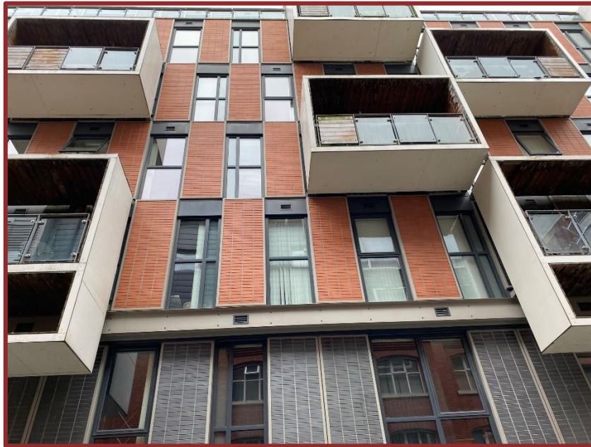
Photograph 04 - North Elevation from Simpson Street
