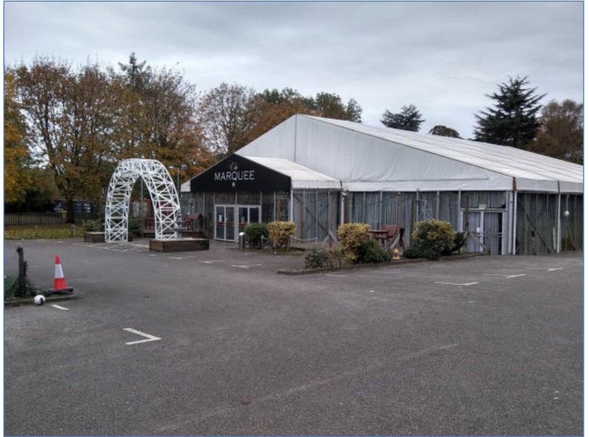
Plate 5: View of the Marquee and car park to the south of the British Muslim Heritage Centre, from the northeast
