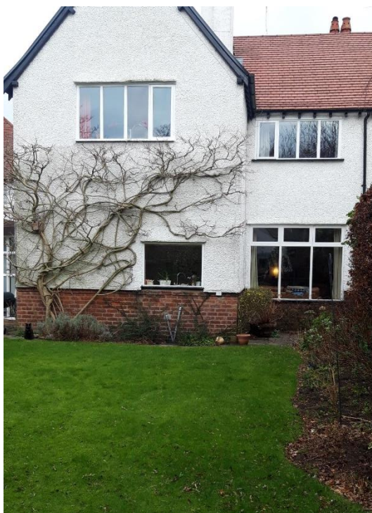
Rear of the house:
