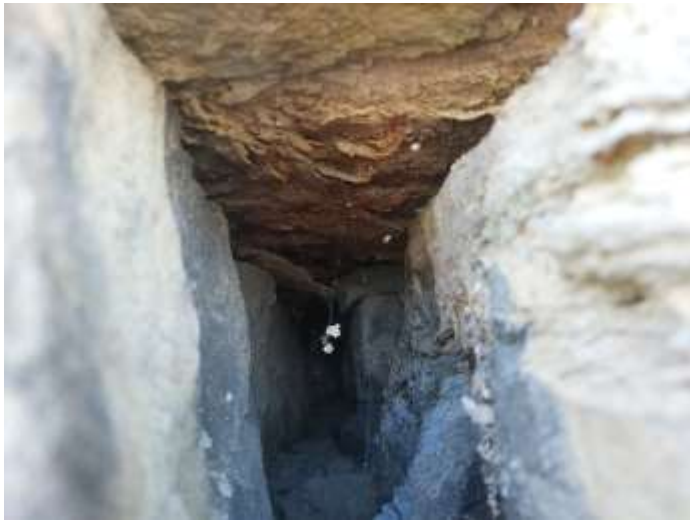
14: North West Elevation: Coping Stone pinned, rebed of top level block, Spalling to be repaired
