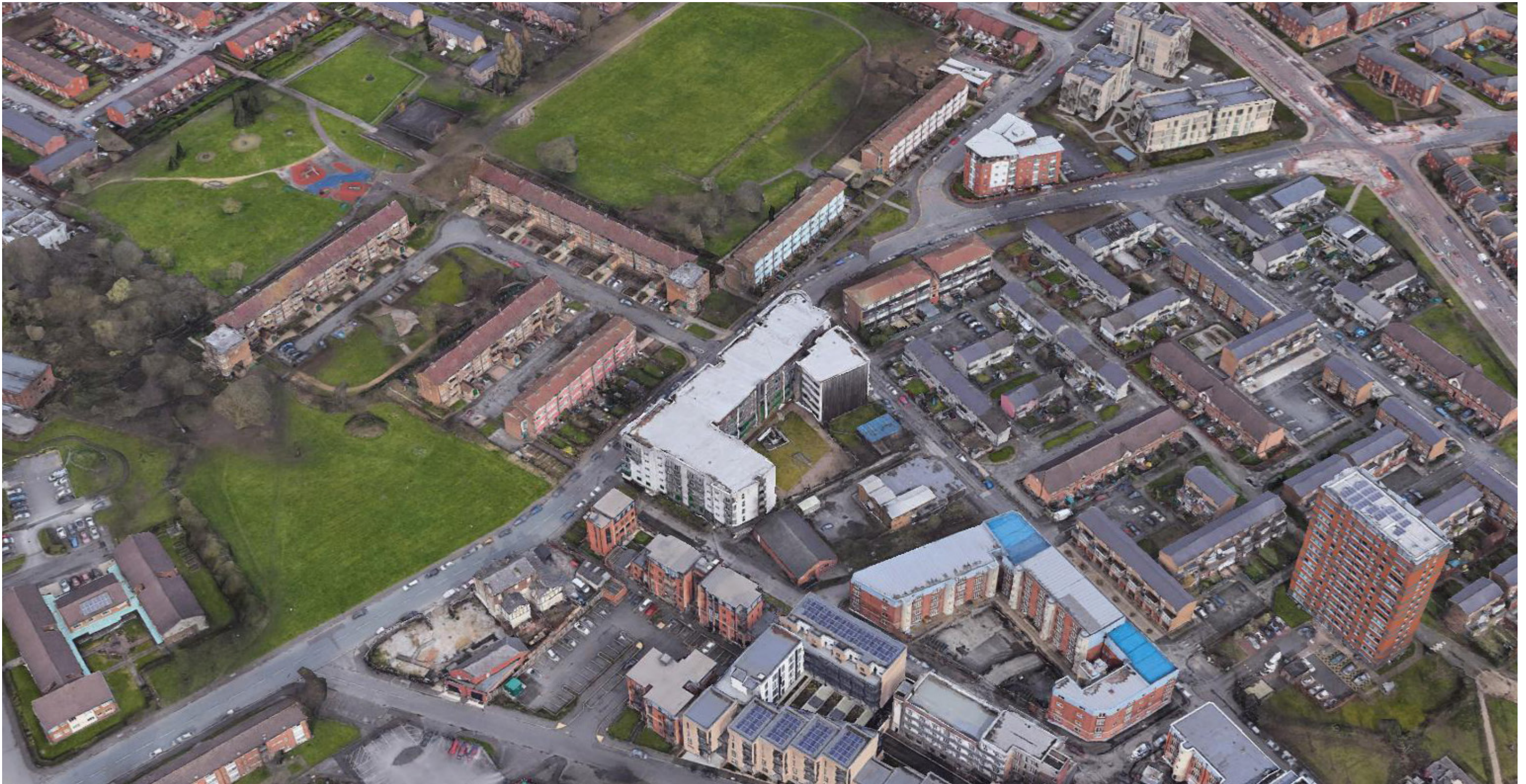
aerial photograph of site
