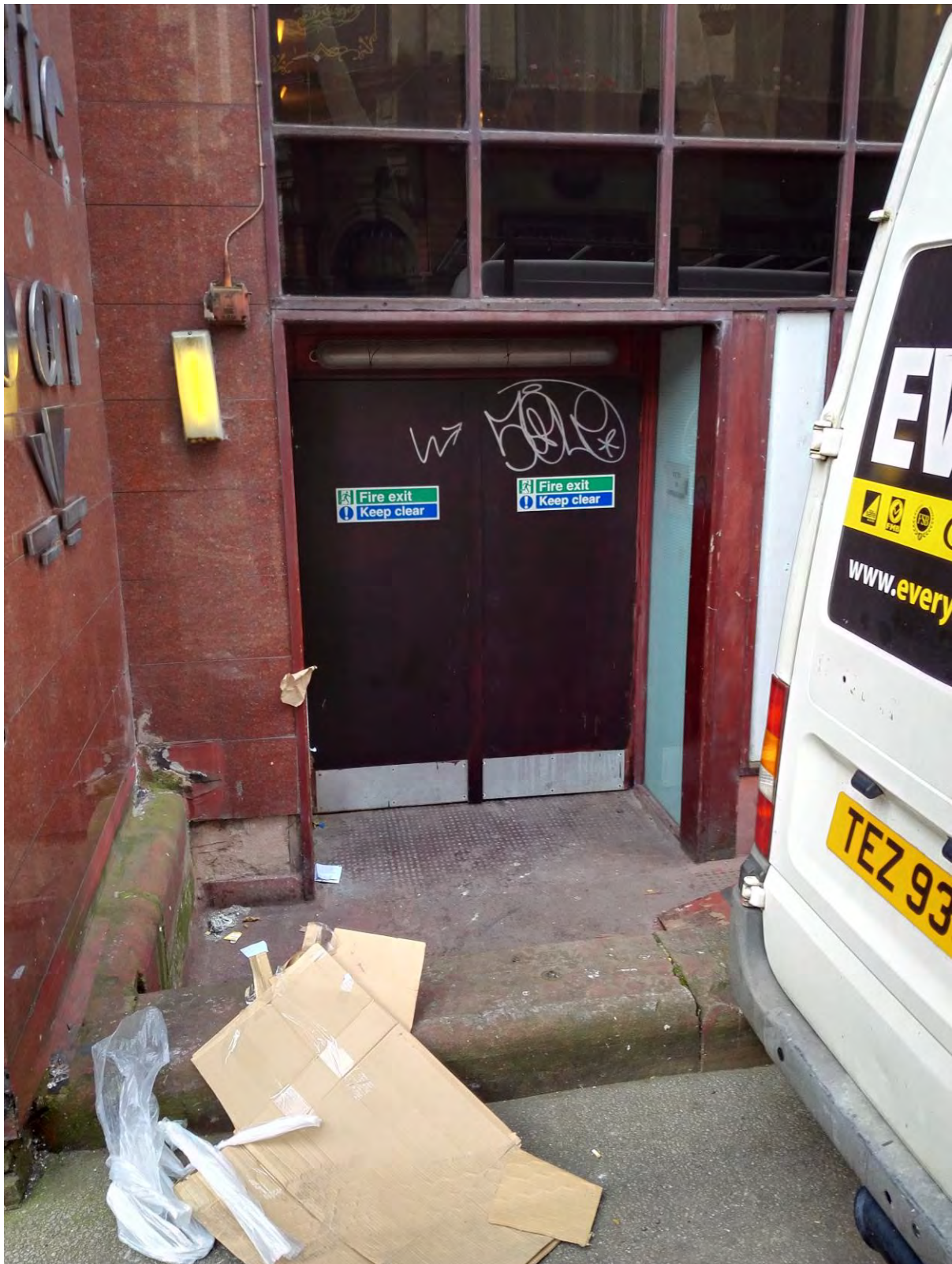
Photograph 3 – Access to the basement through a fire exit off of Back Piccadilly.
