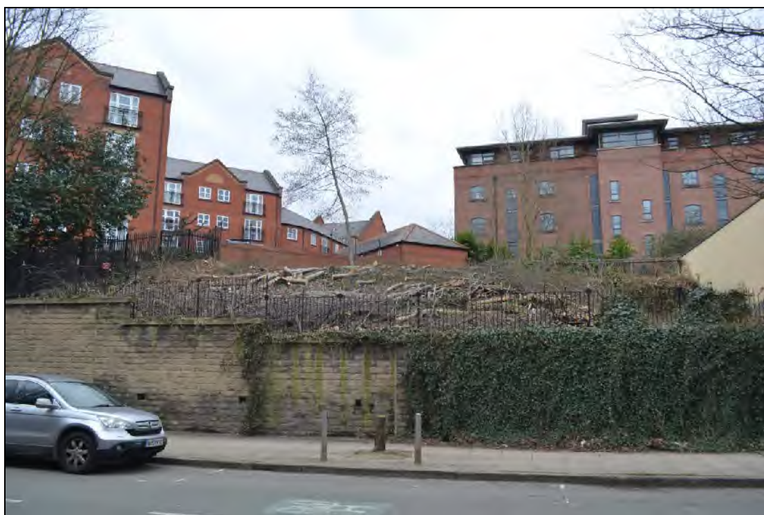
Photograph 3: View south east from Store Street across the PDA showing the rise in ground level within the site itself.
