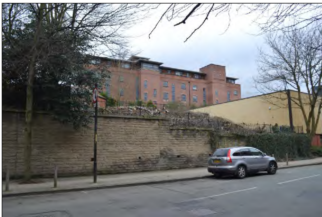
Photograph 4: View south-west along Store Street of the PDA and the adjacent industrial unit.
