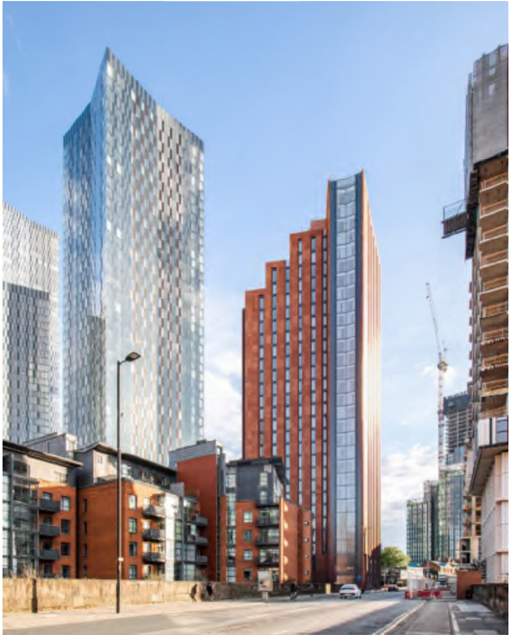
Figure 46: View from west along Chester Road. Scheme Overview Document Appendix 1 Page 21
