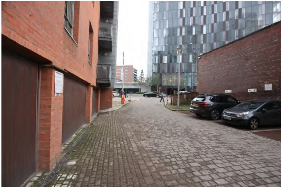
Figure 4: Photograph of boundary to Deansgate Quay. To the left of the frame is Deansgate Quay and to the right the red brick retaining wall at circa 4m
