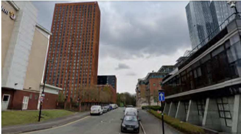
Figure 23: River Street Tower. Student accommodation block in weathered steel cladding. Source: Google Earth
