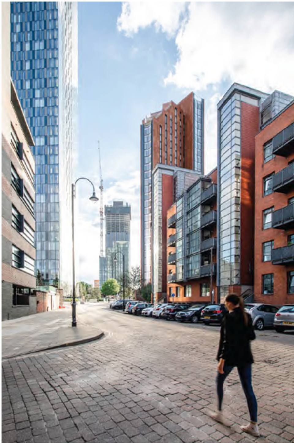
Figure 48: View from South-east along Deansgate. Scheme Overview Document Appendix 1 Page 22
