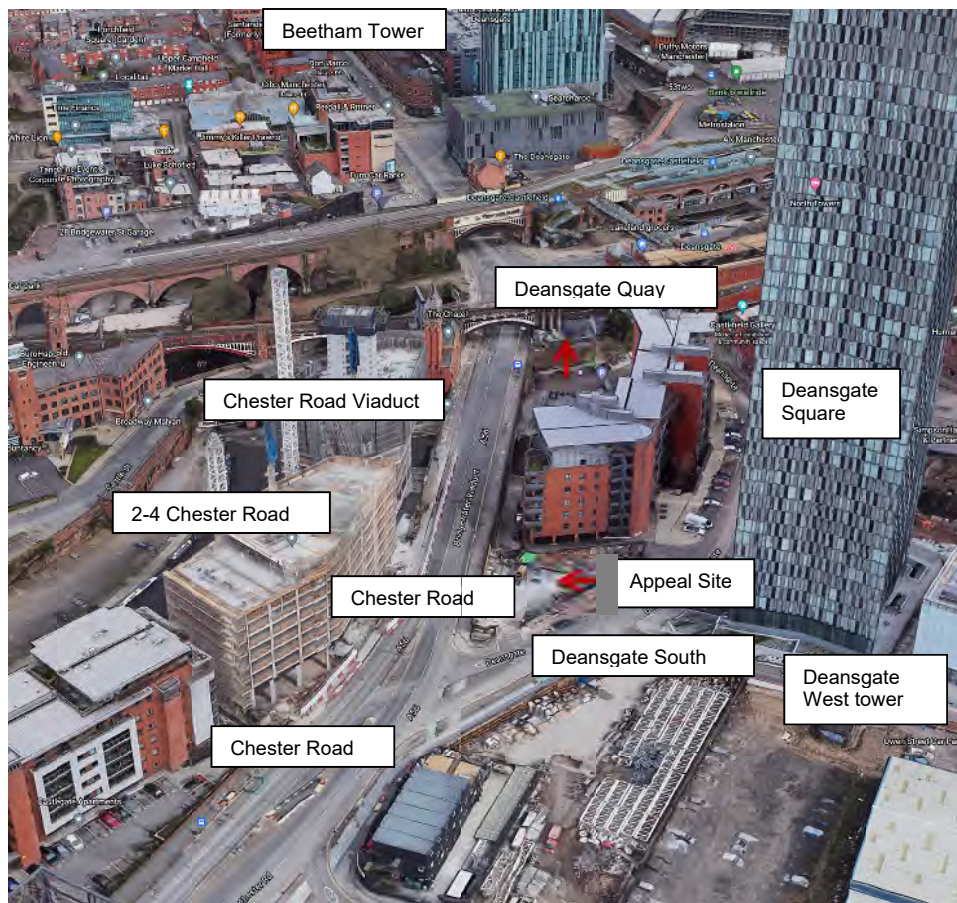
Figure 3: Aerial view of Deansgate Quay looking due east and above at the immediate context of the appeal site. Source: Google Earth. In the foreground left of frame and under construction is the 2-4 Chester Road development now complete. Evident in this view is the significant contrast in height, scale and massing between the Deansgate West tower to the right of the frame and the Deansgate Quay apartments to the centre of frame
