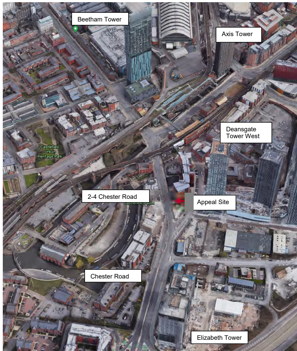
Figure 11: Sequence of tall buildings along Chester Road looking east. Source: Google Earth
