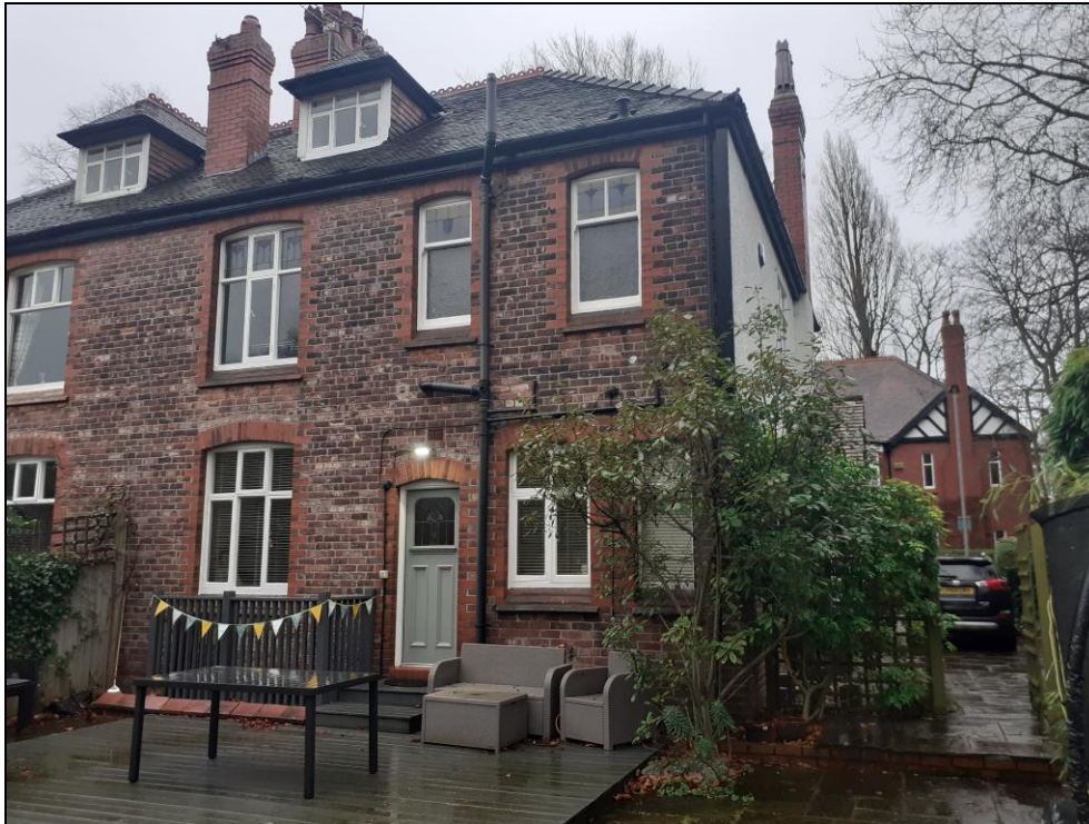
Figure 5.5: View of the rear elevation of 16 Lyndhurst Road.
