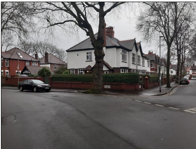
Figure 2.3: View of 16 Lyndhurst Road (south west elevation).
