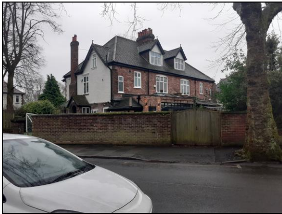
Figure 5.1: Single storey brick rear extension to 18 Lyndhurst Road with flat roof, lantern skylight and bifold doors.
