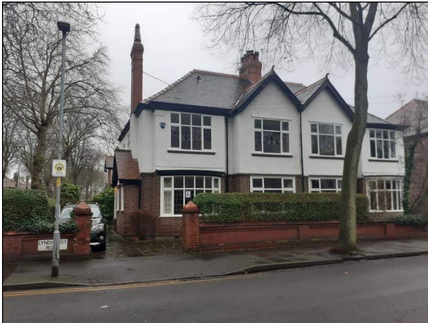
Figure 2.2: View of 16 Lyndhurst Road (south east elevation).
