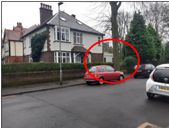
Figure 5.3: Single storey side extension to 19 Ballbrook Avenue with lantern skylight and bifold doors.
