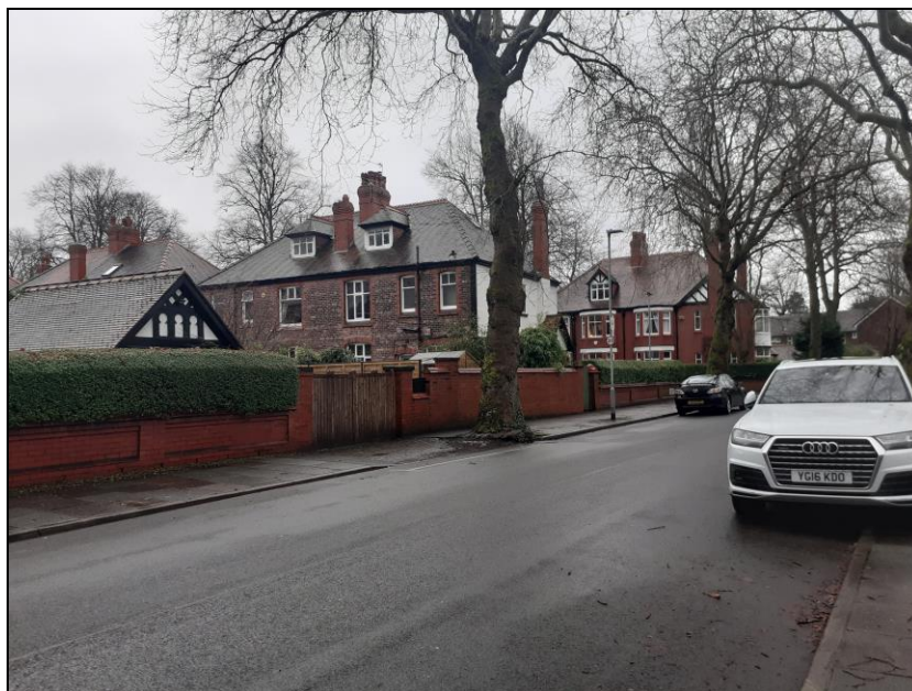
Figure 5.4: View looking east along Ballbrook Avenue towards the rear of 16 Lyndhurst Road.
