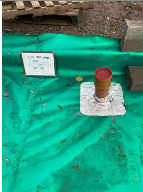
Photograph 7: Validation of Gas Membrane Installation
