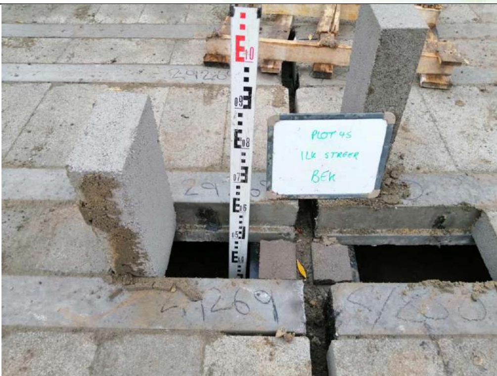
Photograph 4: Validation of Sub-Floor Void Space (min 150 mm)
