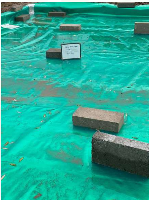
Photograph 6: Validation of Gas Membrane Installation
