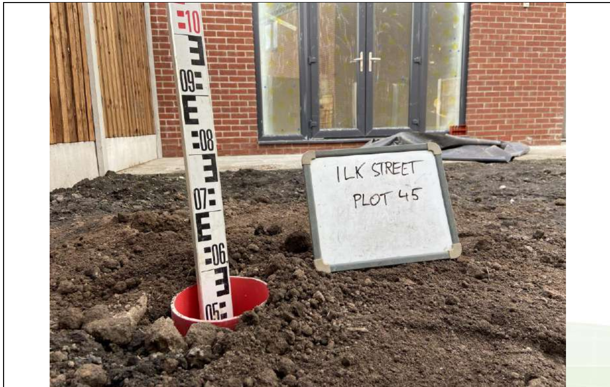
Photograph 1: Validation of Garden Capping Thickness
