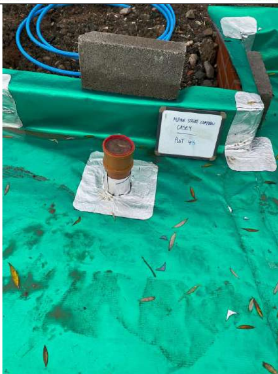
Photograph 5: Validation of Gas Membrane Installation
