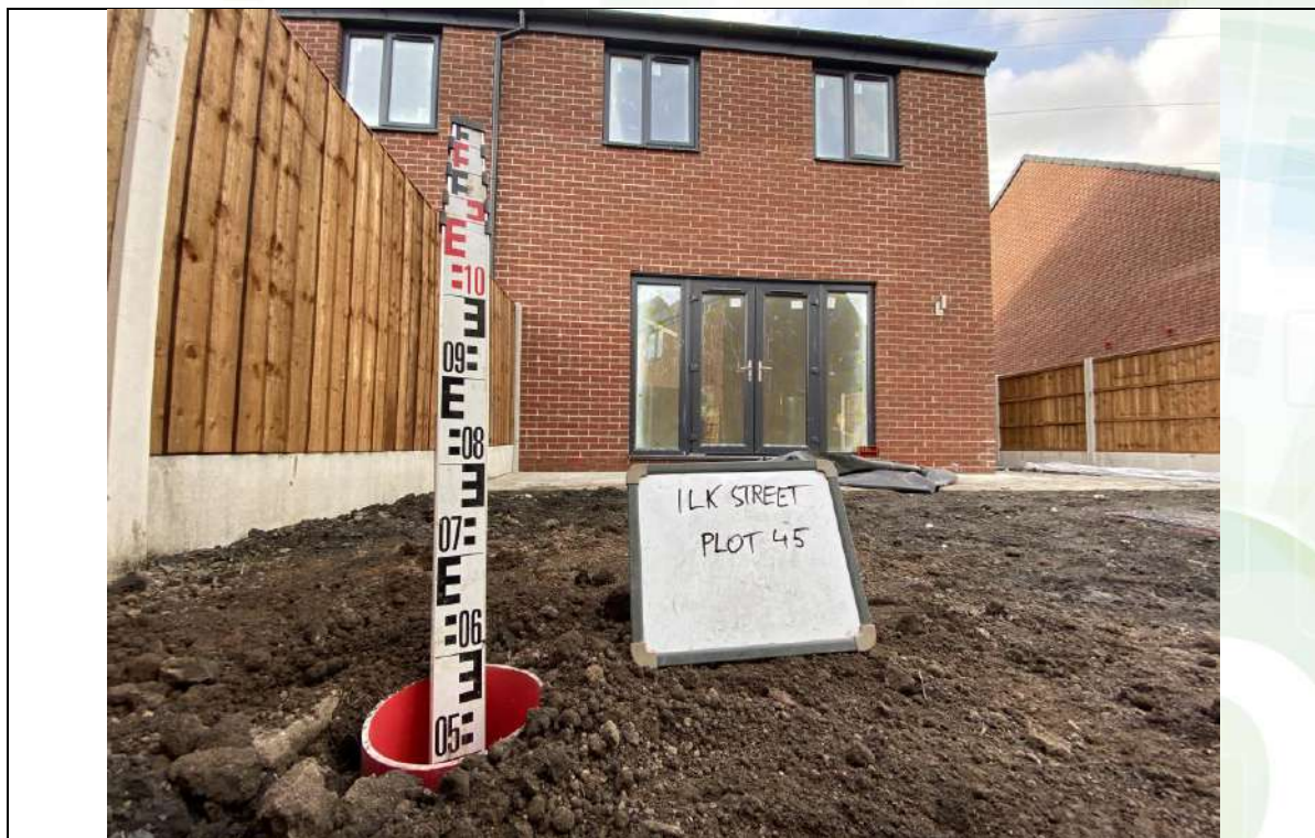
Photograph 2: Validation of Garden Capping Thickness
