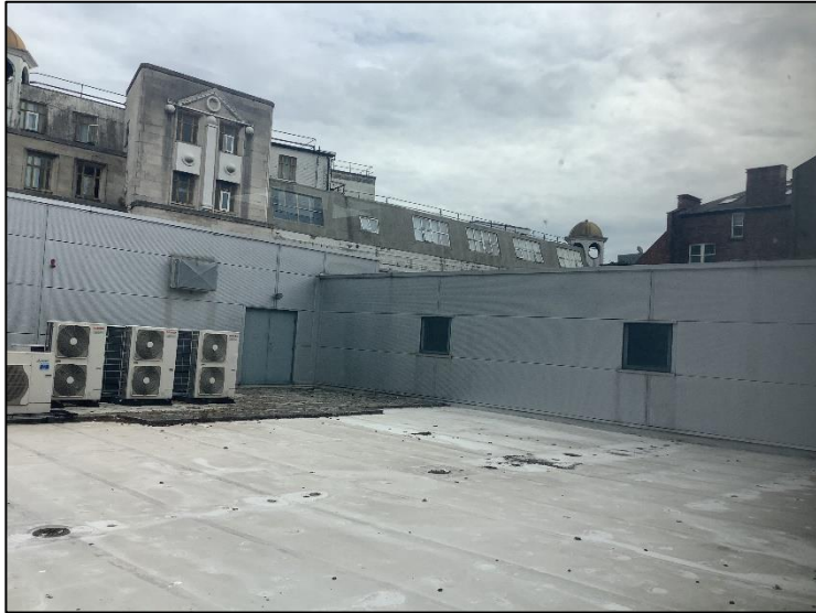
B1 – roof area.
