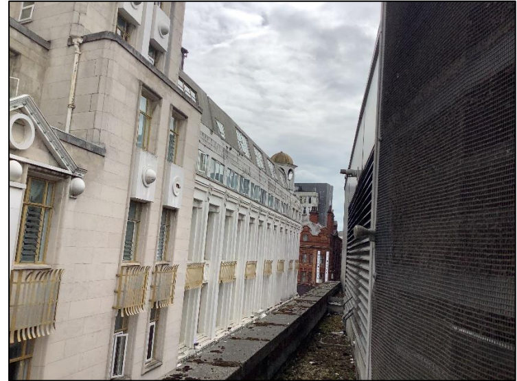
B1 – southern roof area.
