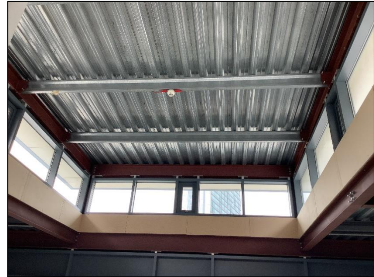
B1 – upper floor roof structure.
