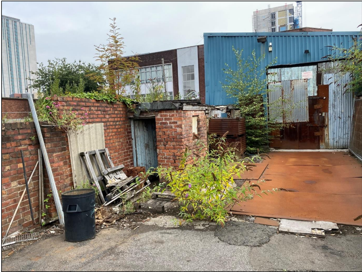
Figure 4 - Main Scrap Yard looking north-east
