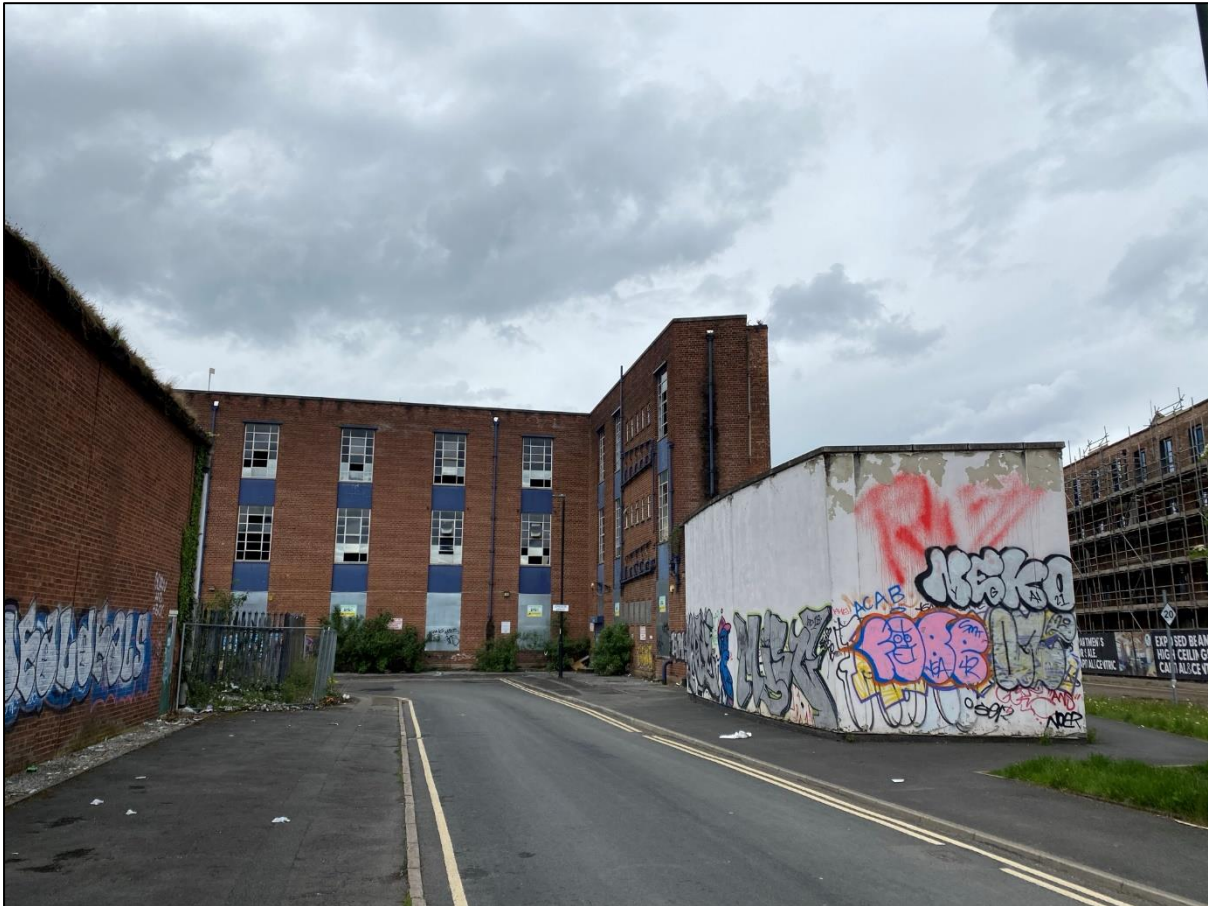
Figure 2 - Rammon House looking south-west along Longacre Street
