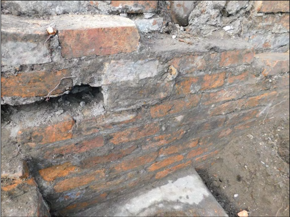
Plate 7: Detail shot of hook above boiler 121, looking south
