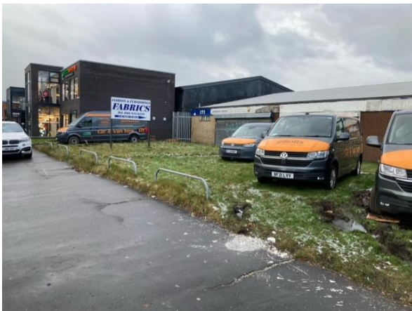
Existing front boundary
