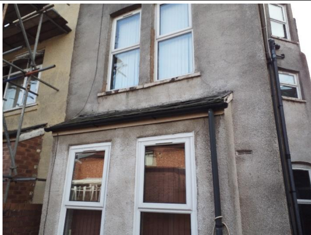
Figure 05: General view of lower rear elevation
