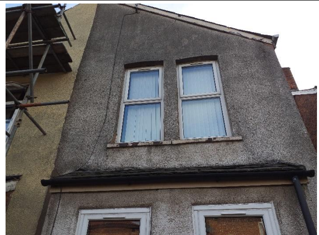
Figure 06: General view of upper Rear Elevation
