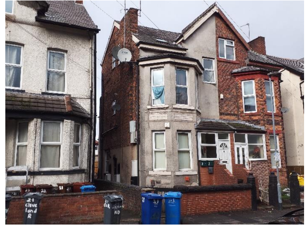
Figure 02: General view of Front and Part side Elevation
