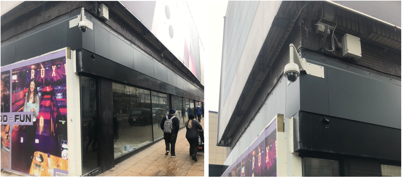
Photographs 3 and 4: Market Street / High Street Corner
