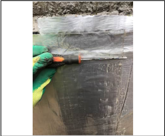
Good overlaps used in D7 core
