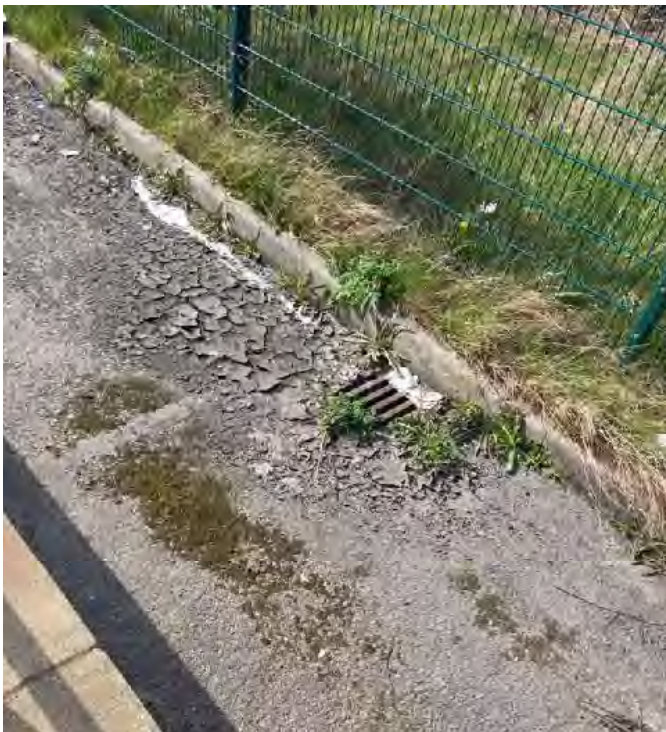
Photo 23: Drainage grid present within Site C.
