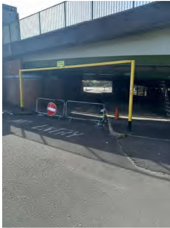
Photo 17: Pre-existing tunnel under the Trinity Way bridge connecting the two sites.
