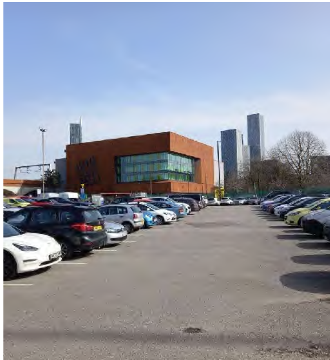
Photo 2: Looking southeast from the centre of Site C, looking at nearby storage building.
