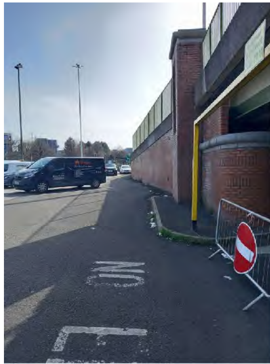
Photo 18: Looking south along the retaining wall adjacent to Trinity Way bridge, in good condition.
