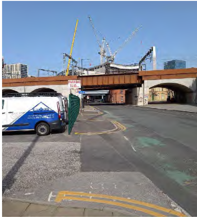
Photo 5: Looking east along Water Street.
