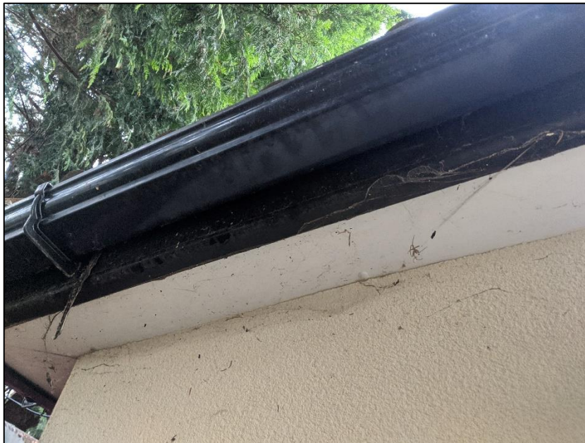
Photograph 5 showing the soffits
