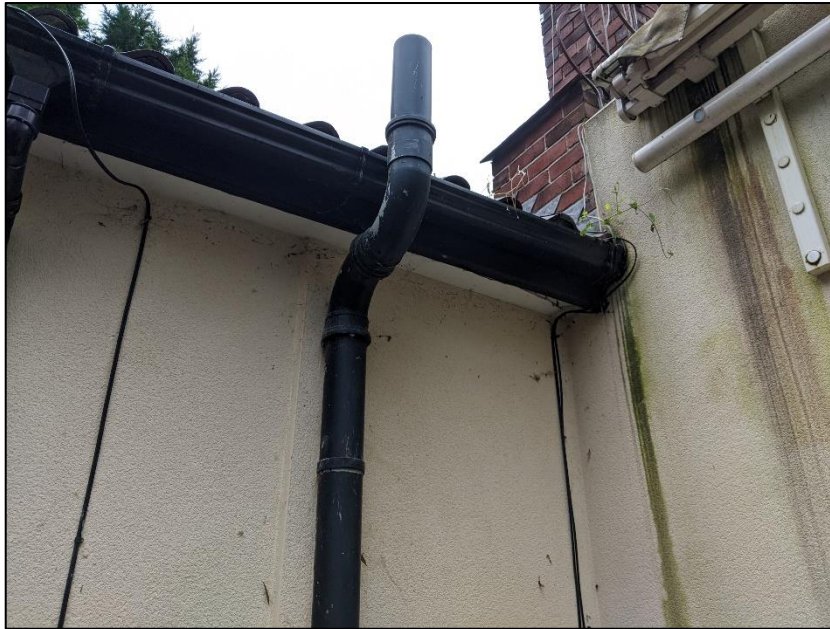
Photograph 2 showing the rear elevation
