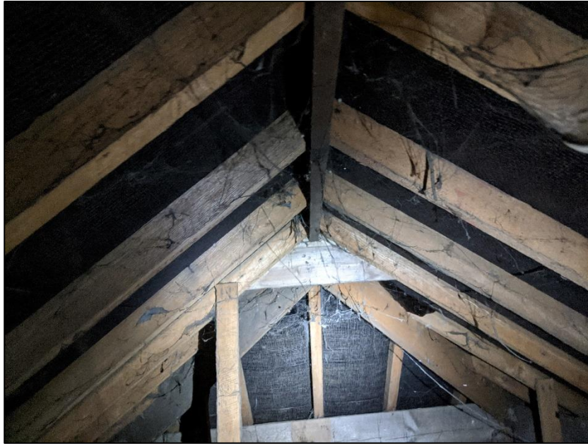
Photograph 6 showing the roof timbers
