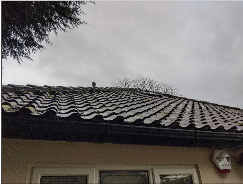
Photograph 4 showing the roof of the property
