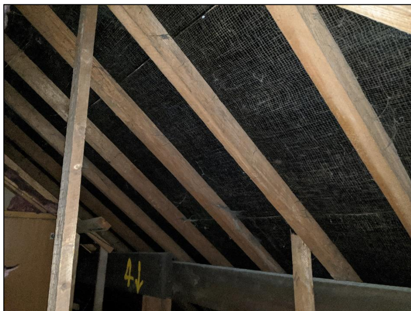
Photograph 7 showing the roof lining
