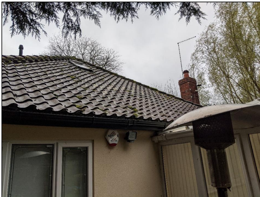
Photograph 3 showing the roof of the property from the rear
