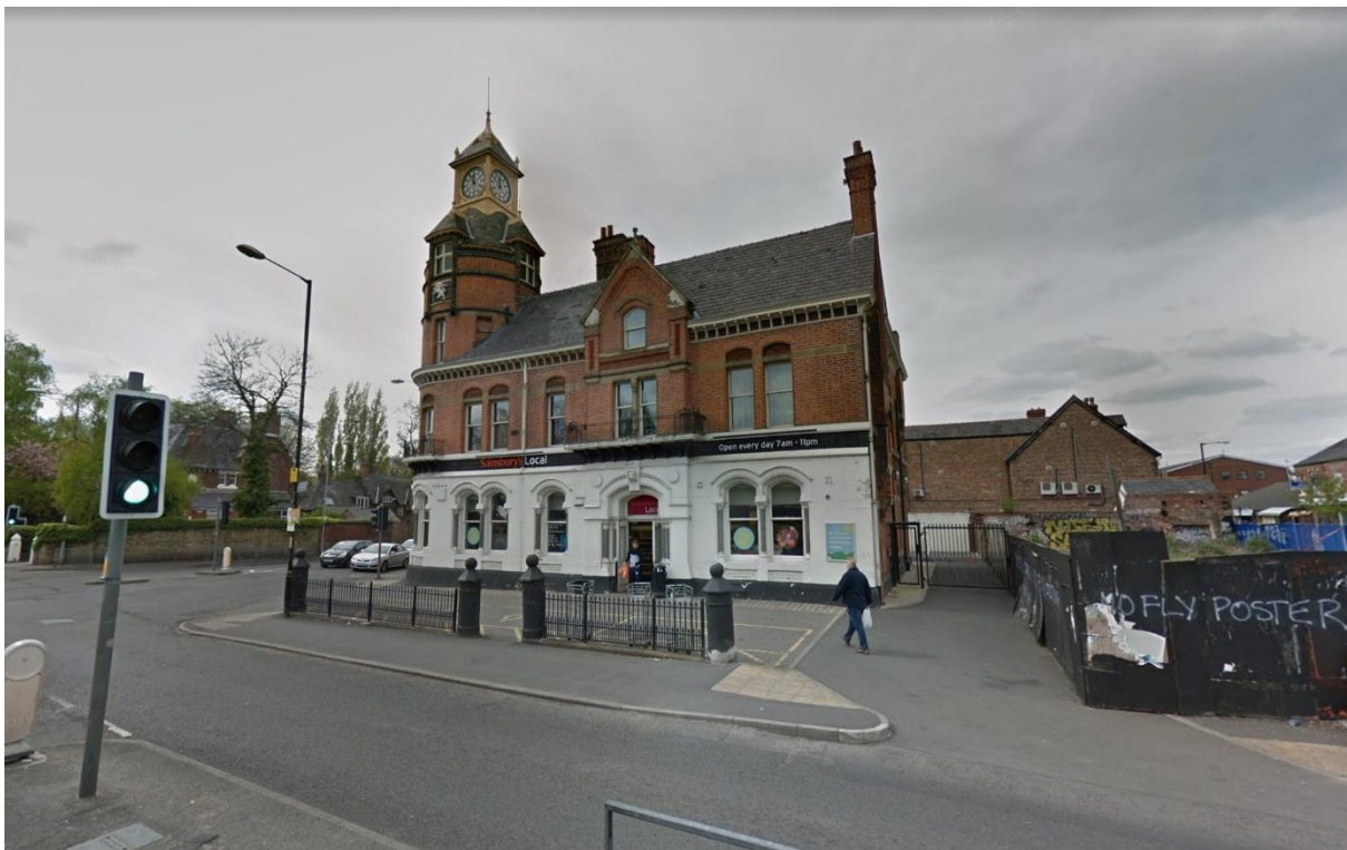
Fig 4: Former White Lion Public House, grade II listed, on the corner of Wilmslow and Burton road.
