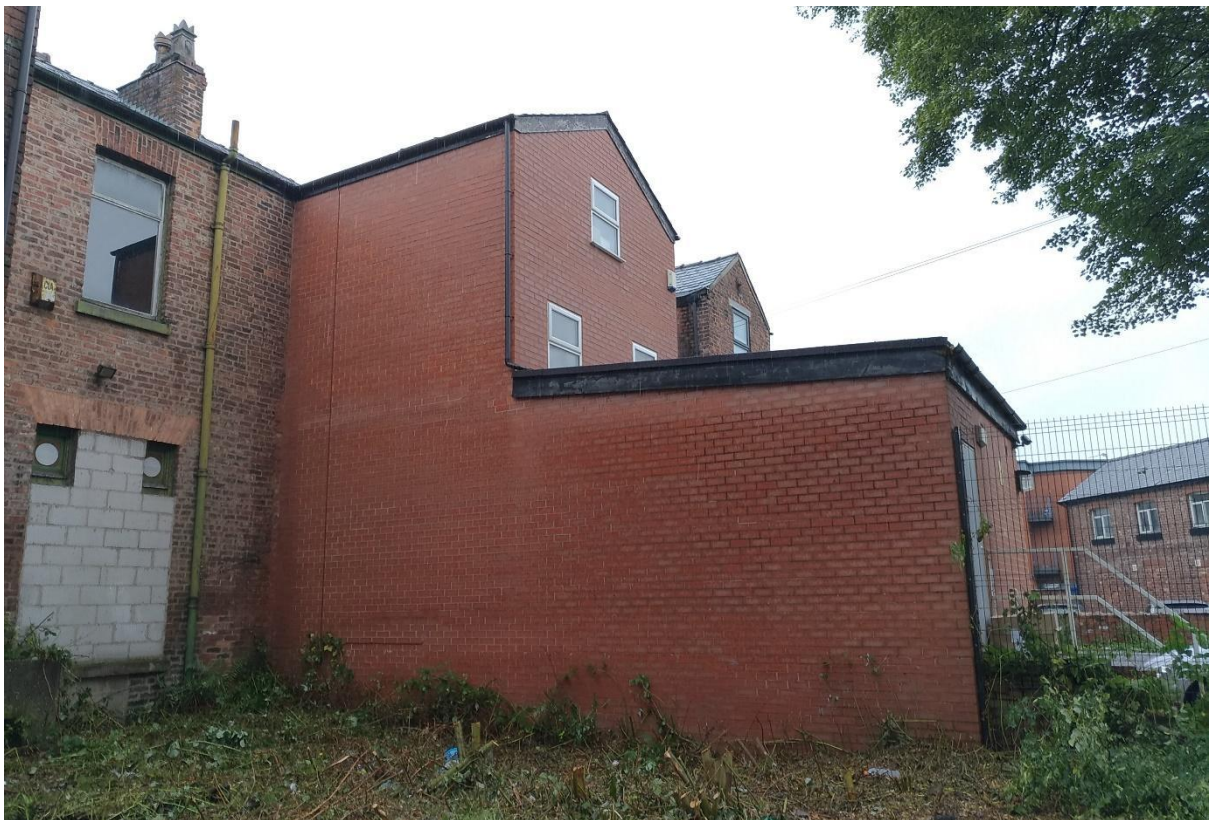
Fig 10: View of adjacent property and extension.
