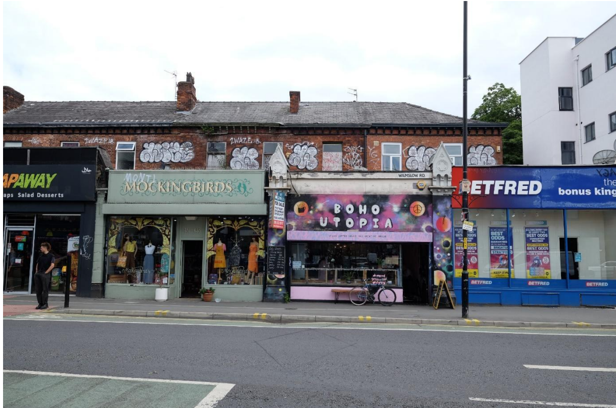
Fig 5: View across Wilmslow Road of application site.
