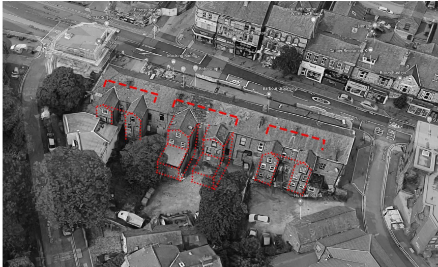
Fig 11: Aerial view of rear of application site in context highlighting pairing of outriggers.
