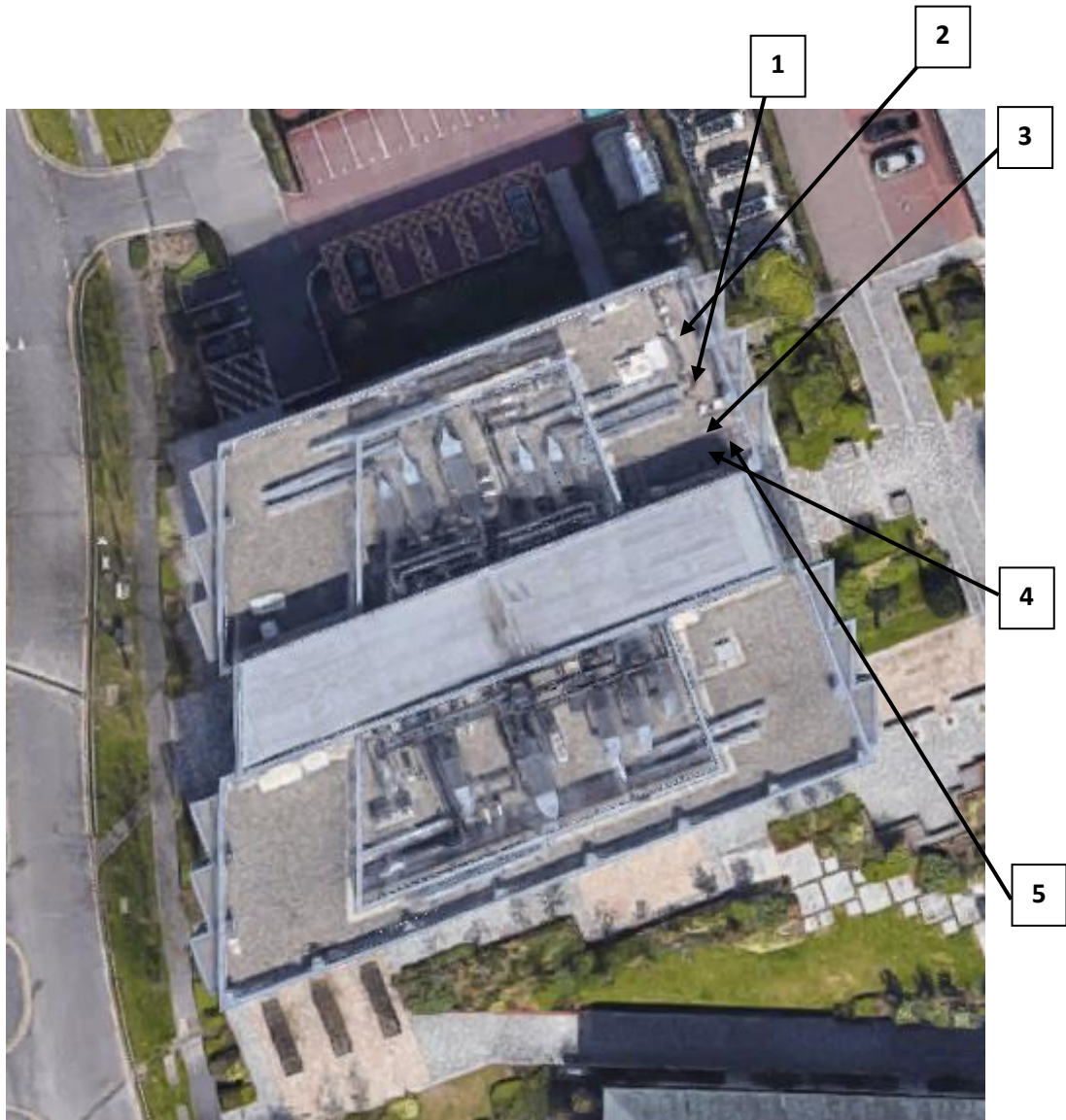
Photographs of Rooftop as Existing (arrows indicate direction of photograph)
