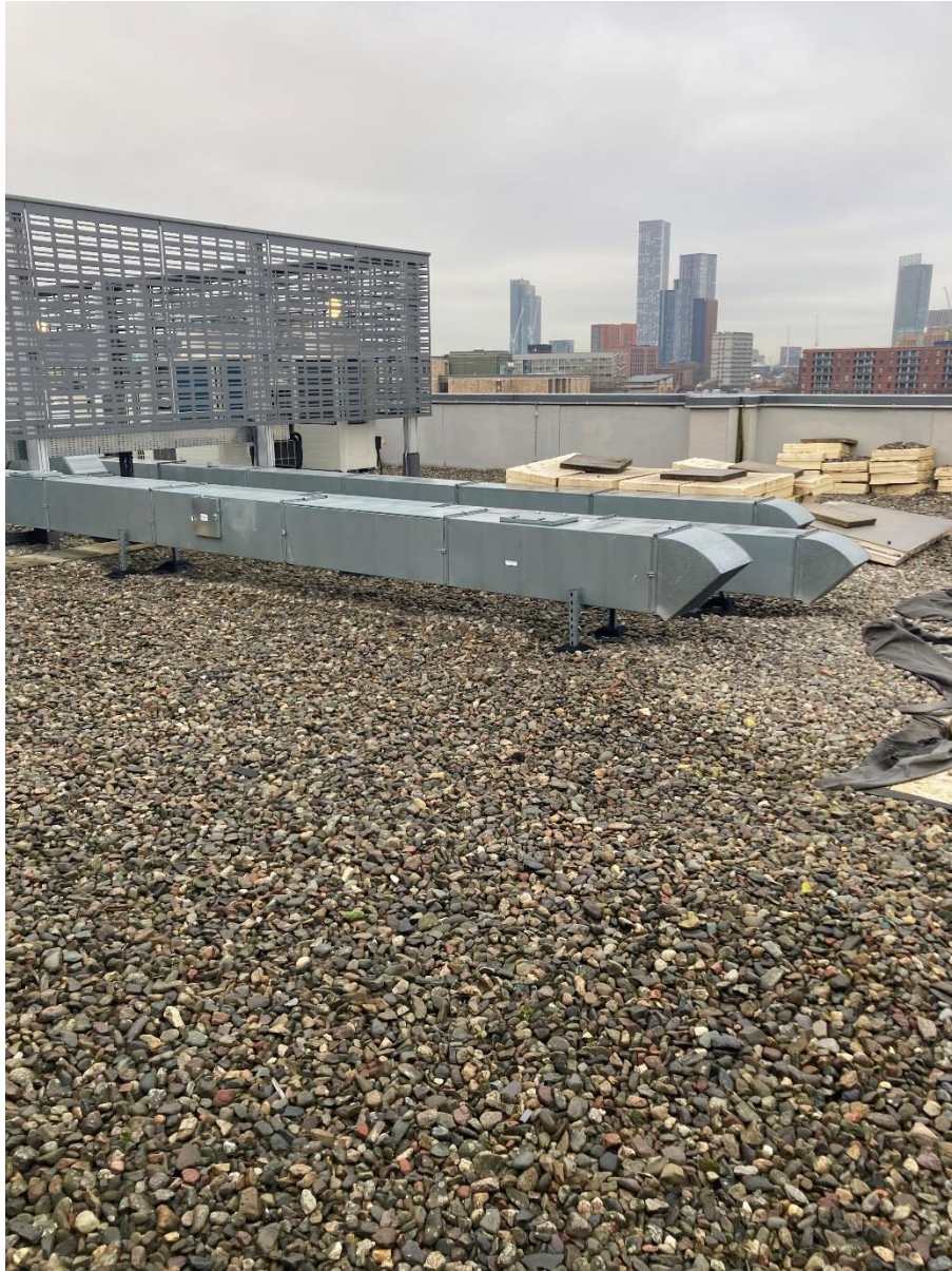
Photographs of Rooftop as Existing (arrows indicate direction of photograph)
