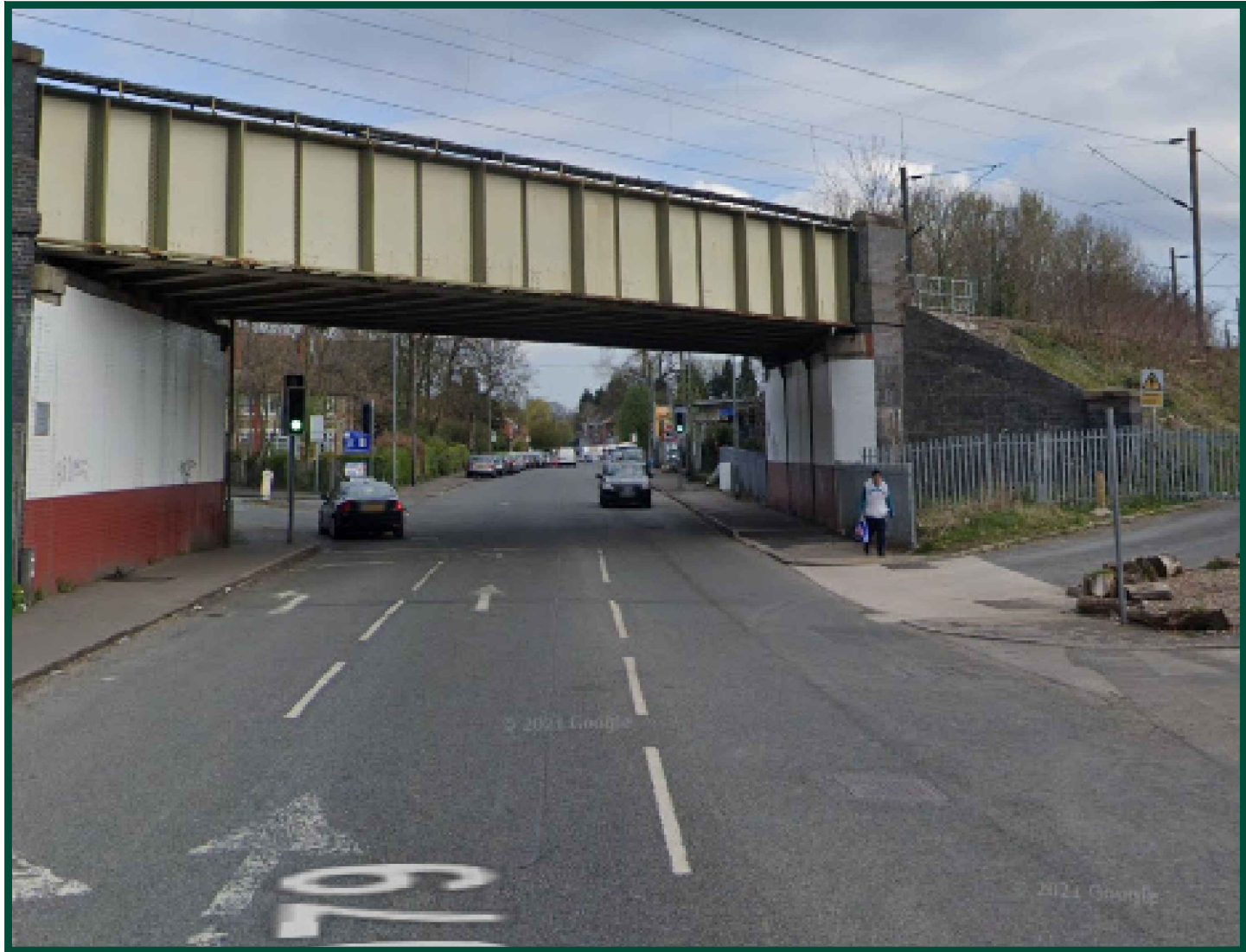
EXISTING SITE VIEW
