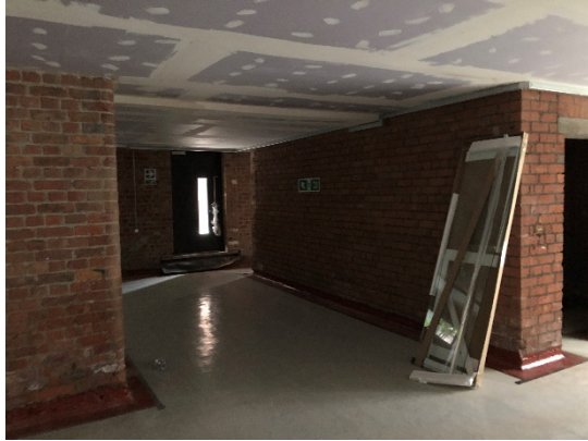
Figure 9: Looking north through the unit towards its entrance from Little David Street. Note the modern concrete floors and plasterboard ceilings.
