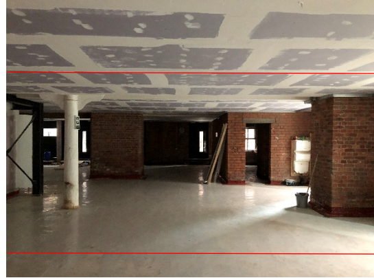
Figure 10: Looking north-west into Unit G4.1.1 from the adjacent unit, showing the approximate location of the proposed party wall (denoted by red lines).
