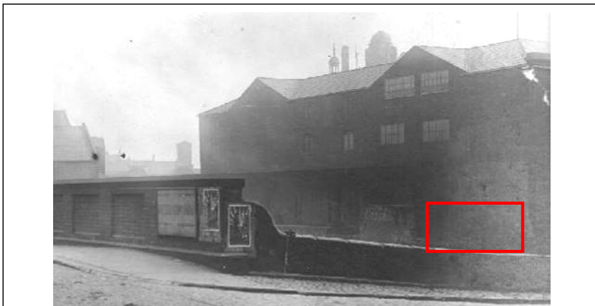
Figure 4: A view looking from the junction of Minshull Street (left) and Canal Street (right) in 1917, showing the rear elevation of Minshull House. The approximate location of the north-east elevation of Unit G4.1.1 is shown outlined.
