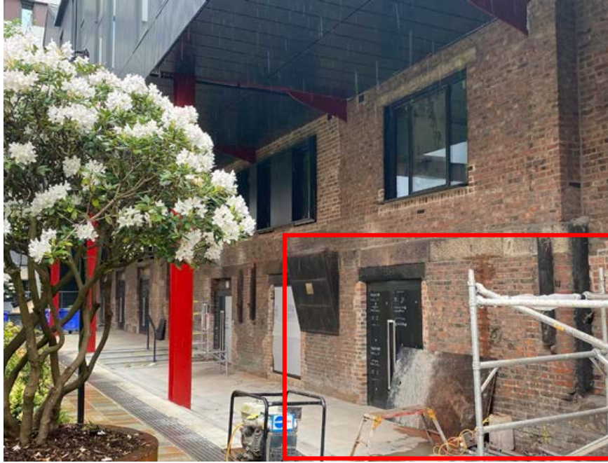
Figure 7: A current view looking in the opposite direction (south-east) along the completed external elevation of Unit G4.1.1 in 2022, which is shown approximately outlined.
